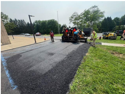
Photo: A paving crew operating an asphalt paving machine to lay fresh blacktop, with a finished paved section in the foreground.
