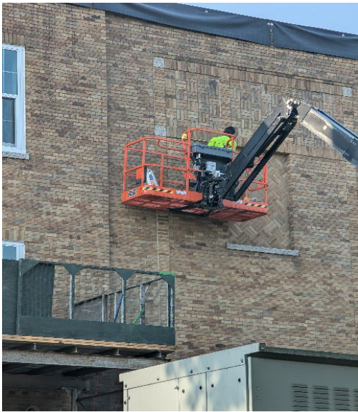
Photo: A worker in an aerial lift performing masonry or window repair work on the brick exterior of the high school.
