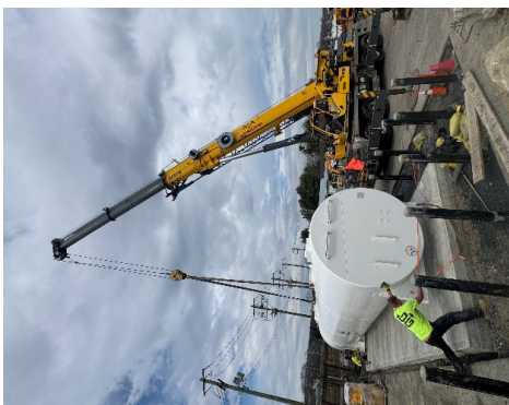
Photo: A crane lifting a large white cylindrical water tank into position outdoors, with a worker guiding it below.
