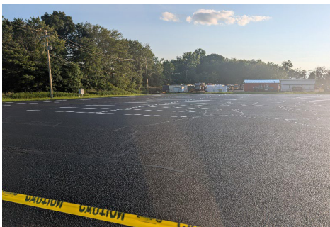
Photo: A newly paved parking lot with fresh striping, cordoned off with yellow caution tape, trees and a building visible in the background.
