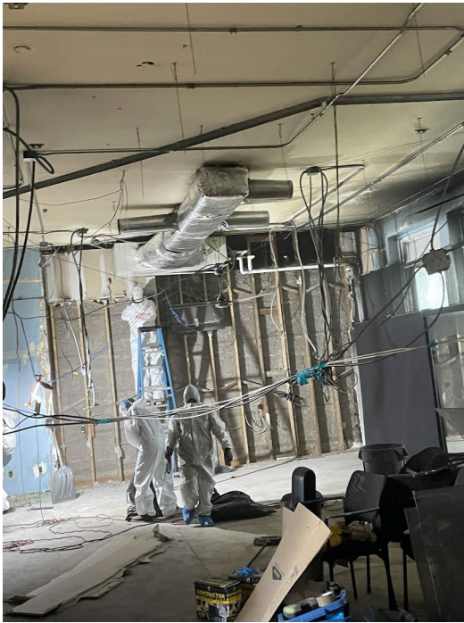
Photo: Two workers in white hazmat-style protective suits performing remediation work in a room with exposed ceiling and wall framing.
