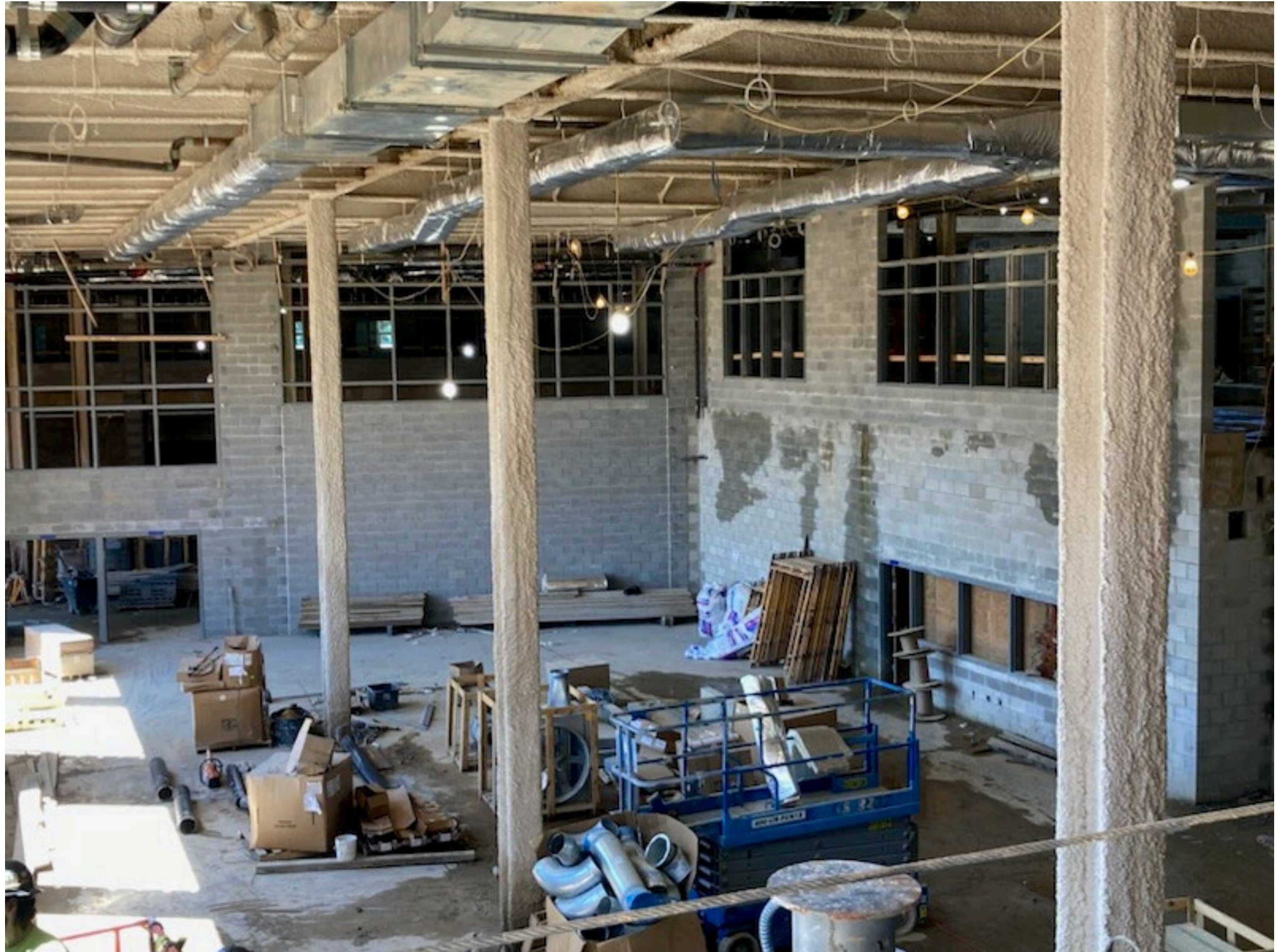
NORTH EAST MIDDLE / HIGH SCHOOL – REPLACEMENT – FIREPROOFING, DUCTWORK INSTALLATION CONTINUE THROUGHOUT
