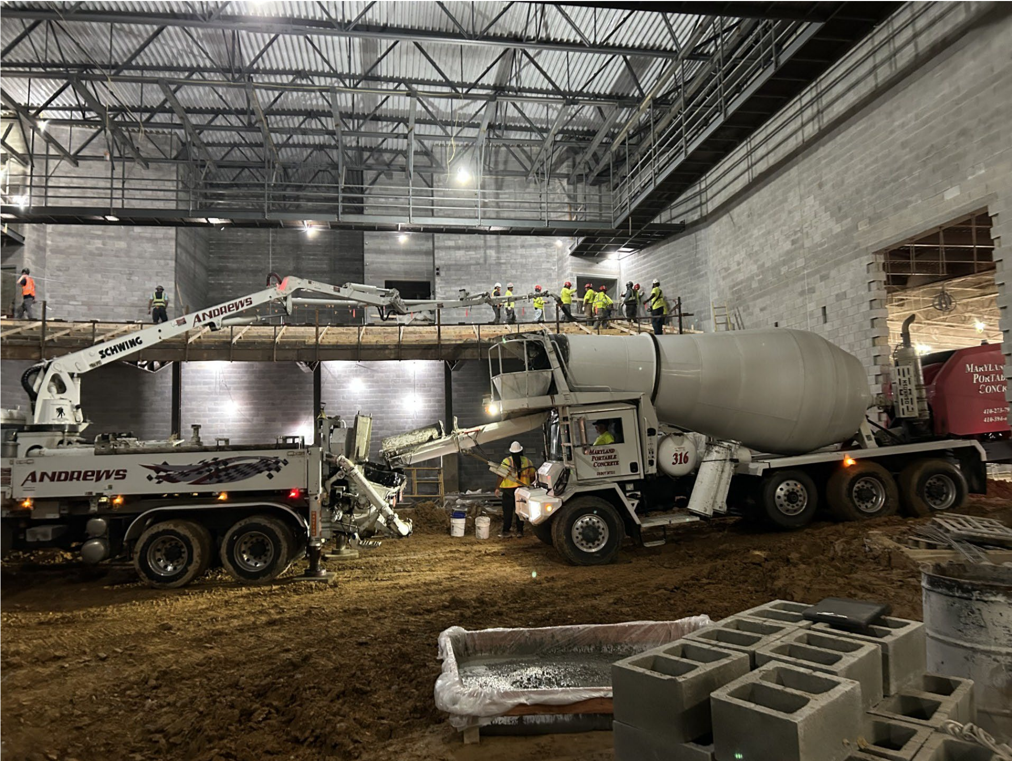
NORTH EAST MIDDLE / HIGH SCHOOL – REPLACEMENT – AUDITORIUM BALCONY
