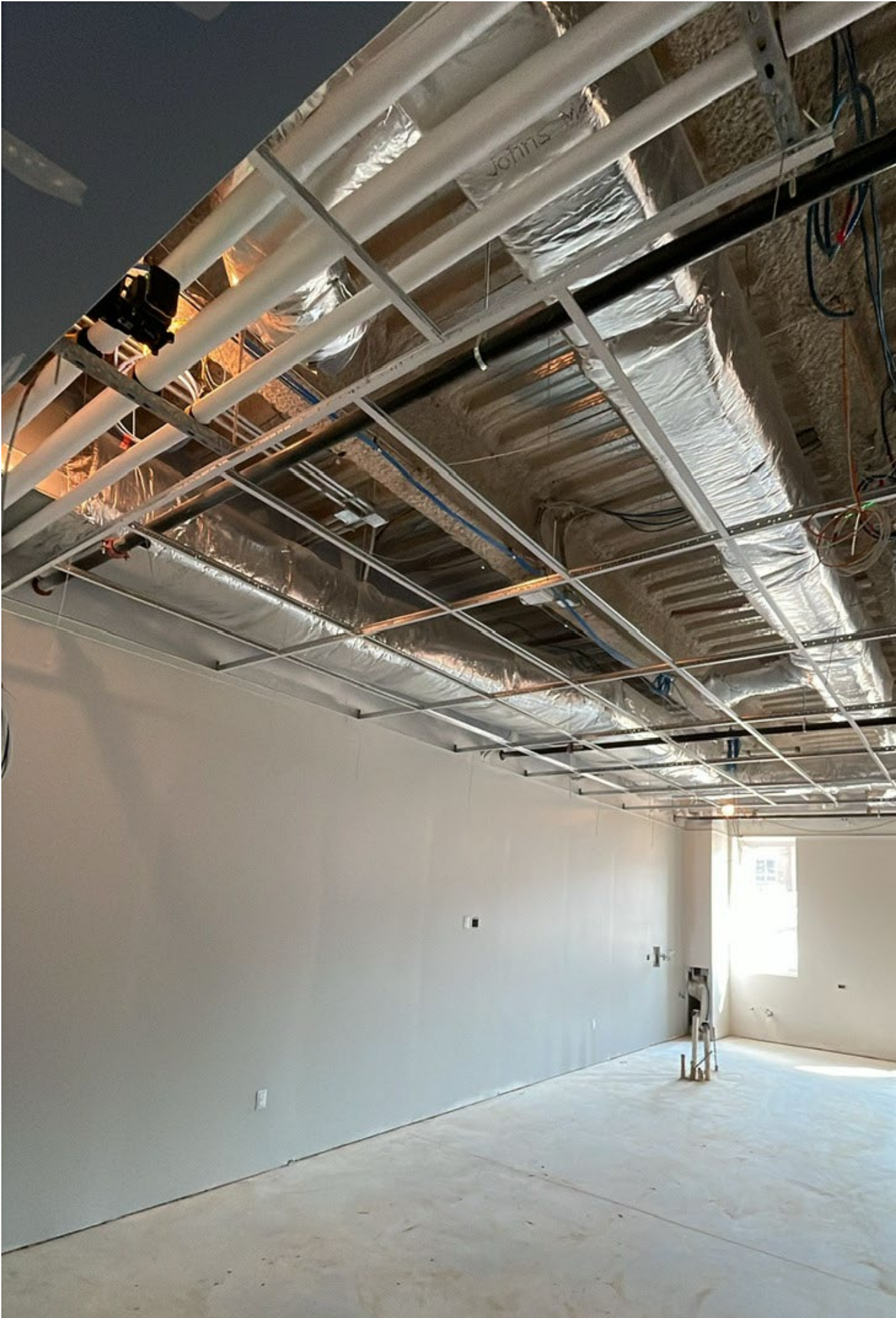
NORTH EAST MIDDLE / HIGH SCHOOL – REPLACEMENT - FRAMING, INSULATION, DRYWALL, PAINTING AND CEILING GRID CONTINUE THROUGHOUT
