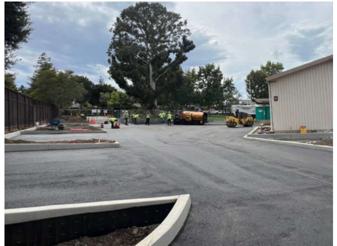
Pictured above : Site paving progress
