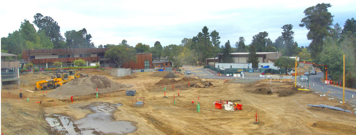
Pictured above : Grading and site infrastructure work
