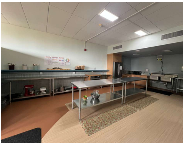
Pictured above : Casework, flooring, and ceiling tile installation
