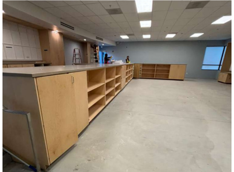
Pictured above : Casework and countertop installation
