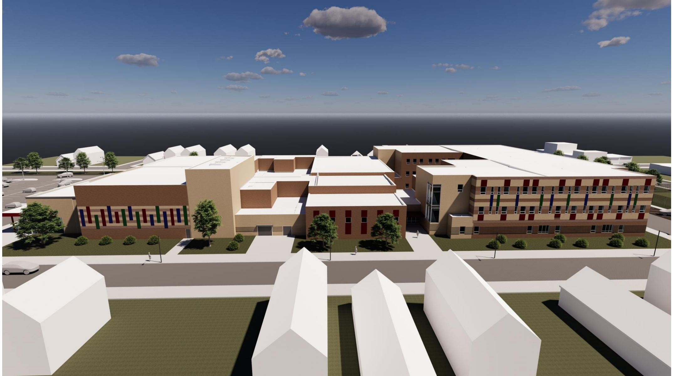
ELEVATED VIEW OF WEST ELEVATION
