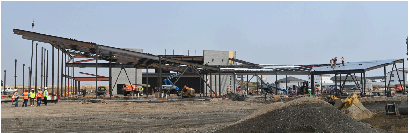
Construction progress at Skyway Elementary on Aug. 12, 2026.
