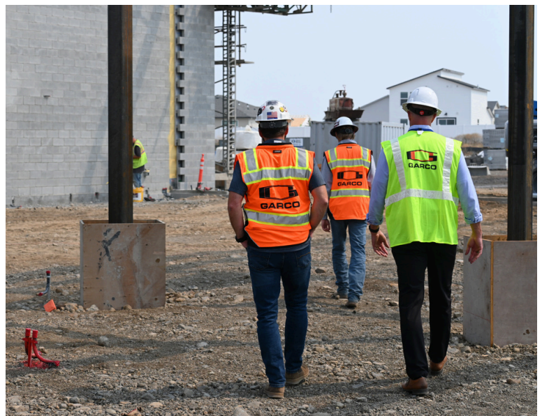
Superintendent Ben Ferney (right) walks the Skyway Elementary construction site with Garco Vice President Rob Decker (left) on Aug. 12.
