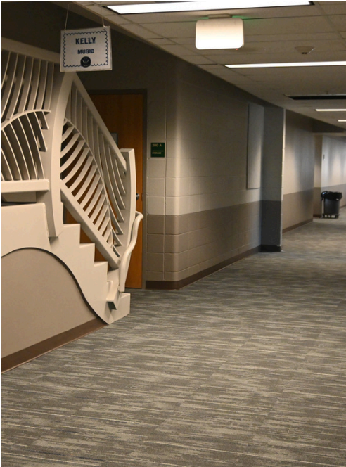
New flooring and fresh paint at Betz Elementary.
