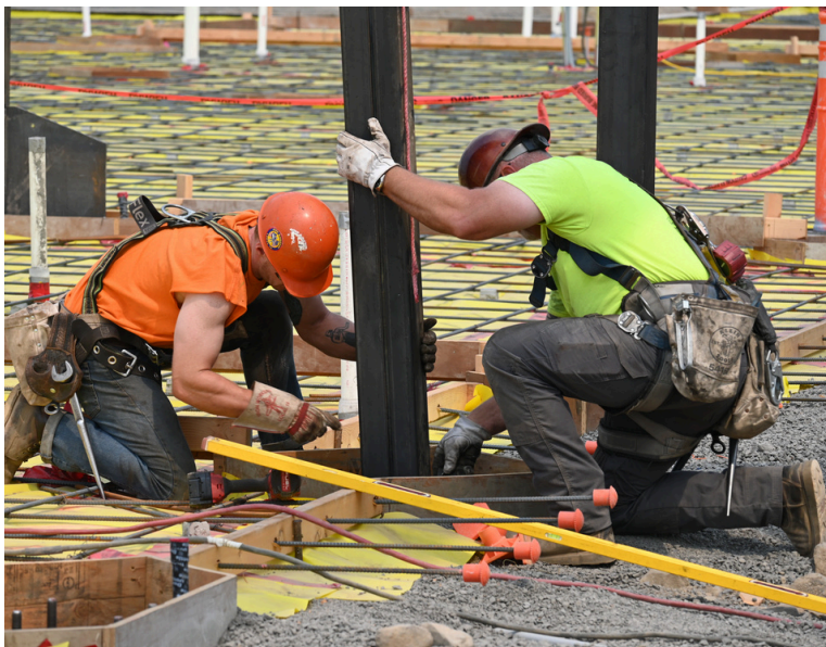
Construction crews work to erect the structural steel on Aug. 12.
