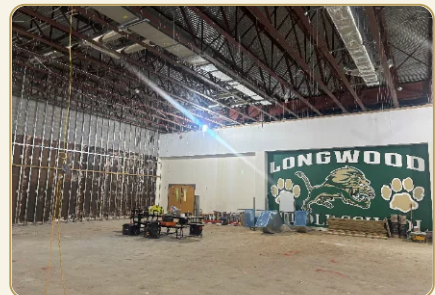
MIDDLE SCHOOL • ACTIVITY COURT RENOVATION
