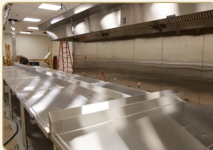
CTE CENTER • INTERIOR CONSTRUCTION
