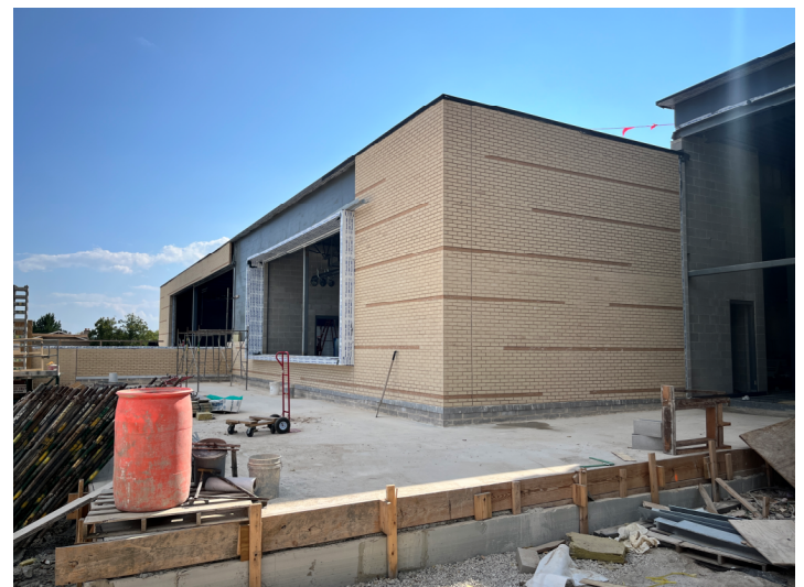
Brick Veneer Installed – Area B1 Patio
