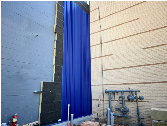
Metal Panels Started – North Elevation Of Area A2
