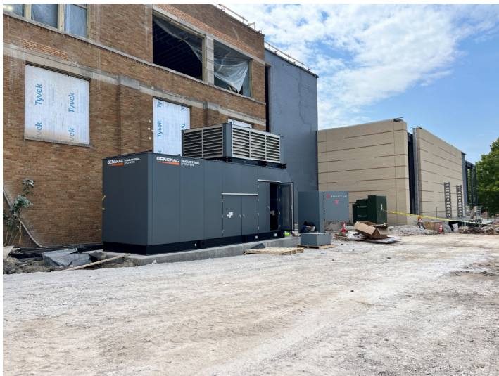
Generator & Transformer Installed – North Of Area A
