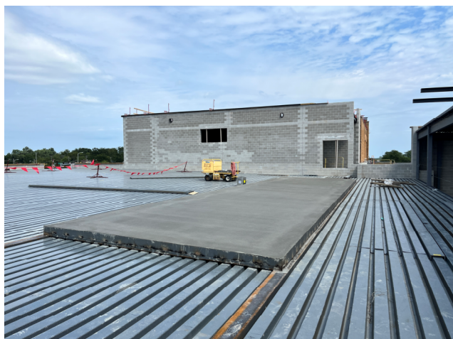
Chiller Pad Poured – Area C2 Roof
