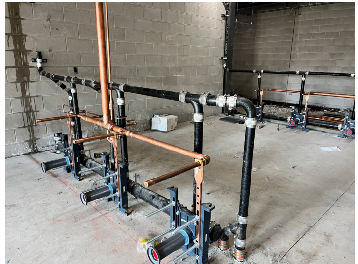
New Plumbing – Area B1 Ground Level Locker Rooms
