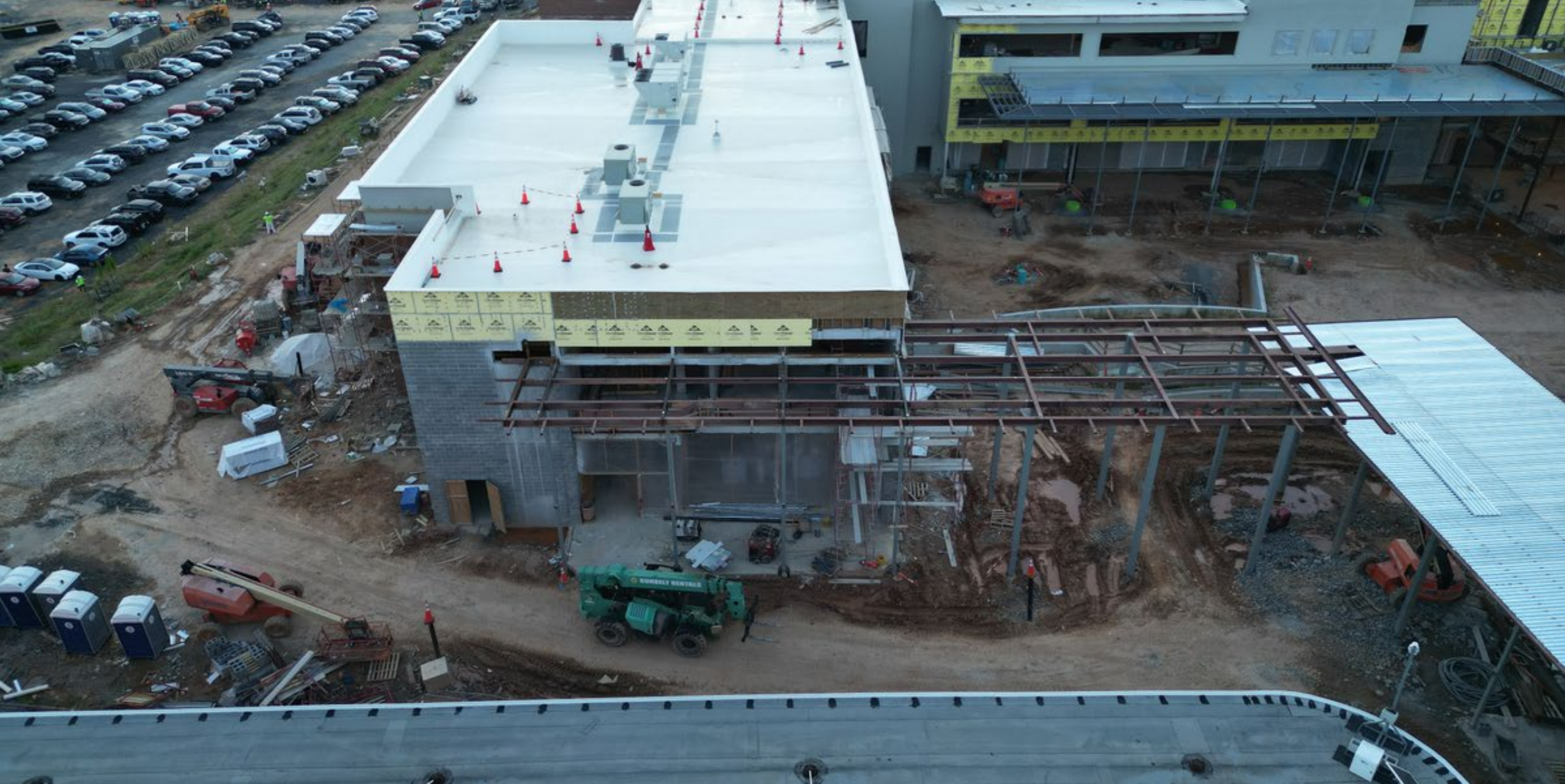
Area 2- Entrance Canopy steel structure
