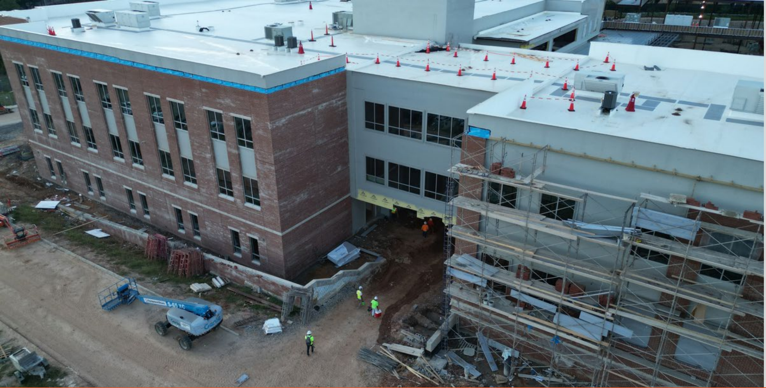
Area 2/3- Breezeway- Exterior Brick work
