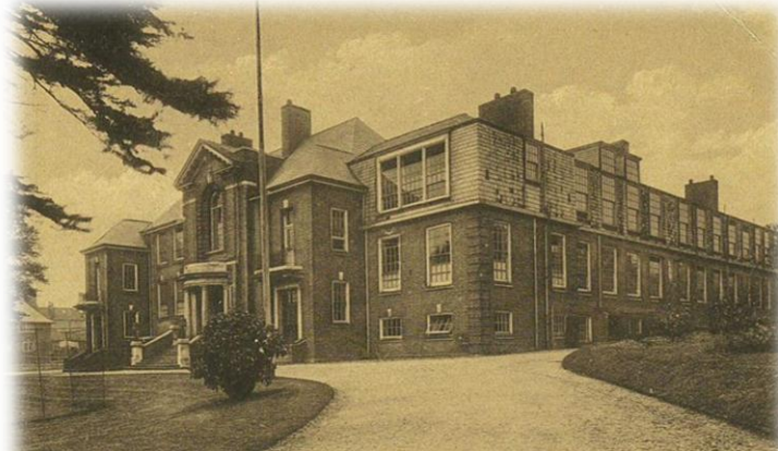
County Secondary School, Sydenham
