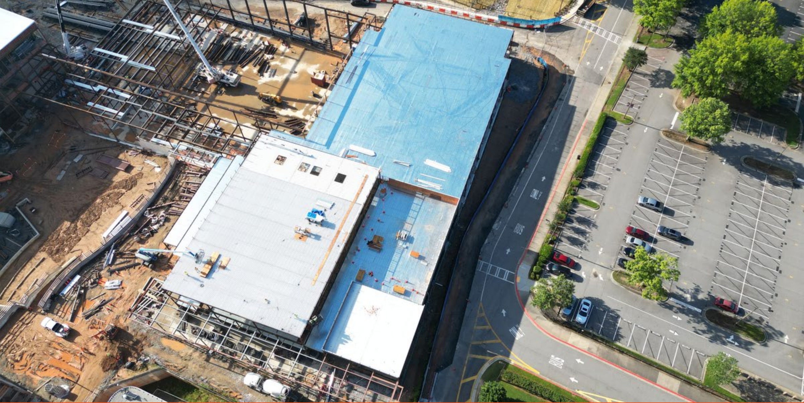
Area 7 & 8- Roof Progress
