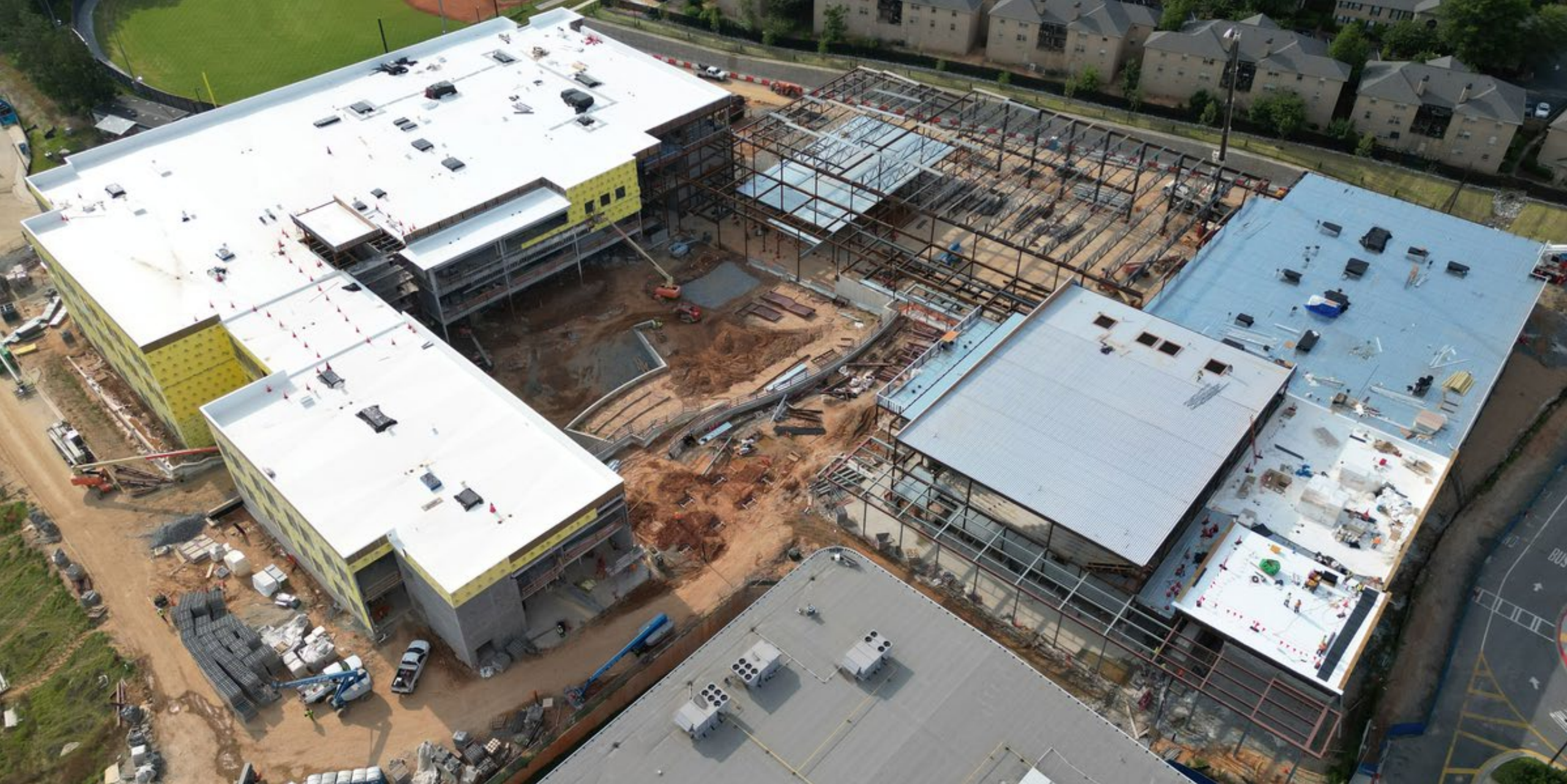
Overall Site Progress
