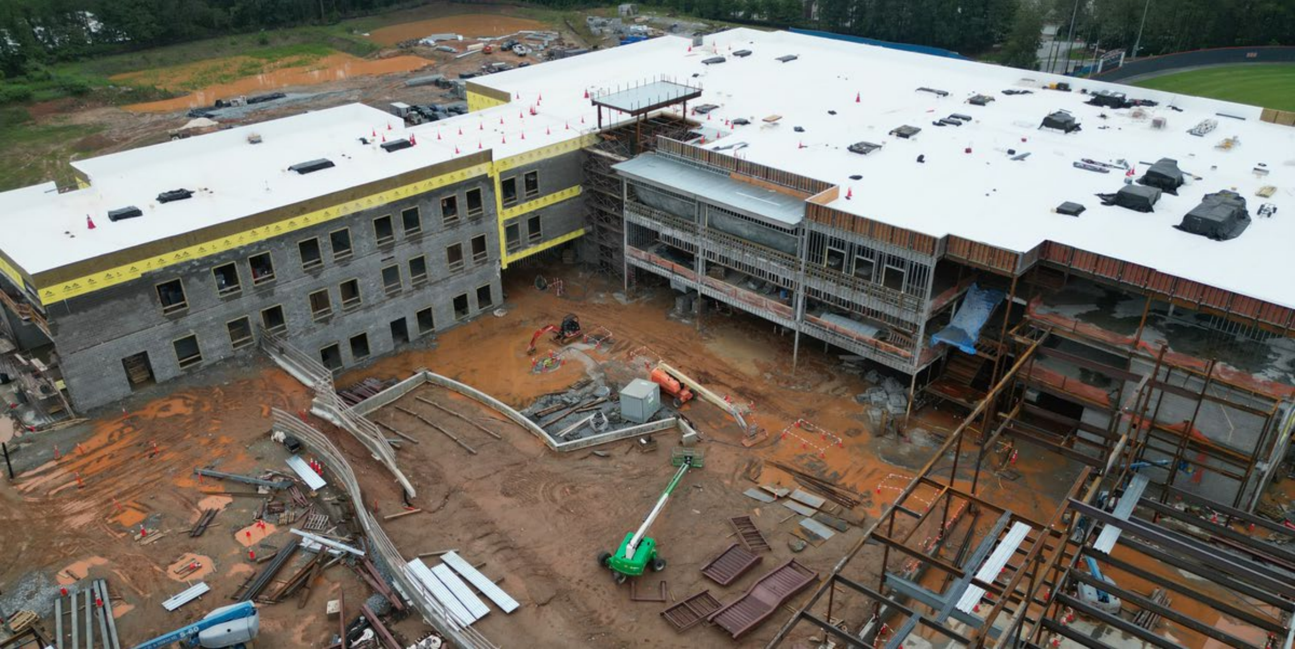
External Framing and Masonry
