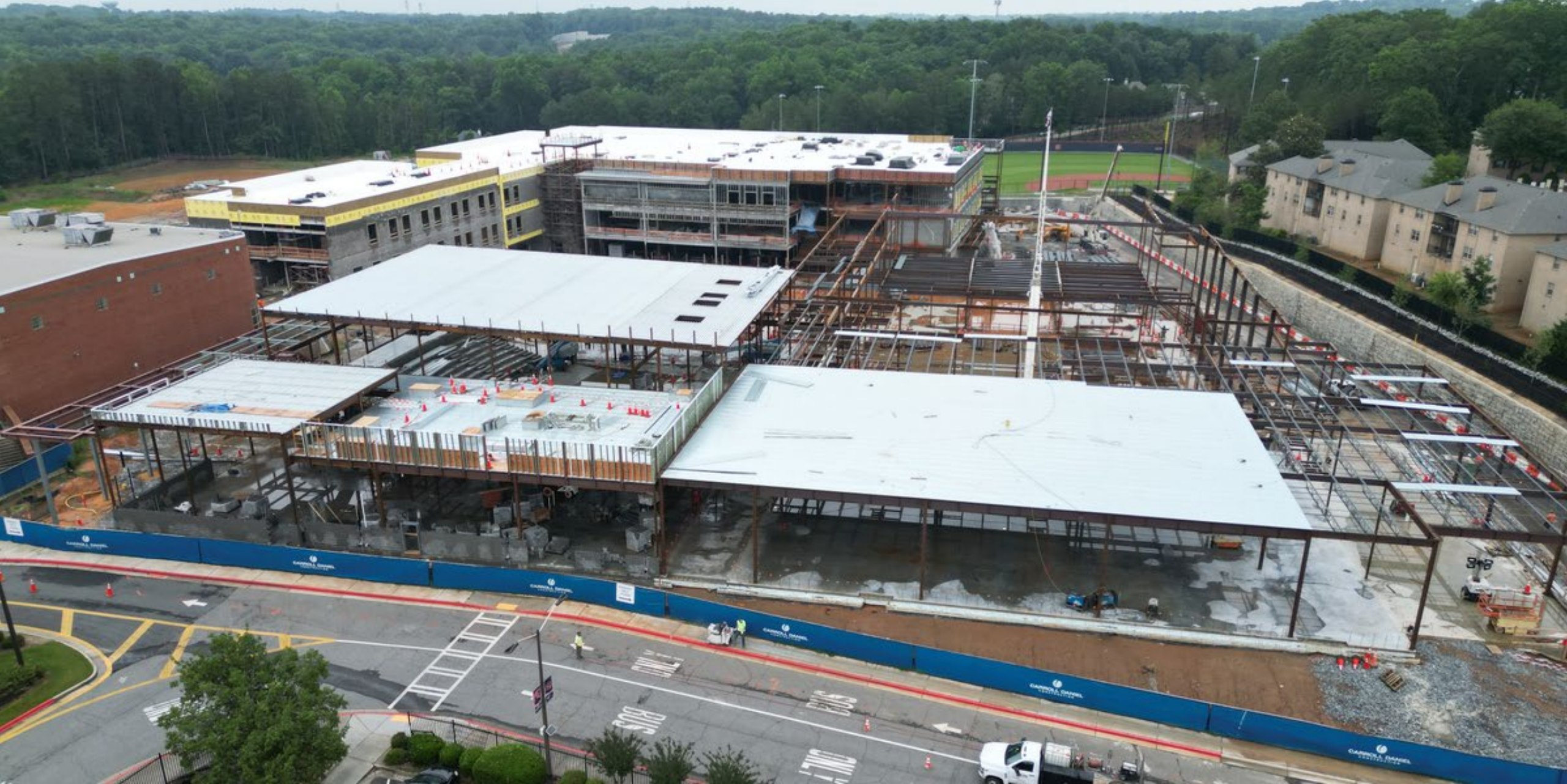
Area 6,7 and 8 Steel Erection and roof in progress
