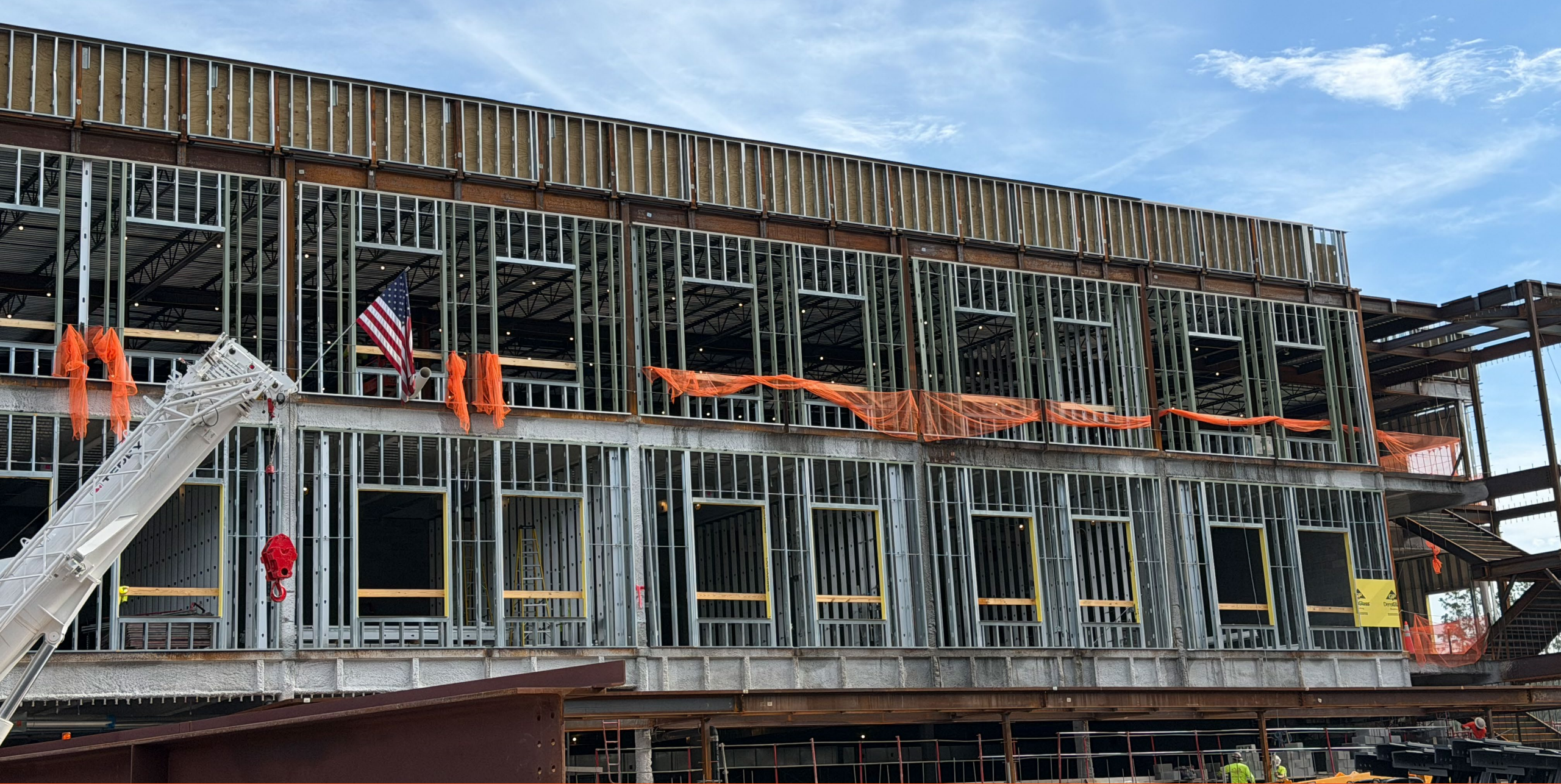
External Framing- South Elevation
