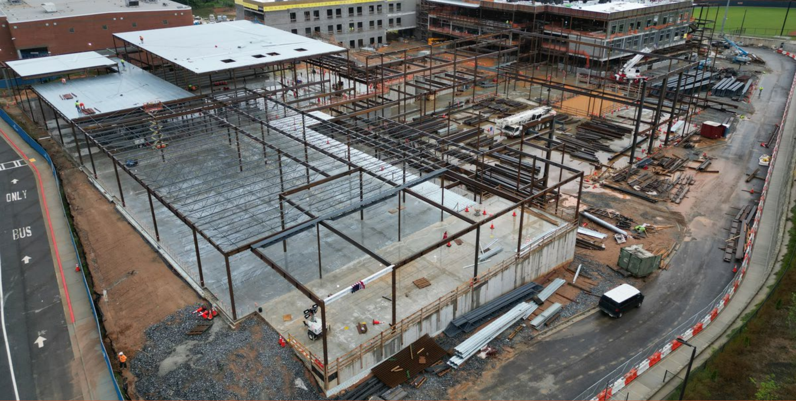
Area 6,7 and 8 Steel Erection
