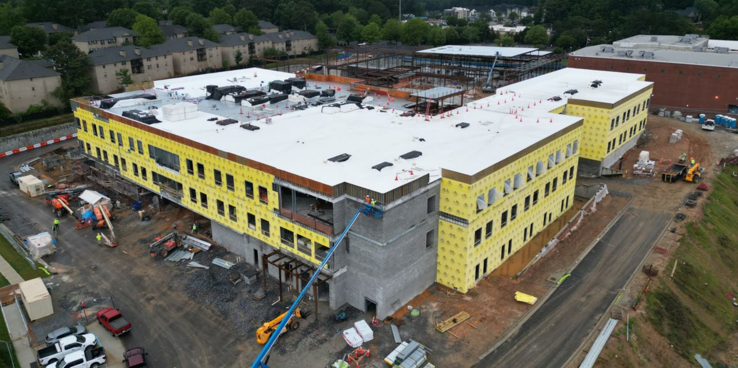
Sheathing- East and North Elevation
