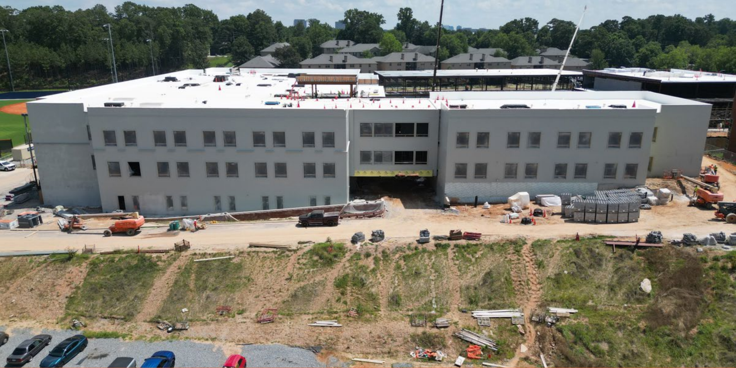
North Elevation- Exterior Air Barrier in progress
