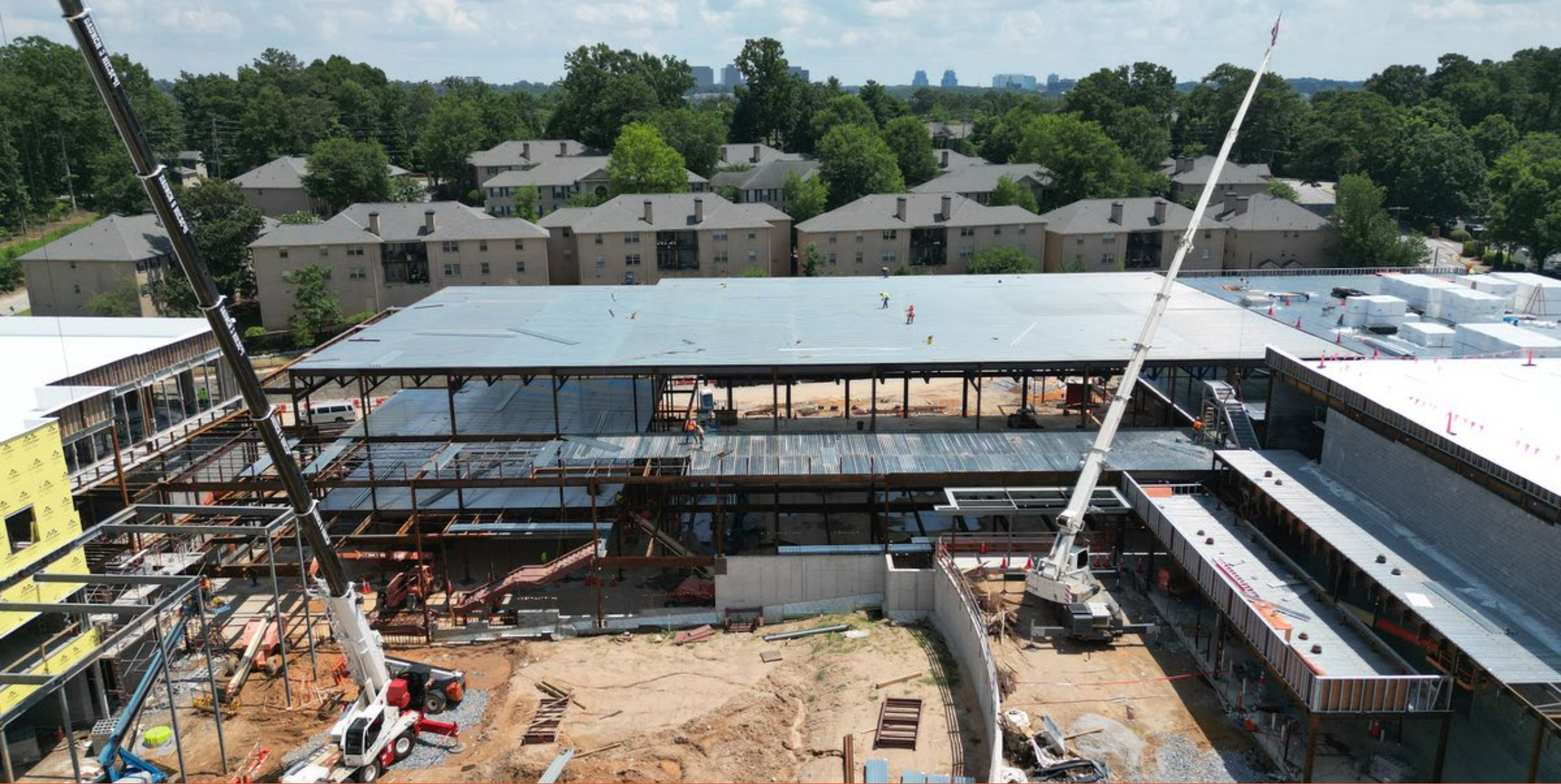
Gym Roof in Progress
