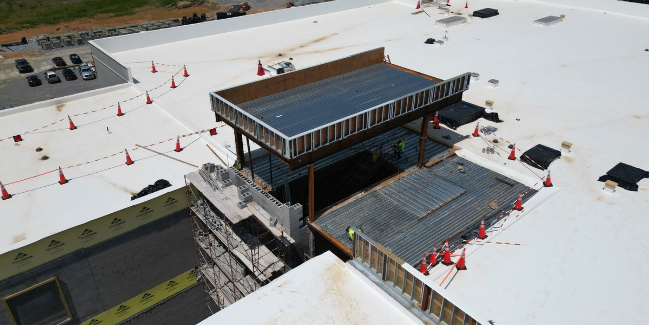
Area 2/3- Roof Canopy in progress
