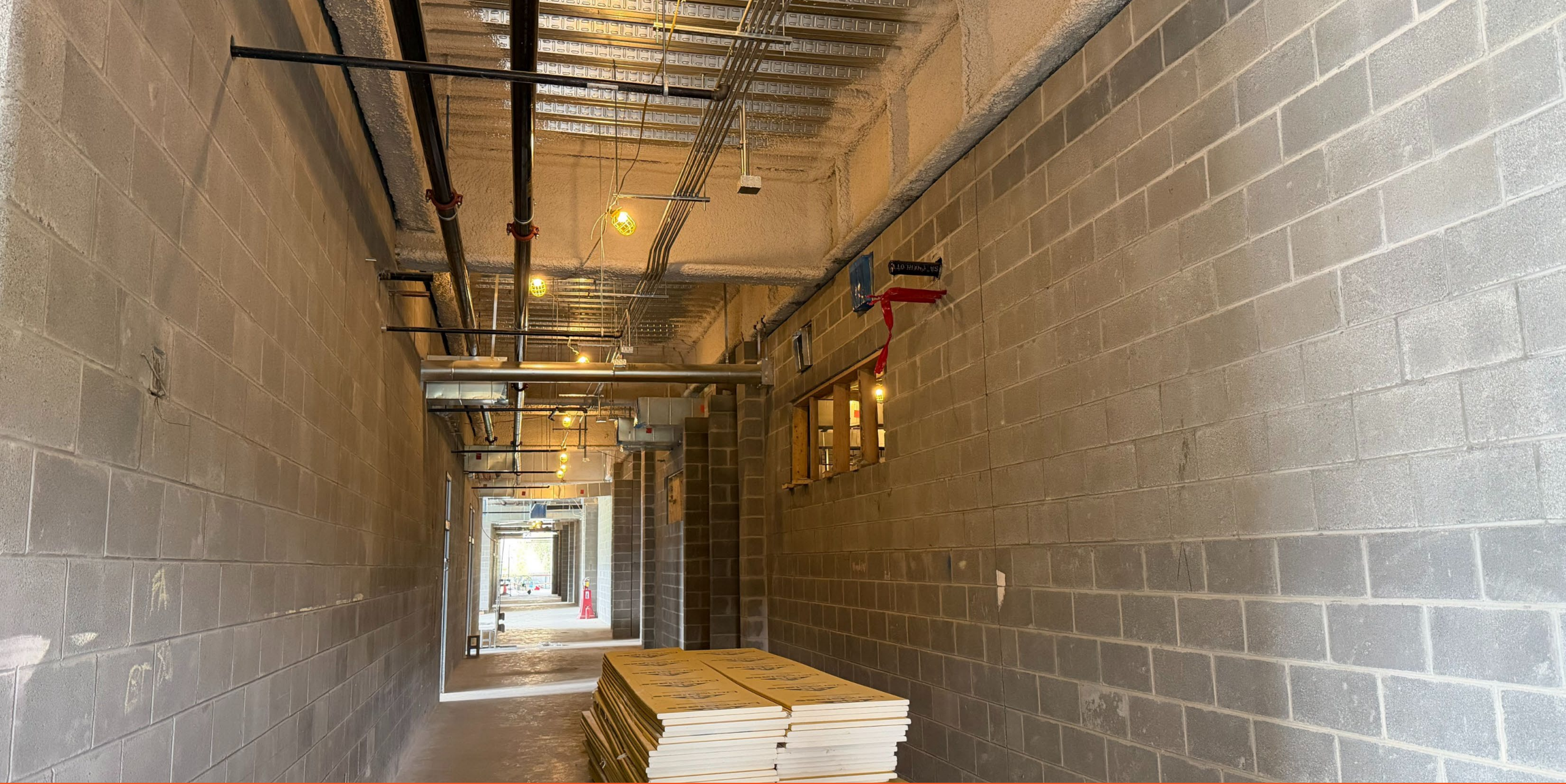
Level 3- Interior Masonry
