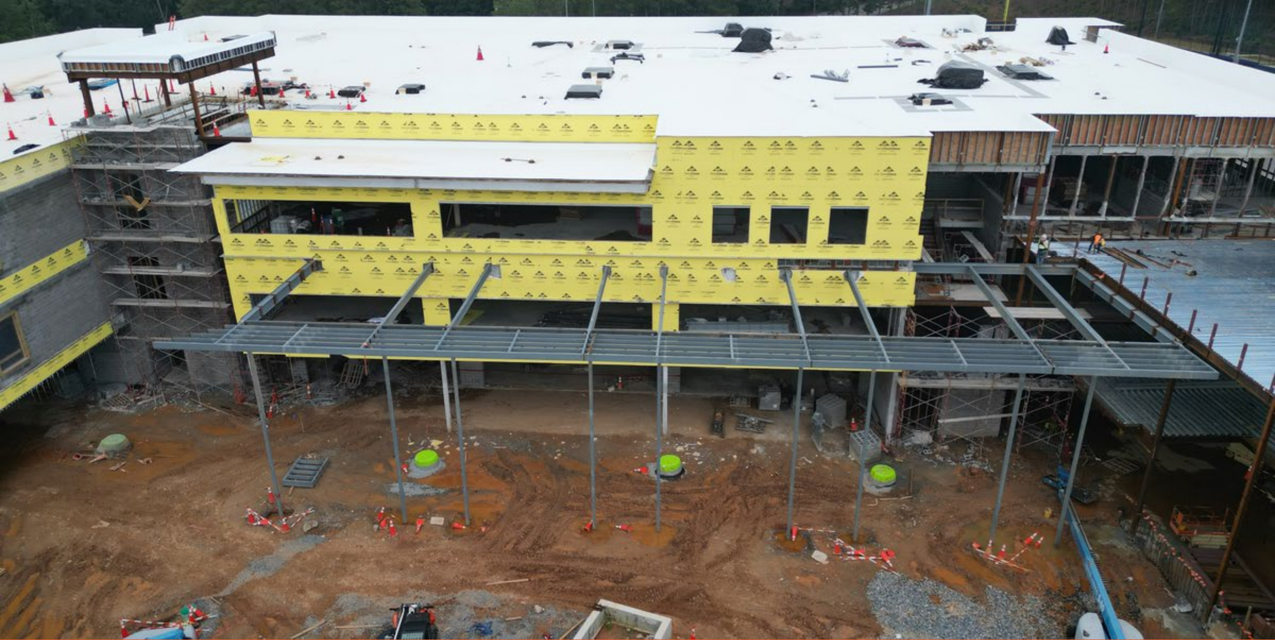
Canopies in Courtyard- In Progress
