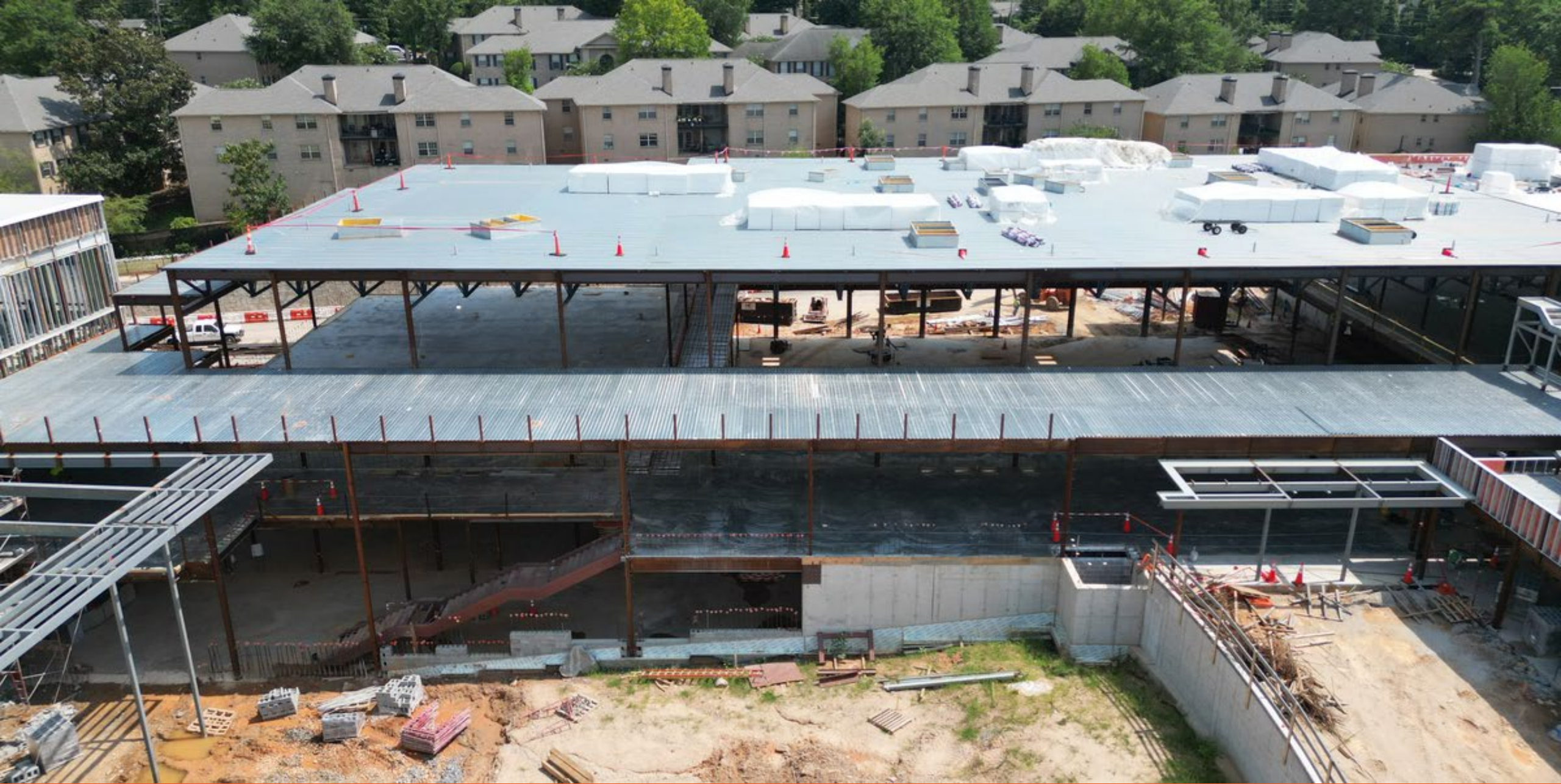
Area 6/7 Gym- Roof Work
