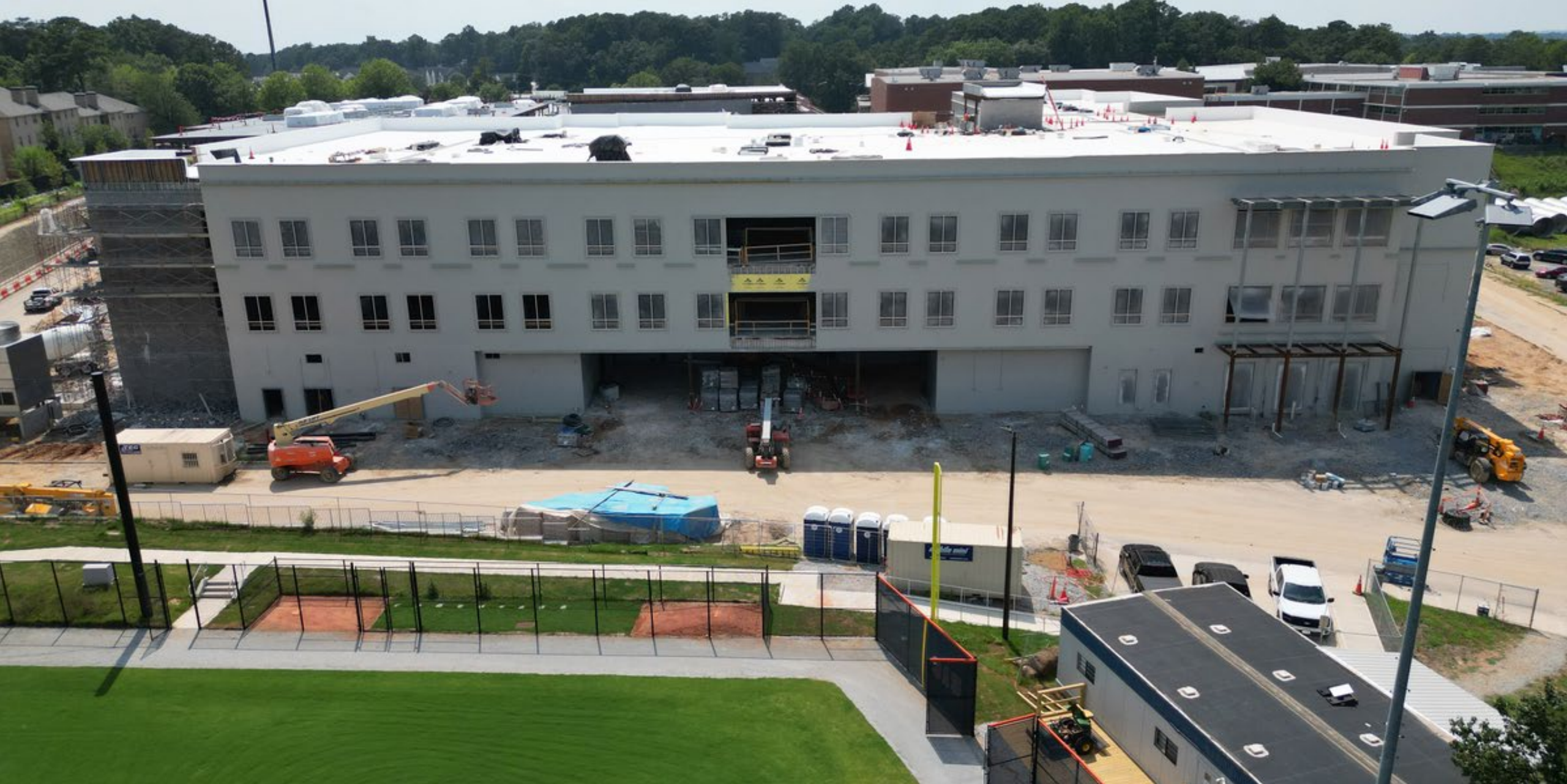
Area 4/5- Exterior Air Barrier
