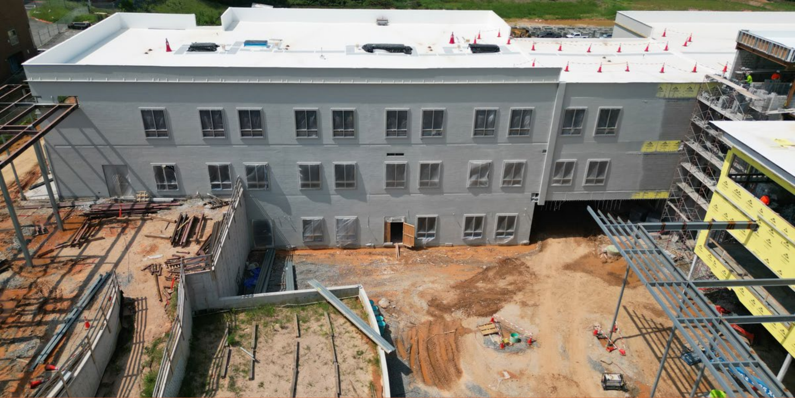
Area 2- South- Exterior Air Barrier
