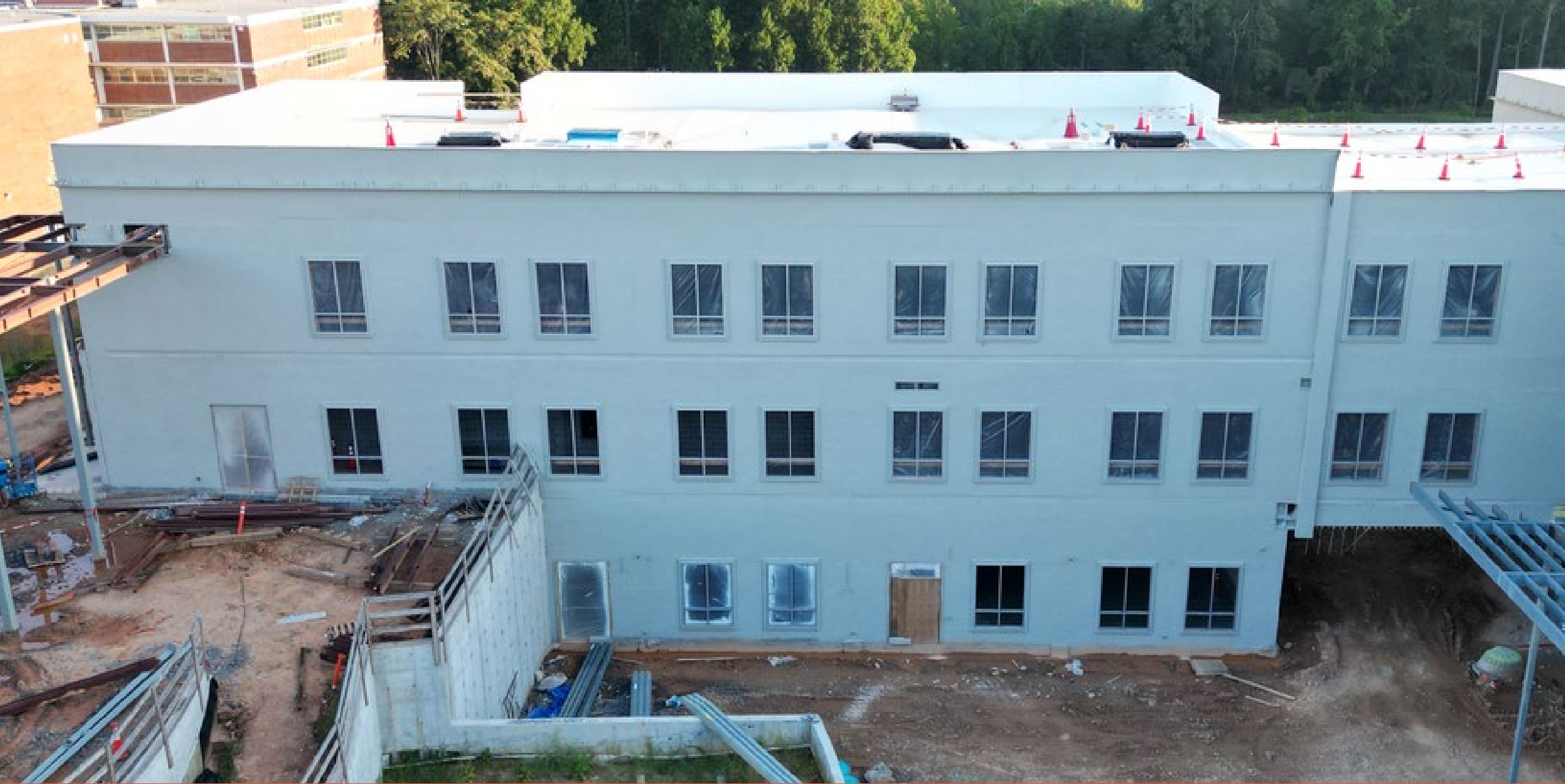
Area 2- South- Window Frame installation
