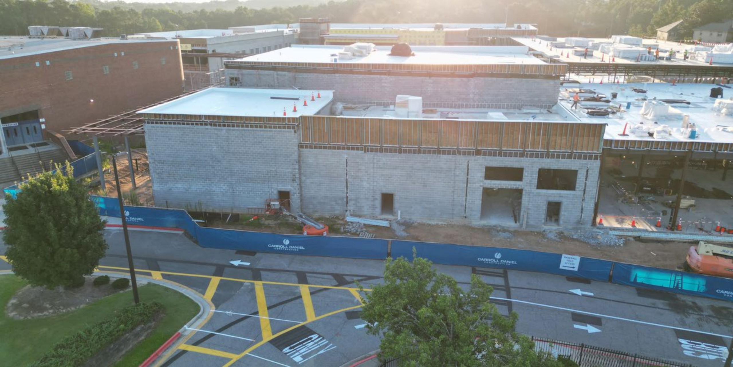
Area 8- CMU Block Work, Roof and Steel Canopies
