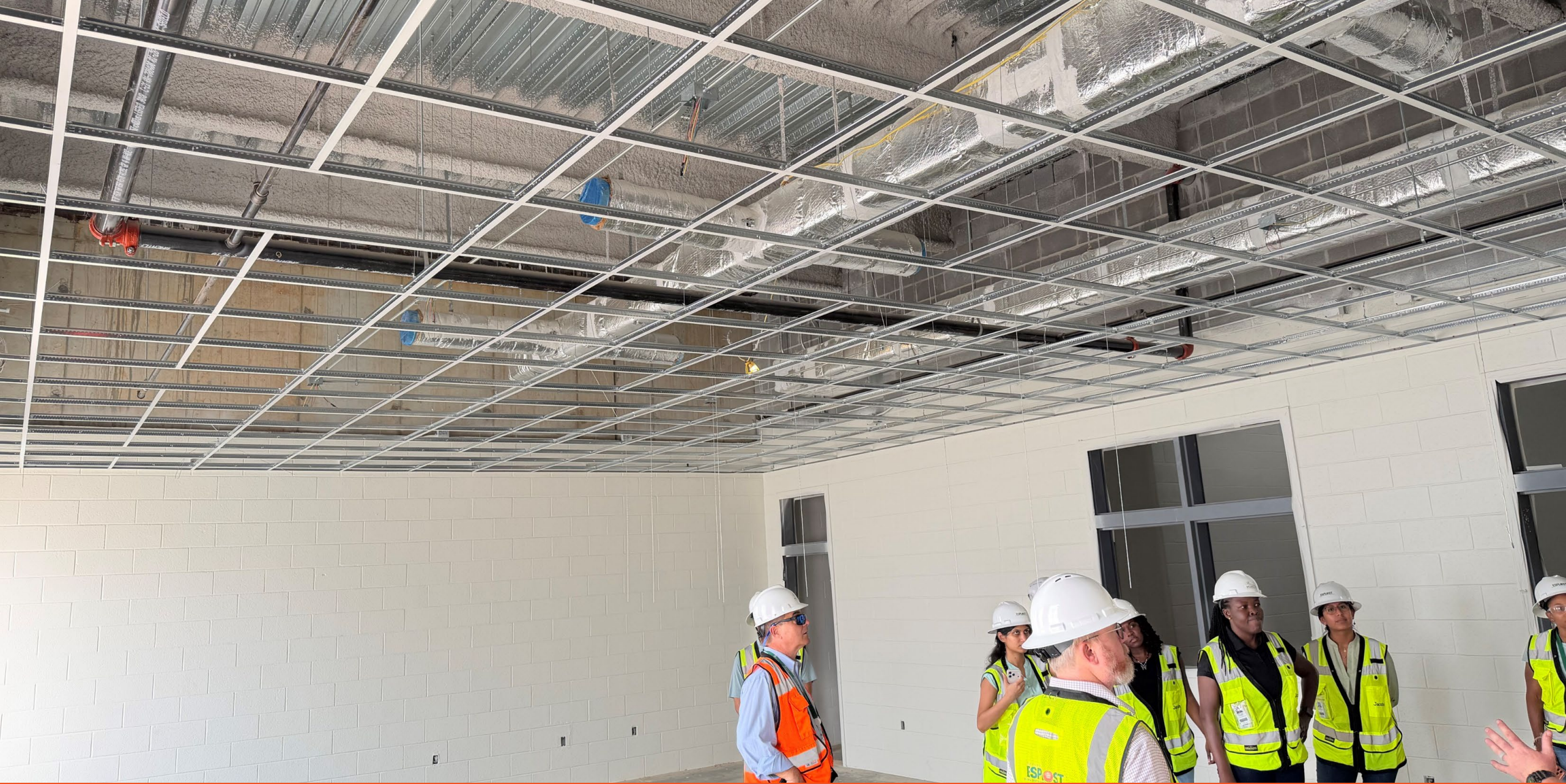
Area 2- Ceiling Grid installation and Paint
