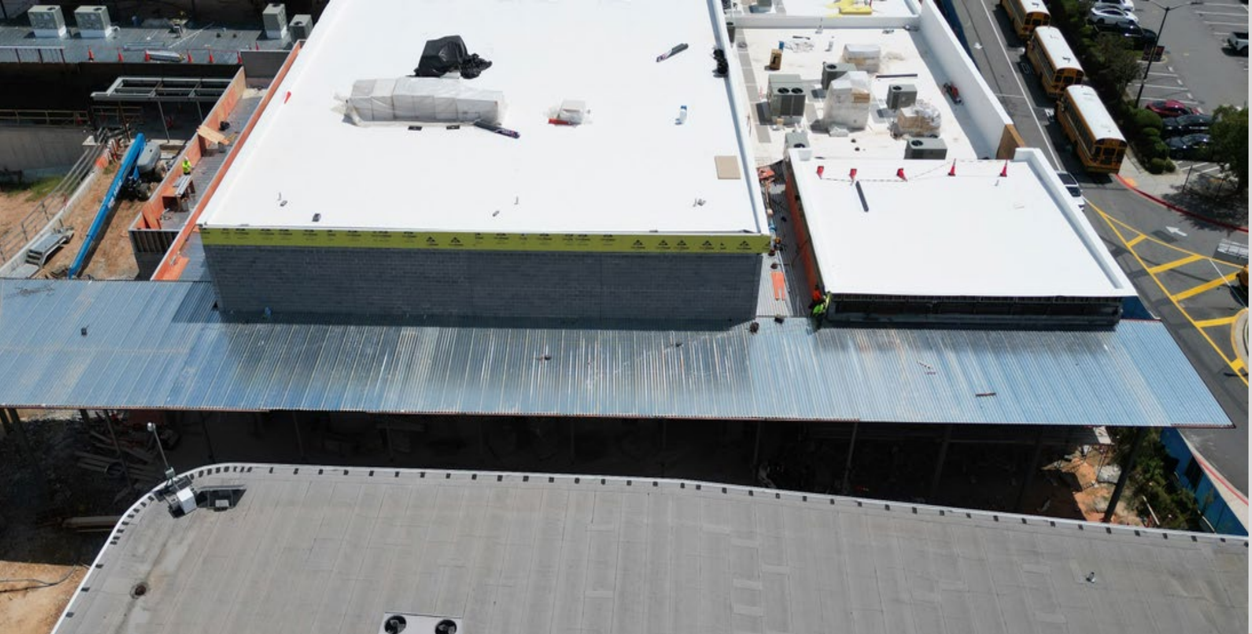
Area 8- Auditorium- Steel Canopy
