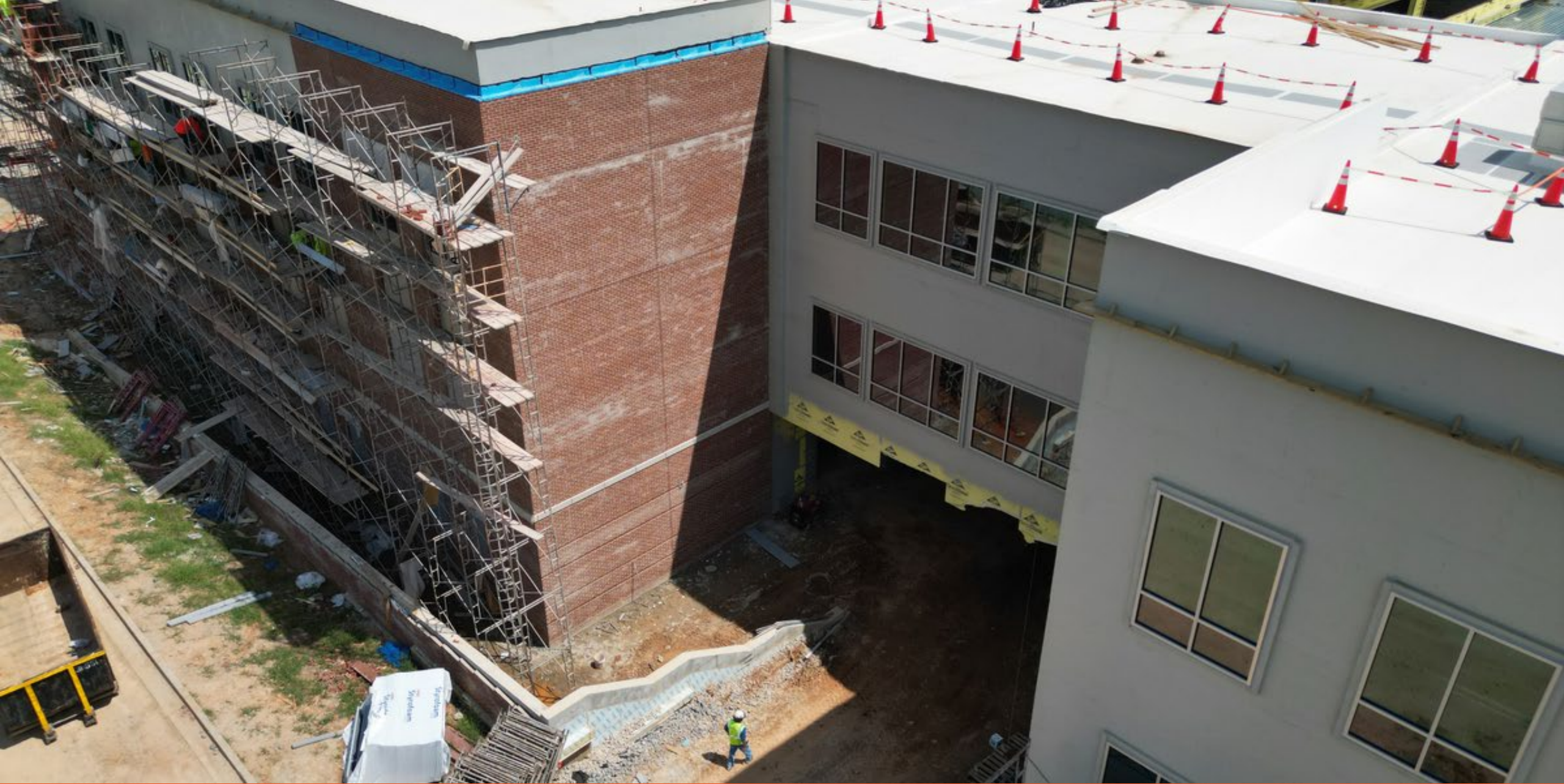
Area 2- North Elevation- Ex. Brick and Window Glass installation
