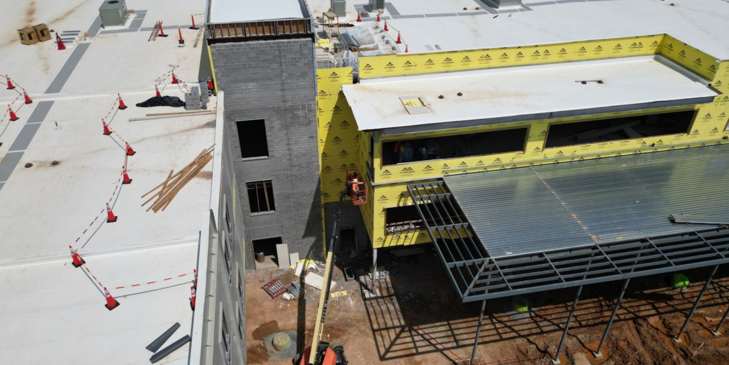
Area 3- Steel canopy installation in the courtyard.
