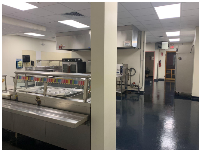
Renovated Kitchen ready to re-occupy
