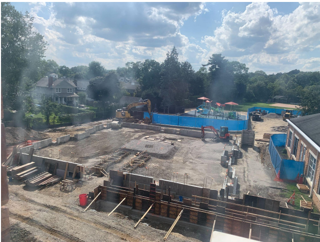
New addition interior footings being formed
