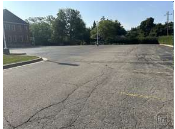
Rear parking lot
