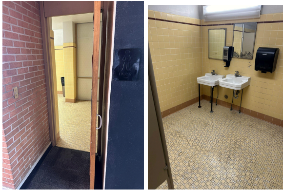
POD Bathrooms - not ADA compliant, fixtures original to the building
