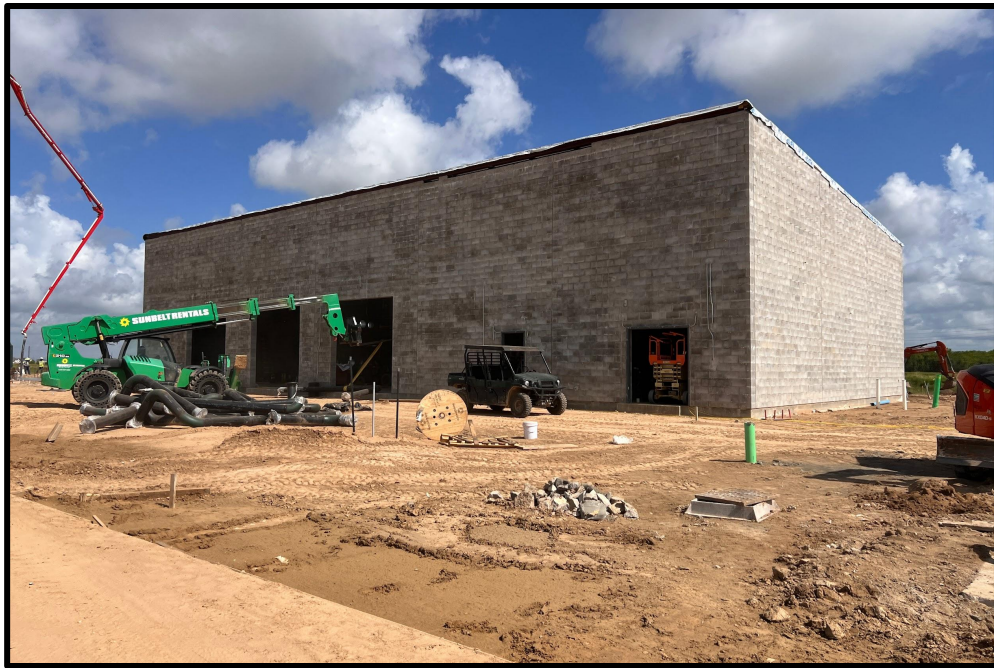
Central Plant Exterior CMU and Lightweight Roof
