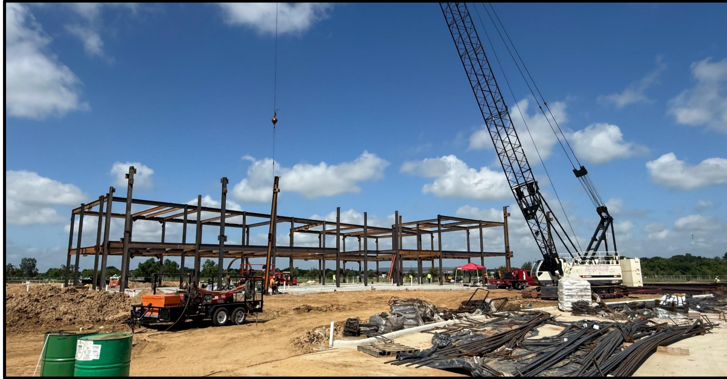
Area E Steel Erection
