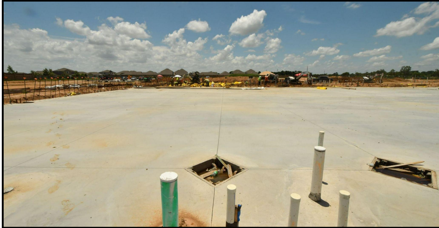
Area B Slab
