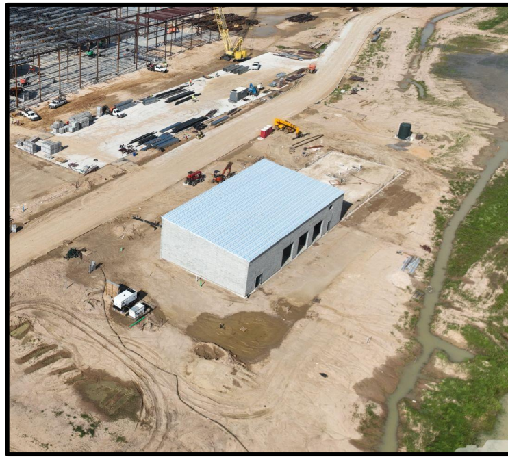
Central Plant Exterior CMU and Lightweight Roof
