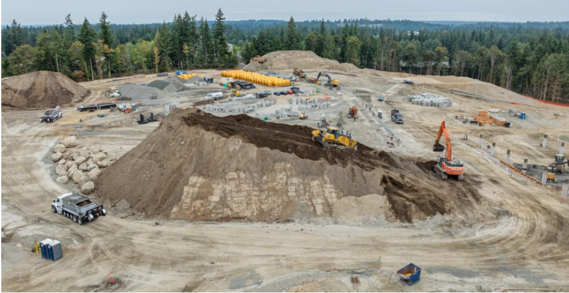
View of the site showing several of the large stockpiles of dirt that is being moved around the site (Drone photo taken 8/17/26)
