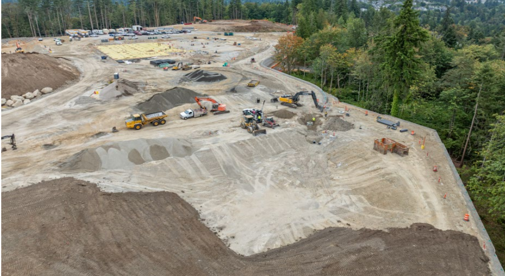
Retaining wall work along the south end of the site nearing completion (Drone photo taken 8/17/26)
