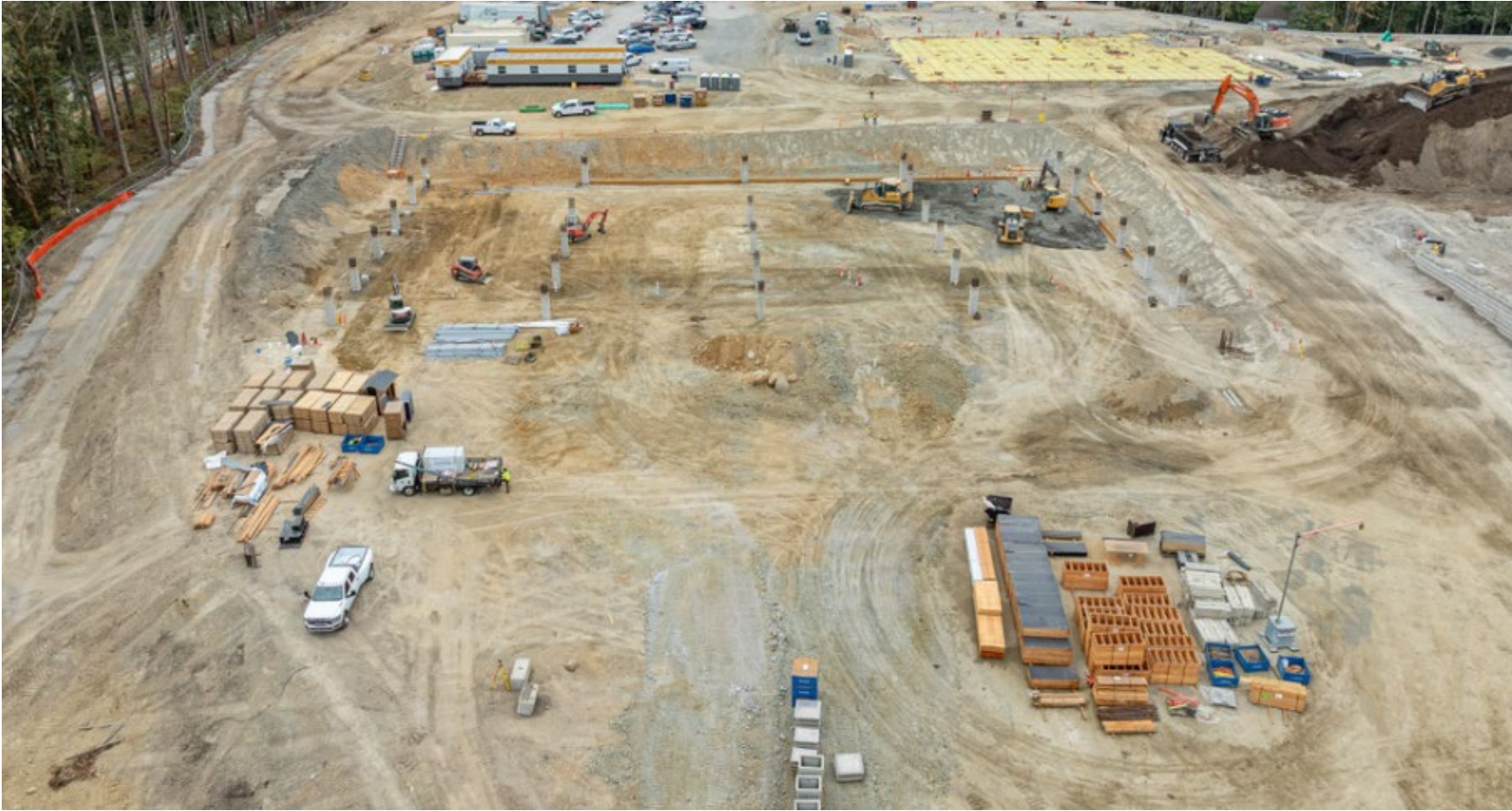
Footings and columns for the new parking garage installed (Drone photo taken 8/17/26)
