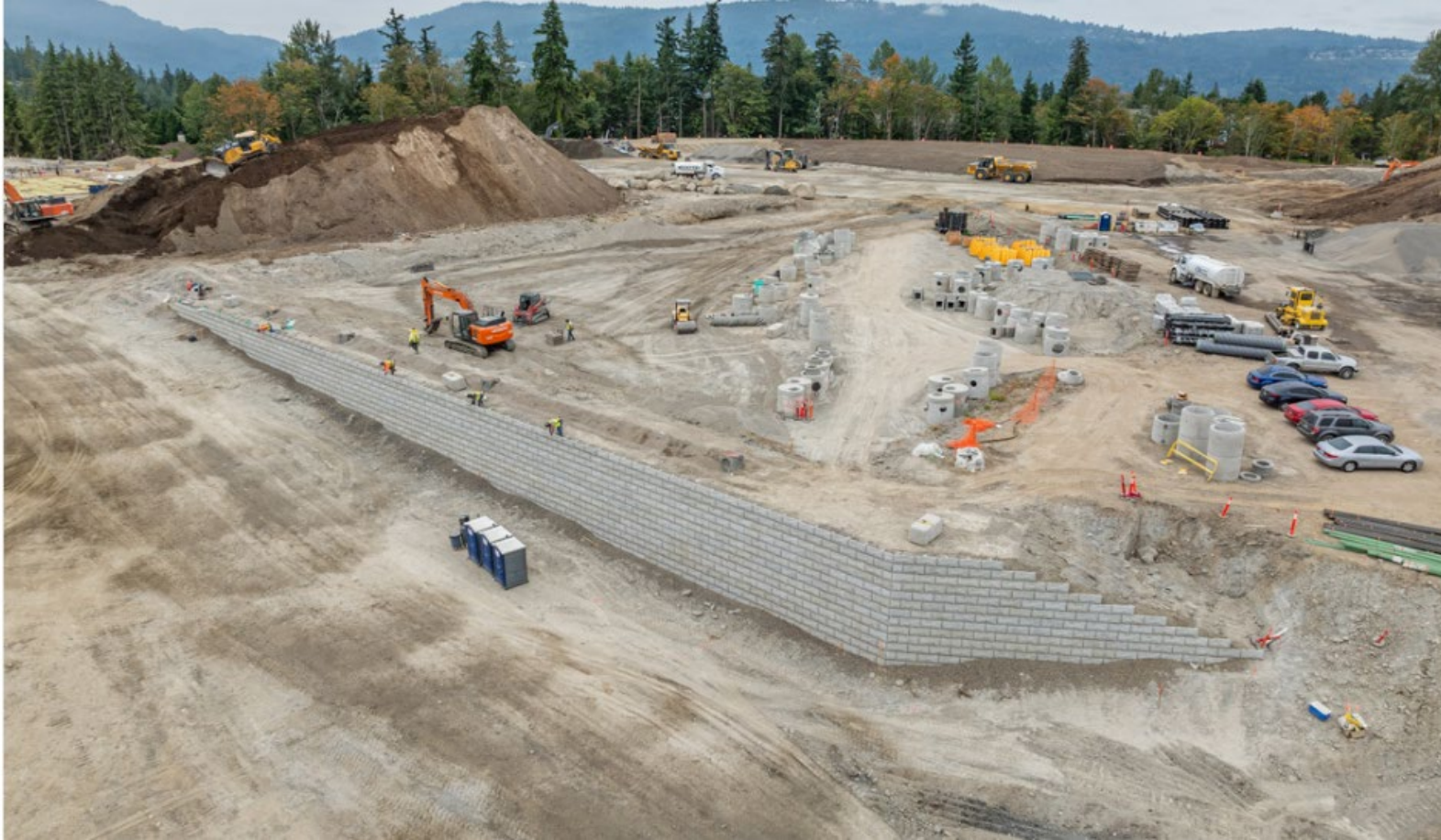
Retaining wall that “holds-up” the sports field well underway (Drone photo taken 8/173/26)
