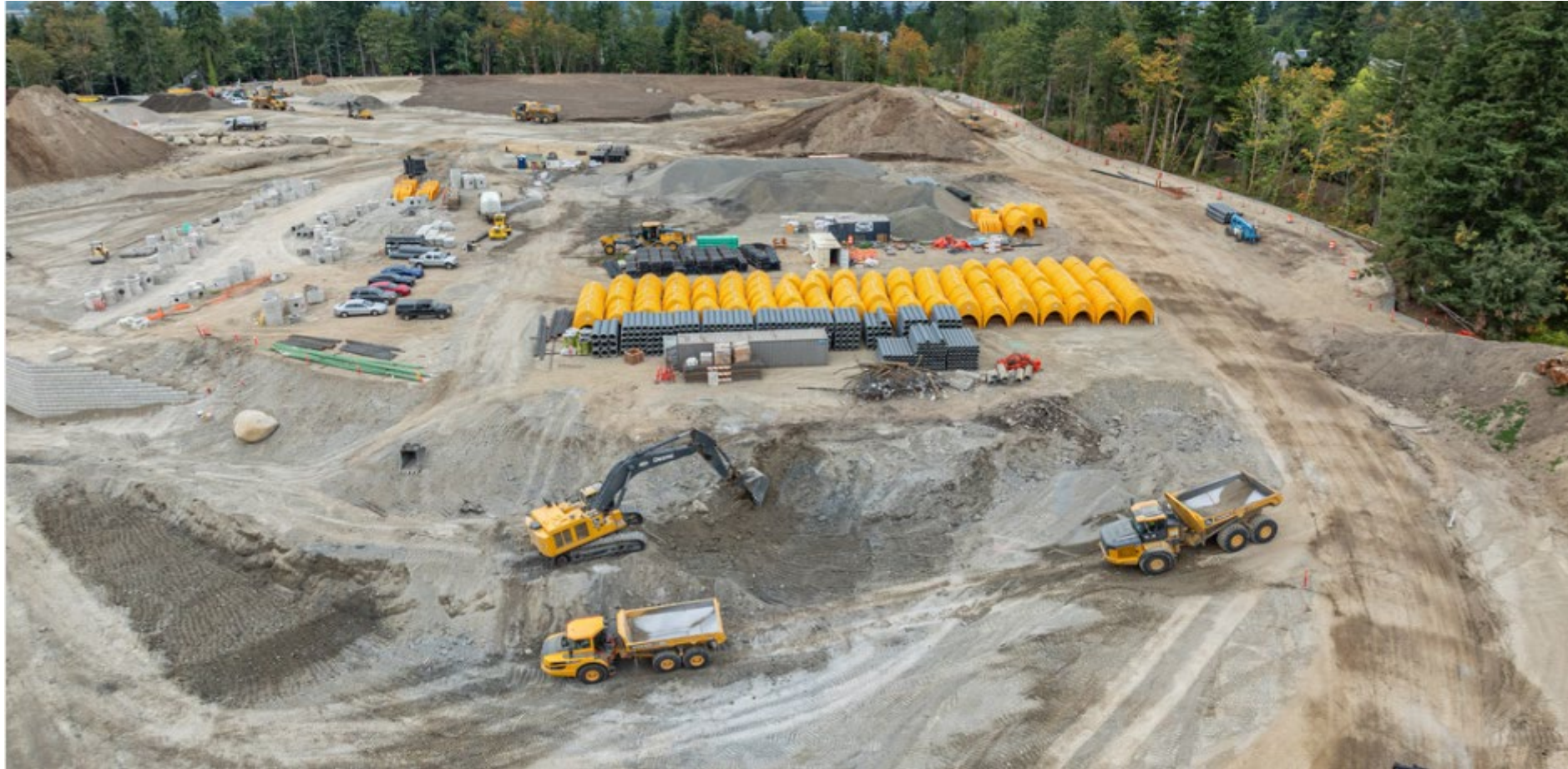
View showing stockpiles of underground utilities materials including underground stormwater storage system (yellow), as well as stormwater catch basins, sewer manholes and pipe (Drone photo taken 8/17/26)
