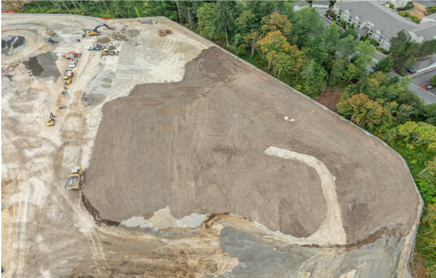
Retaining wall work along the west side of the site nearing completion (Drone photo taken 8/17/26)
