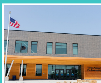
Tointon Academy of Pre-Engineering
