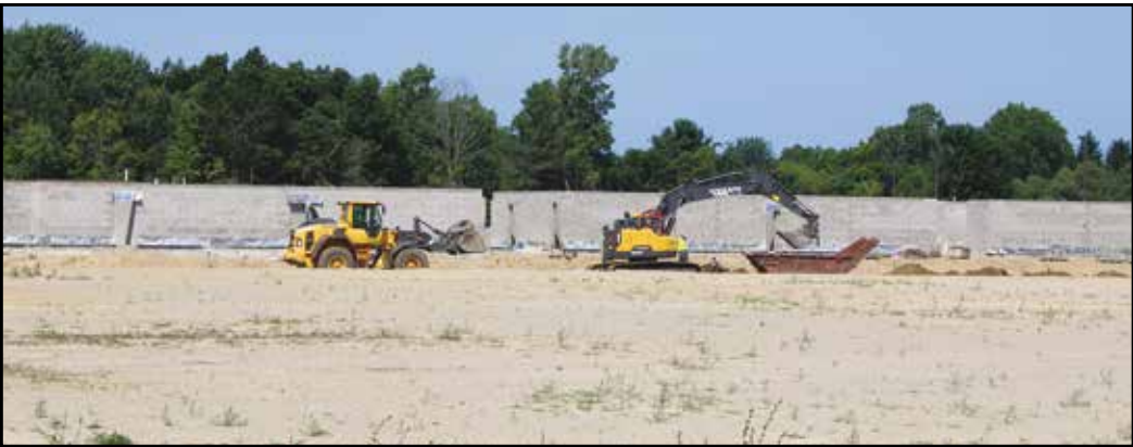
Construction well underway at the high school.
