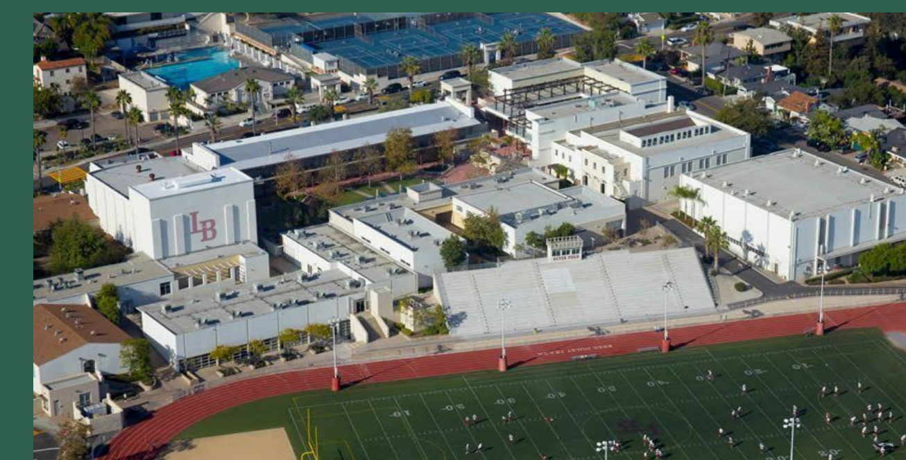
Laguna Beach High School - white cool roof
