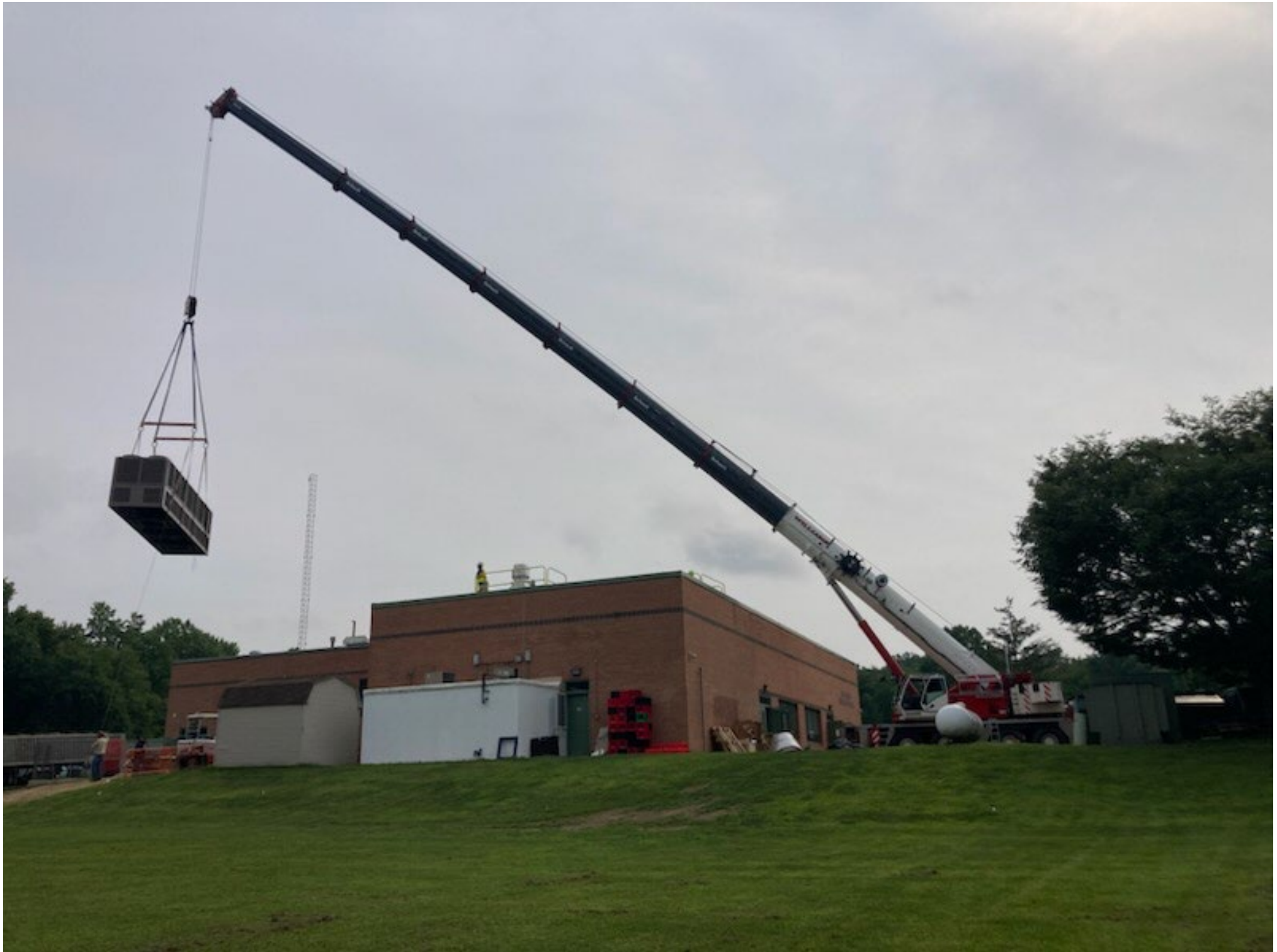
CECIL MANOR ELEMENTARY SCHOOL – HVAC REPLACEMENT
