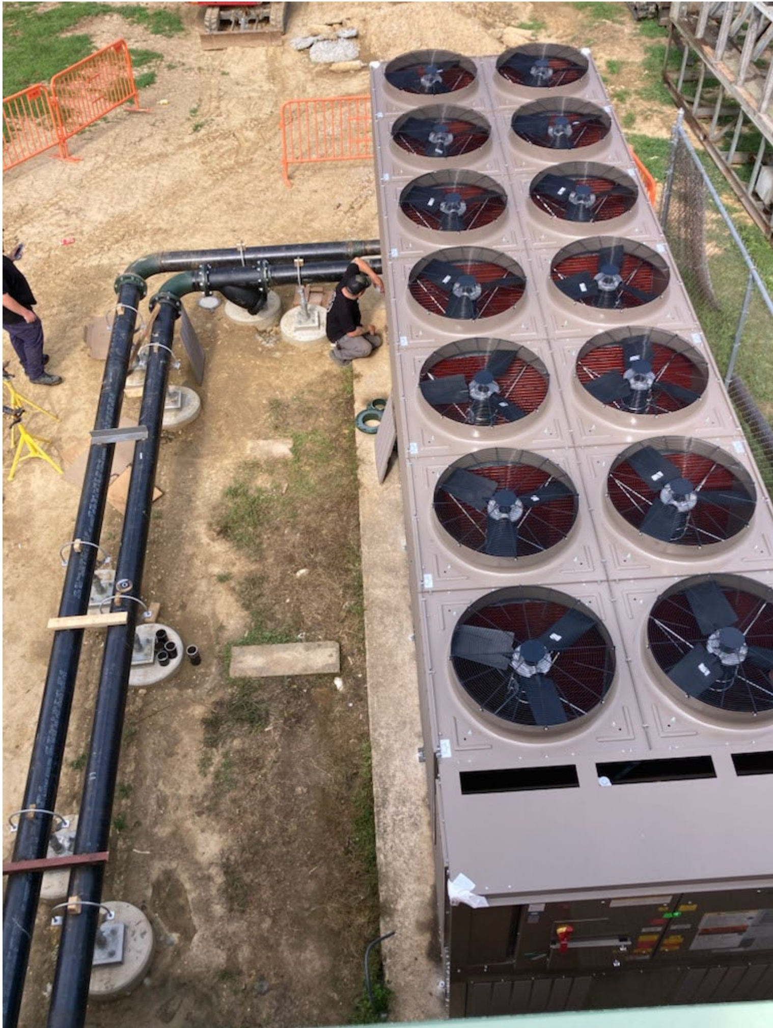
CECIL MANOR ELEMENTARY SCHOOL - HVAC REPLACEMENT
