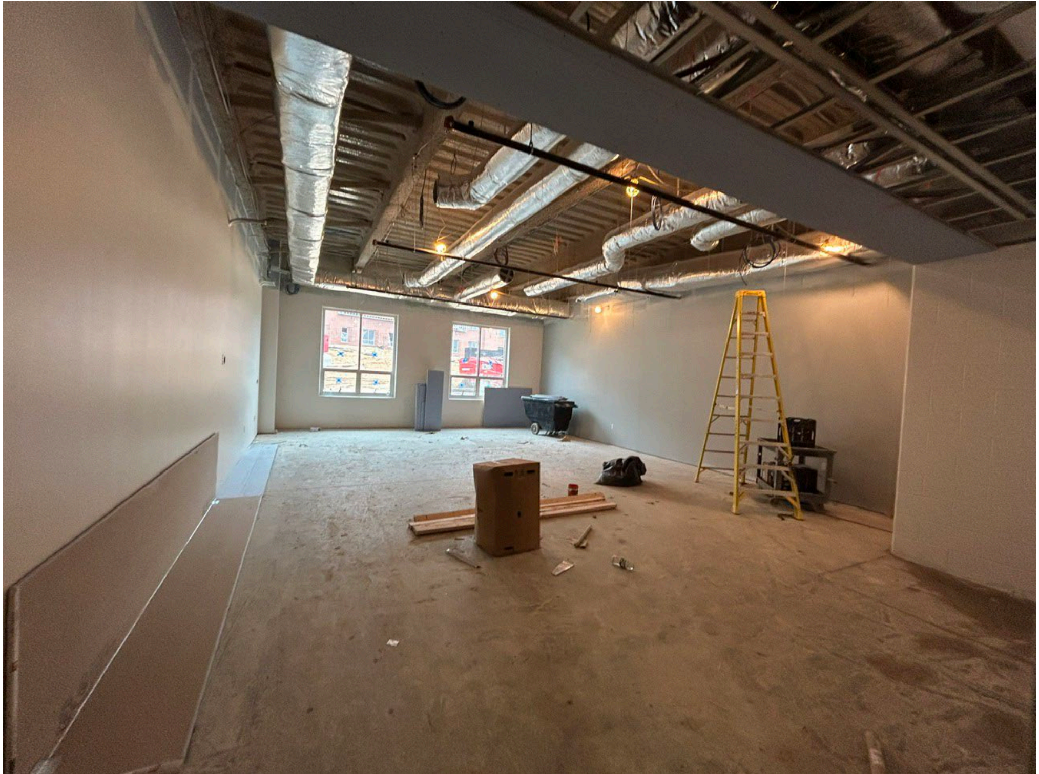
NORTH EAST MIDDLE / HIGH SCHOOL – REPLACEMENT – FRAMING, INSULATION, DRYWALL AND PAINTING
