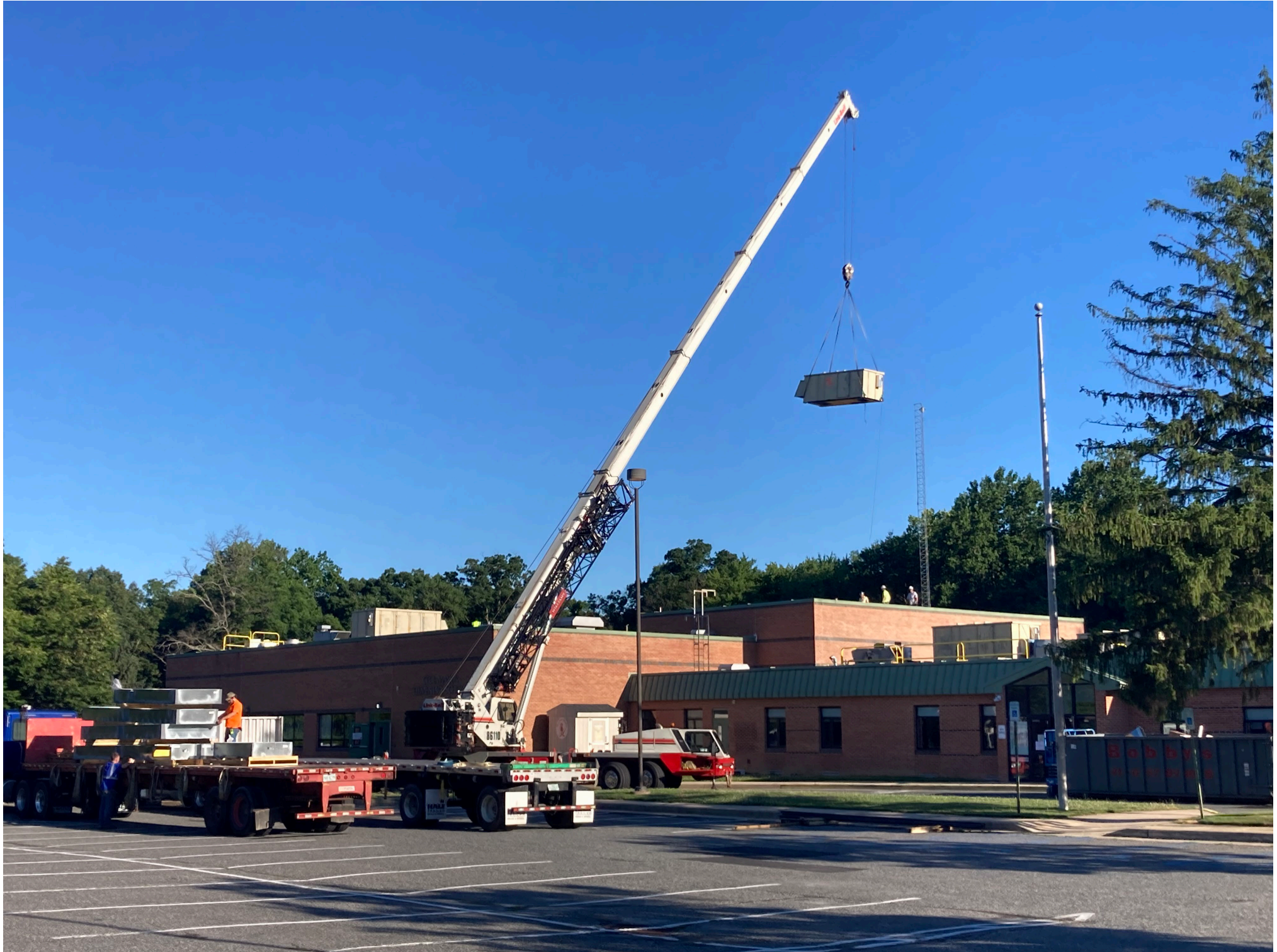
CECIL MANOR ELEMENTARY SCHOOL – HVAC REPLACEMENT
