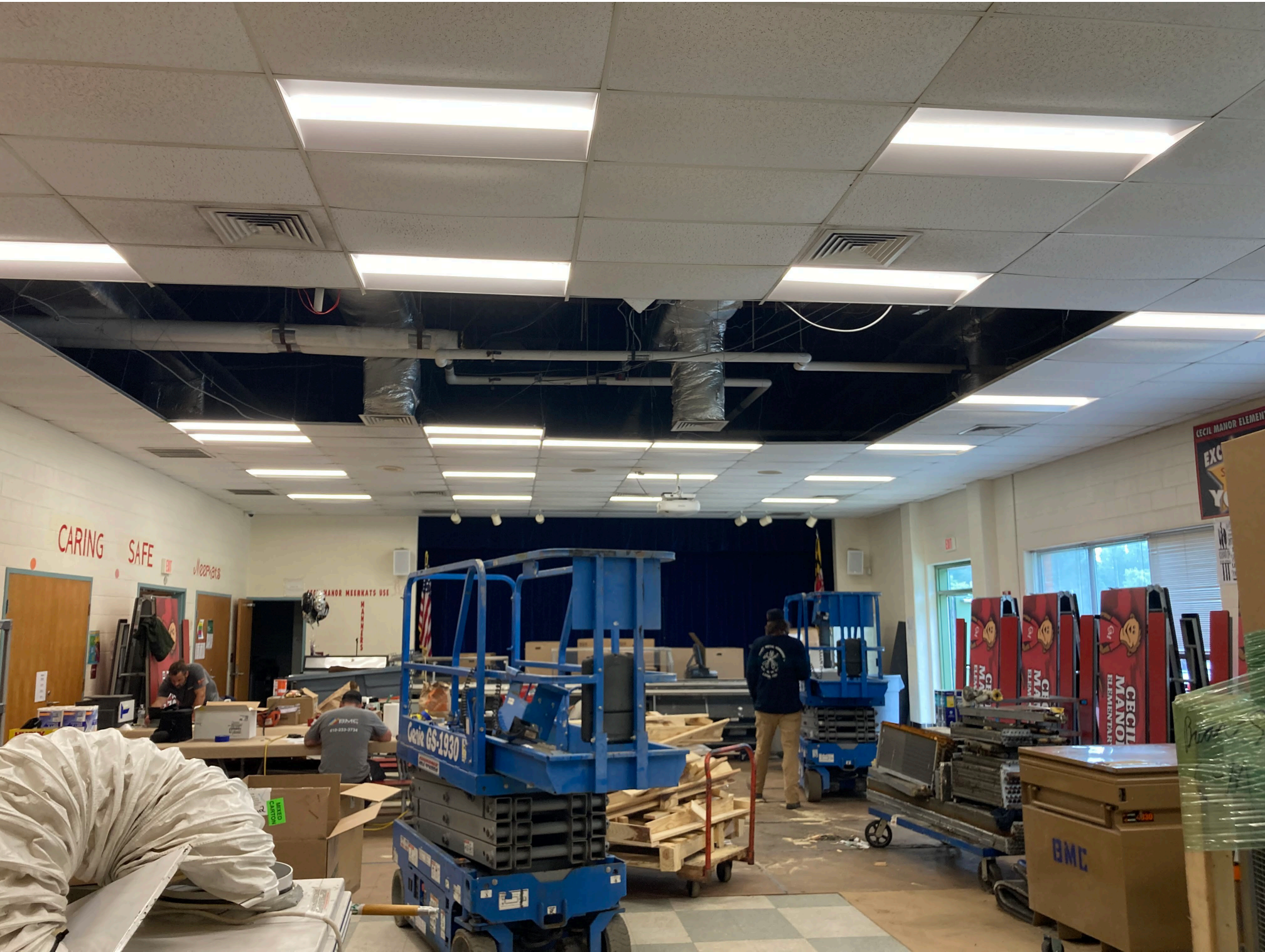
CECIL MANOR ELEMENTARY SCHOOL – HVAC REPLACEMENT
