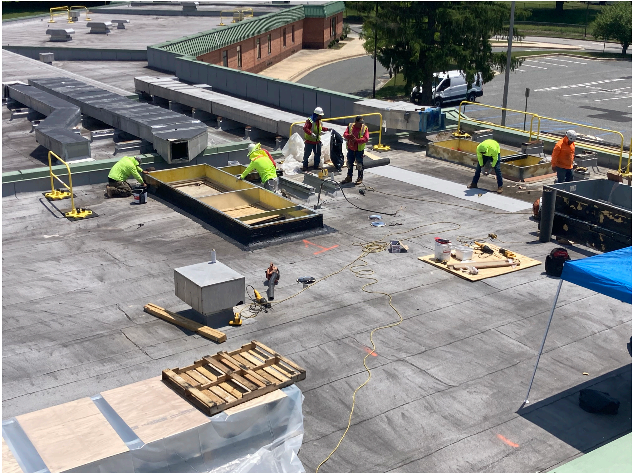
CECIL MANOR ELEMENTARY SCHOOL – HVAC REPLACEMENT
