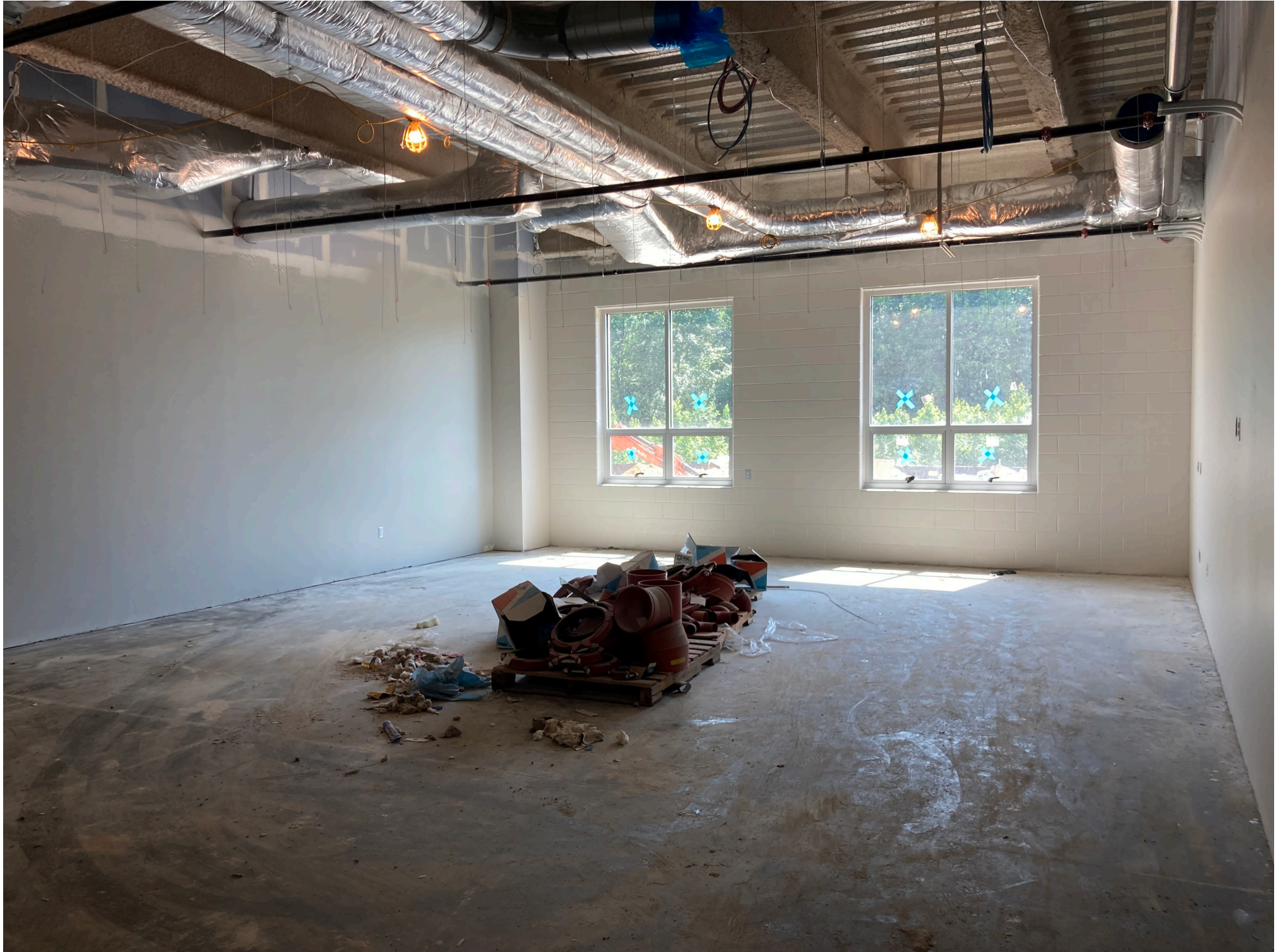
NORTH EAST MIDDLE / HIGH SCHOOL – REPLACEMENT – FRAMING, INSULATION, DRYWALL AND PAINTING CONTINUE THROUGHTOUT
