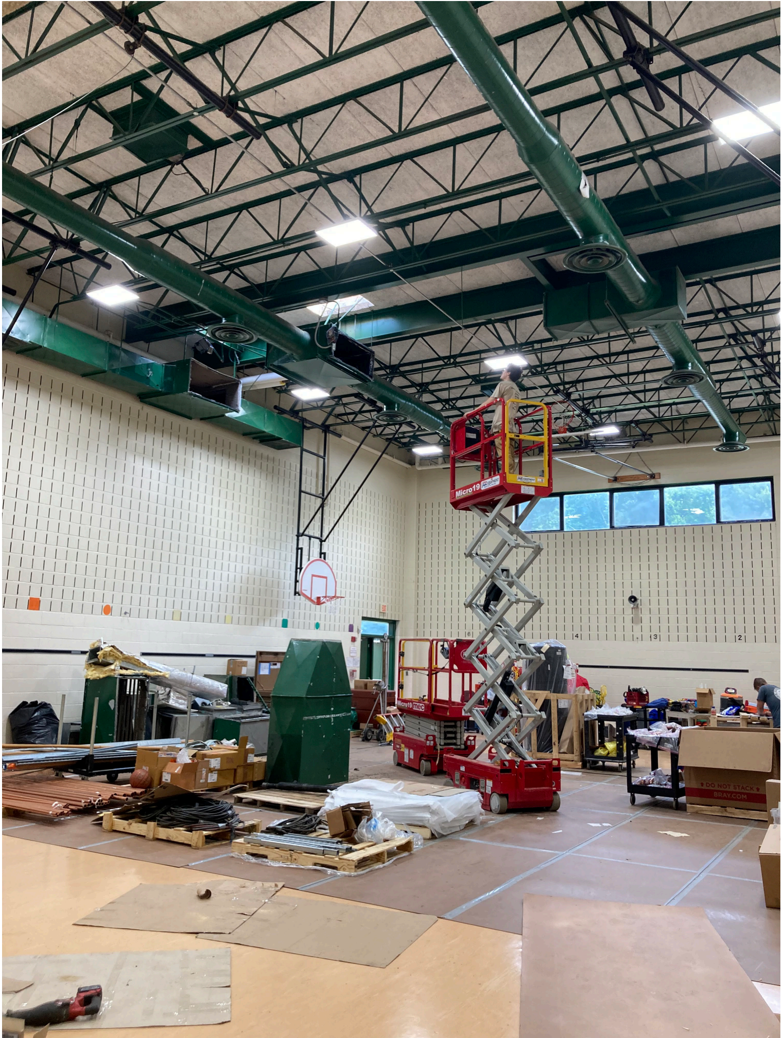
CECIL MANOR ELEMENTARY SCHOOL – HVAC REPLACEMENT
