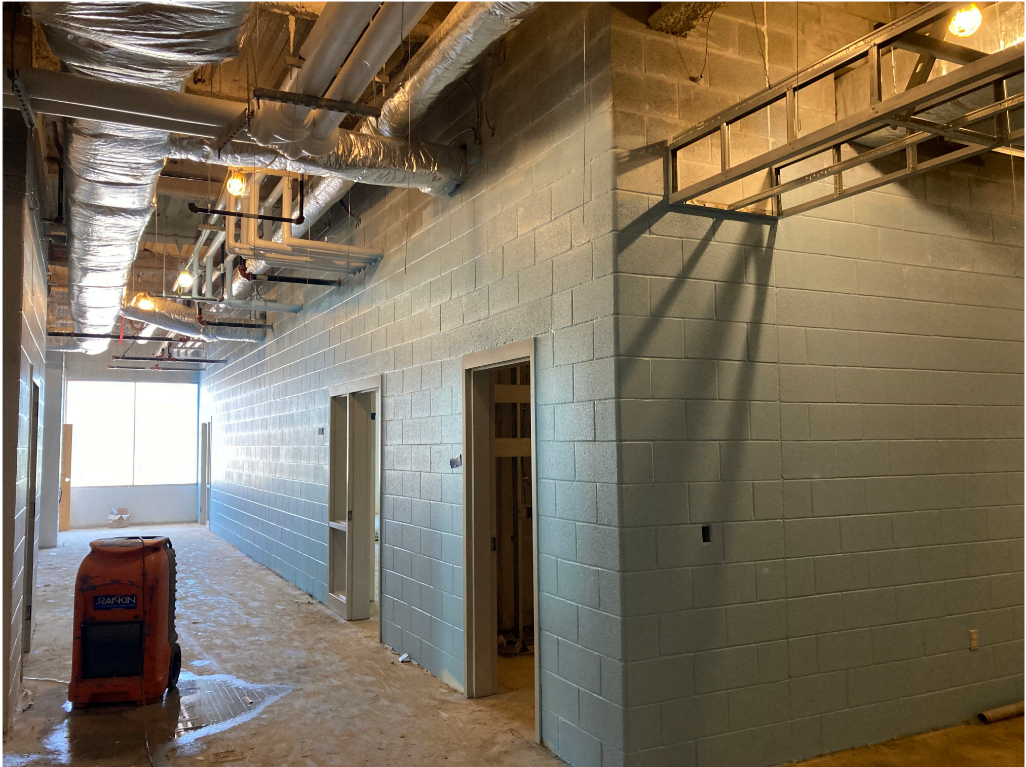
NORTH EAST MIDDLE / HIGH SCHOOL – REPLACEMENT – DRYWALL AND PAINTING CONTINUE THROUGHTOUT CLASSROOM HALLS
