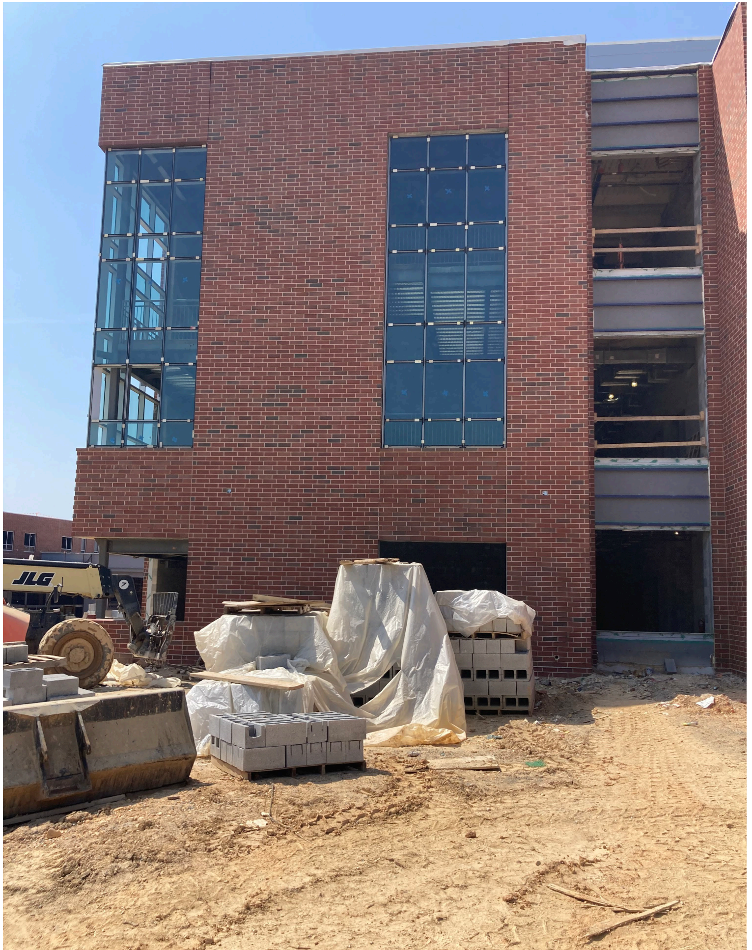
NORTH EAST MIDDLE / HIGH SCHOOL – REPLACEMENT – AREA G (HIGH SCHOOL) – WINDOW INSTALLATION
