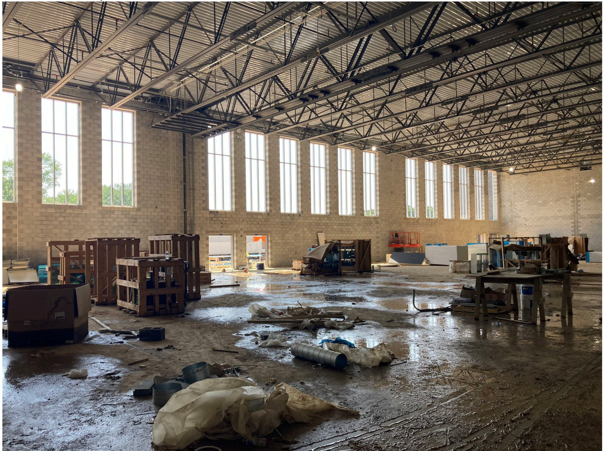
NORTH EAST MIDDLE / HIGH SCHOOL – REPLACEMENT – AREA A – GYMNASIUM INTERIOR – WINDOWS INSTALLED
