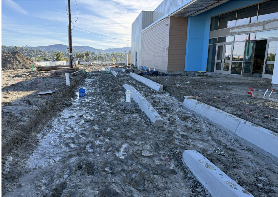
Upper Parking Lot Curb Install
