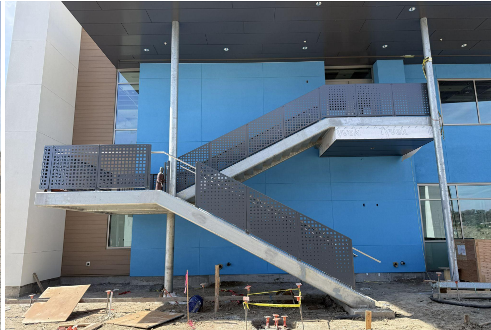
Bldg A Exterior Stair Handrail and Panel Installation
