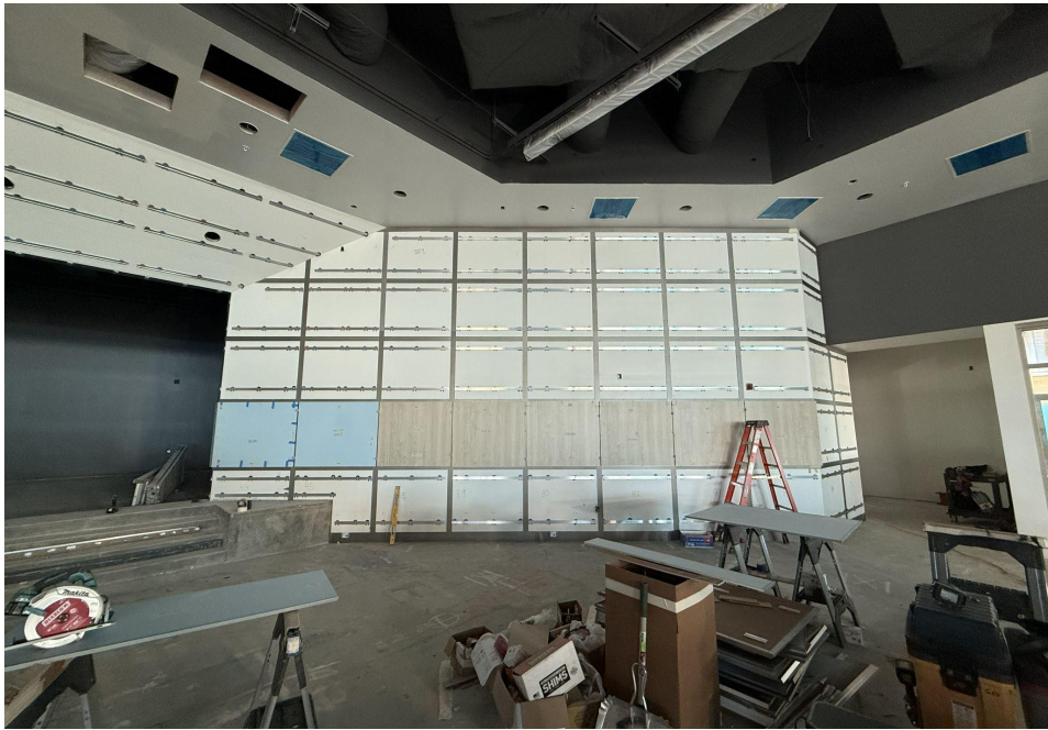
Bldg B MPR Door Wall Panel Installation
