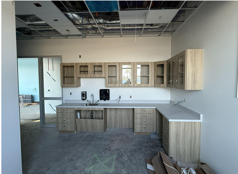
Bldg A Health Office Casework Installation
