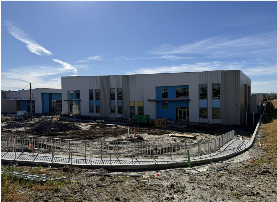
Bldg A View From Bobier Dr.
