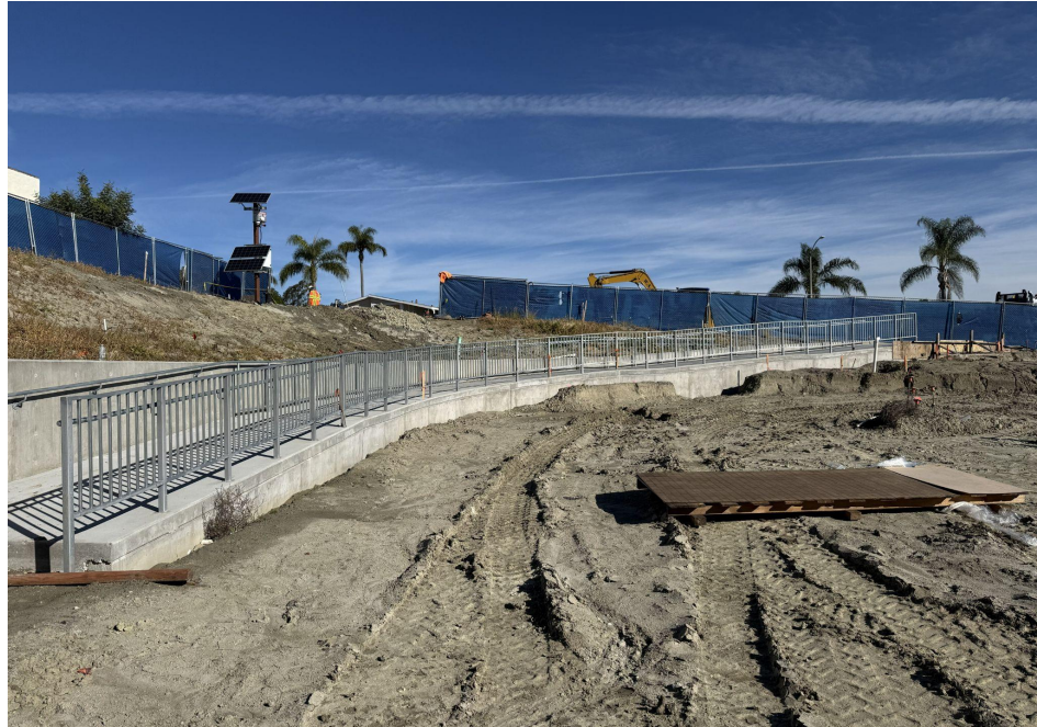
Upper Parking Lot Ramp Handrail Installation
