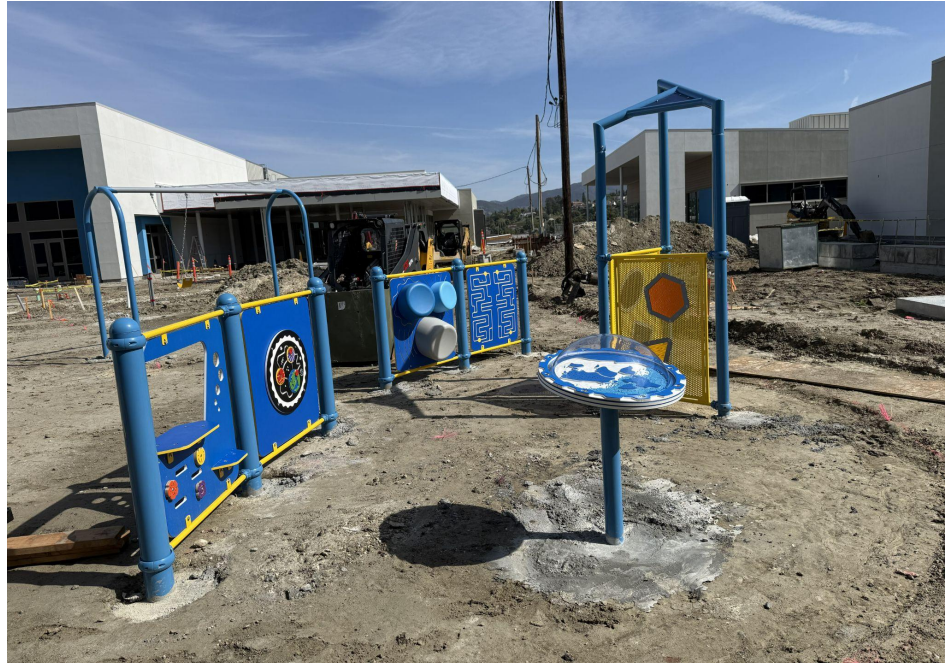
2 - 5 Age Group Play Ground Equipment Installation
