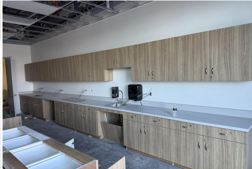
Bldg A Staff Workroom Casework Installation
