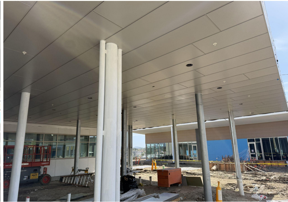
Bldg B Outdoor Lunch Area Canopy Installation
