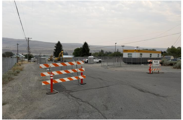
Construction access and staging
