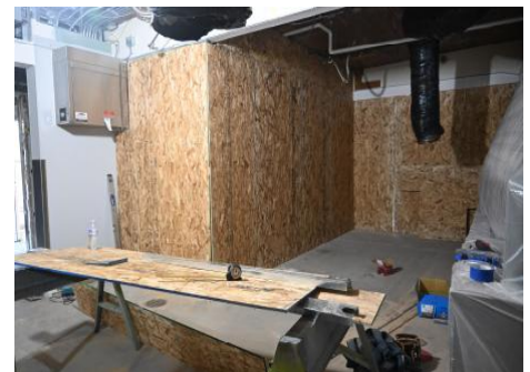
Selective Demolition in Progress
