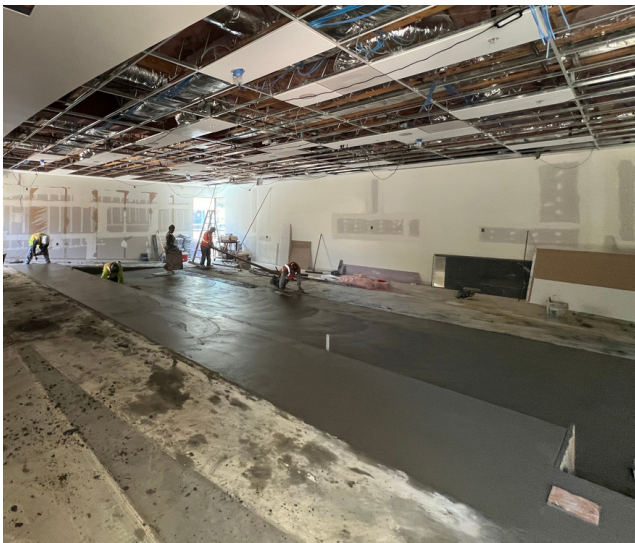
Pictured above : Concrete Placement in the new Makerspace
