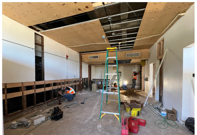
Pictured above : Framing work in the new Culinary Arts Room
