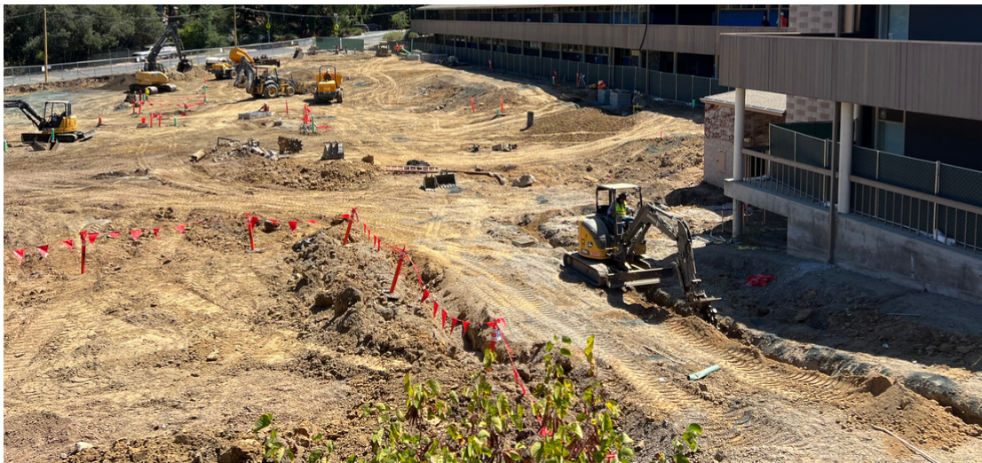
Pictured above : Site Preparation and Underground Utility Work
