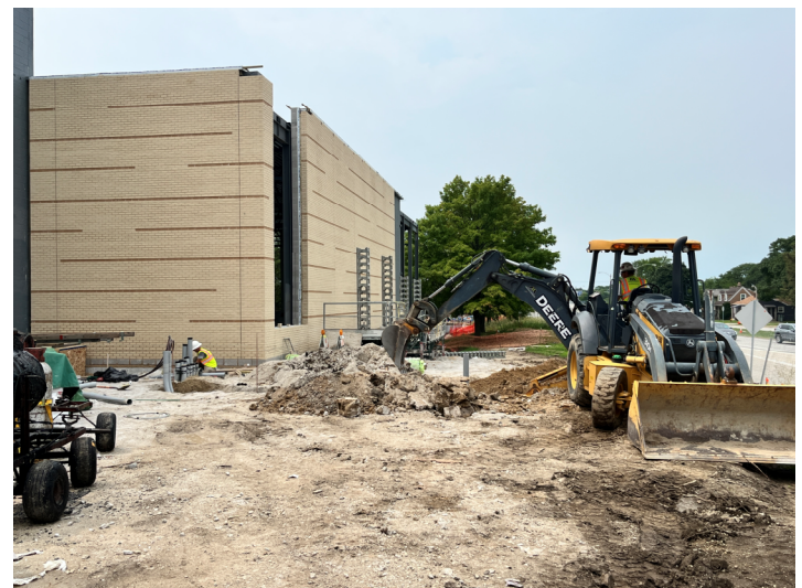
Excavating For Transformer – Northside Of Site
