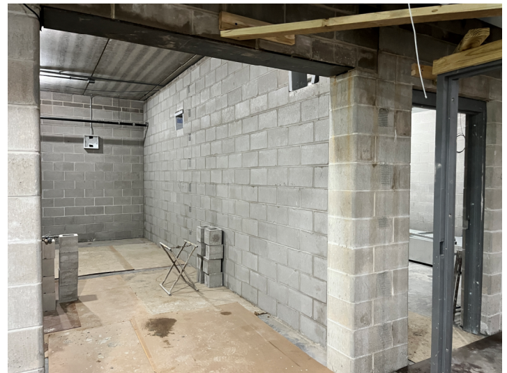
CMU Partition Built – Area B1 Ground Level Chem Storage Room
