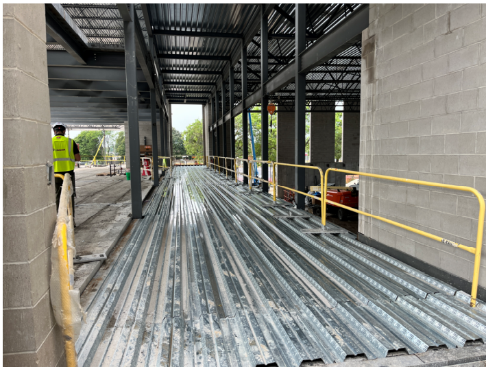
Floor Decking Installed – Area C1 1 st Level Corridor
