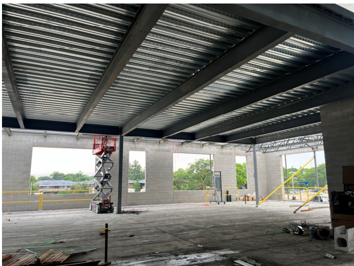
Floor Decking Installed – Area C1 2 nd Level Mechanical Room
