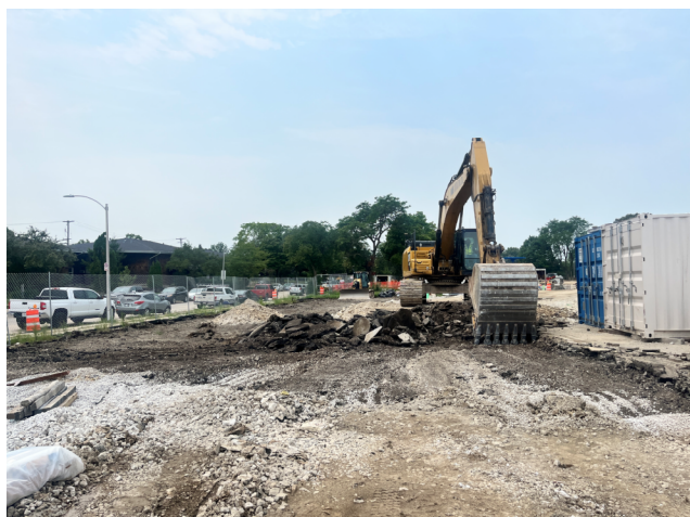
Grading – Southside Of Site
