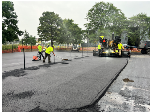
Sports Courts Paved – Site
