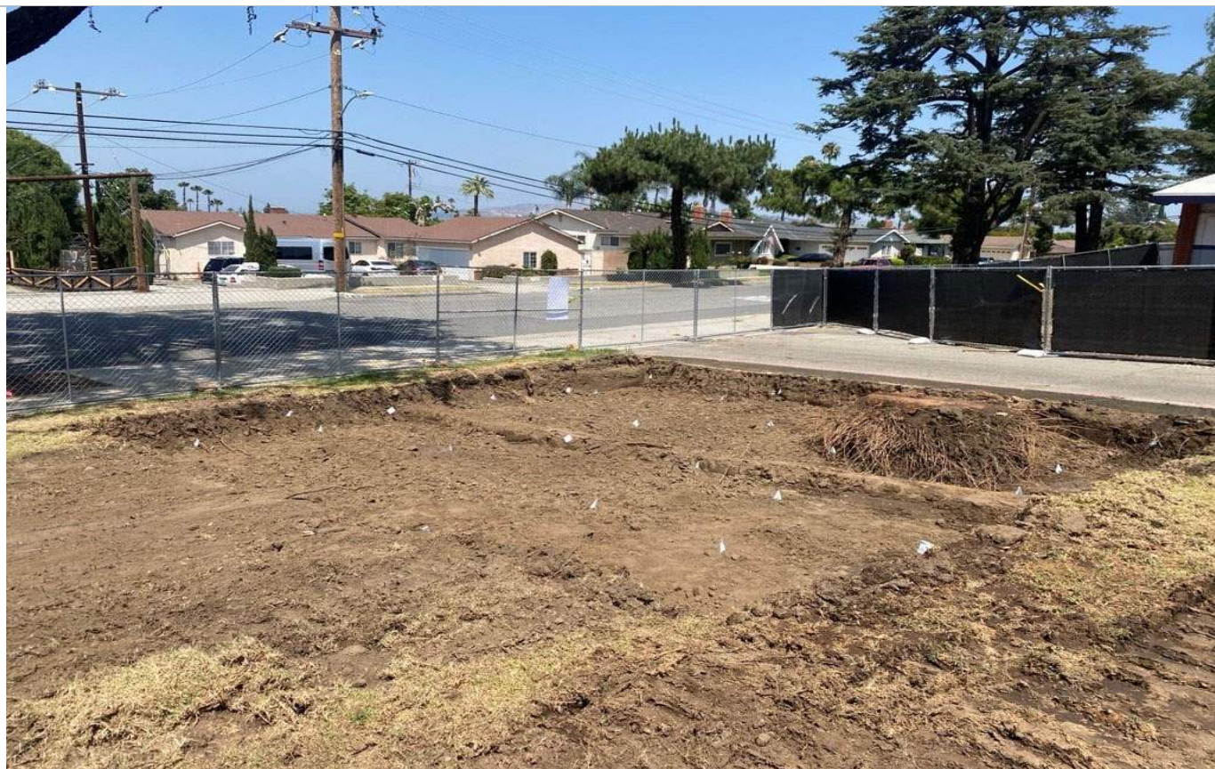
3: Zone 13.4 following excavation to 2 feet. XRF sample locations are shown.
