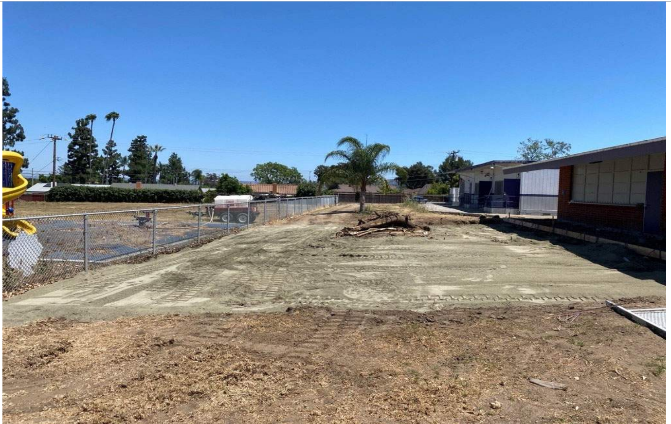
15: Zone 9 after backfill placement.
