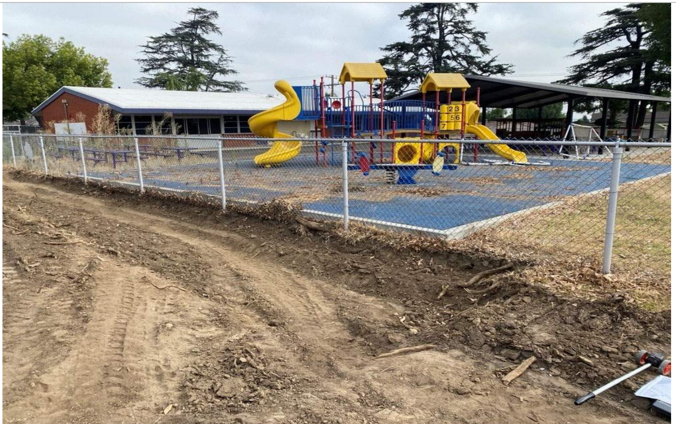
10: Zone 9 following 0.5-foot scrape down to 1.5 feet bgs.
