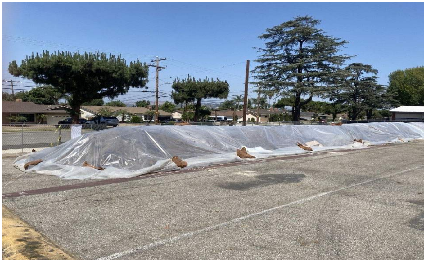
4: Stockpile #1 after Day 2 of excavation activities.
