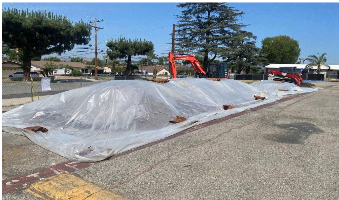
2: Stockpile #1 at the end of Day 1.
