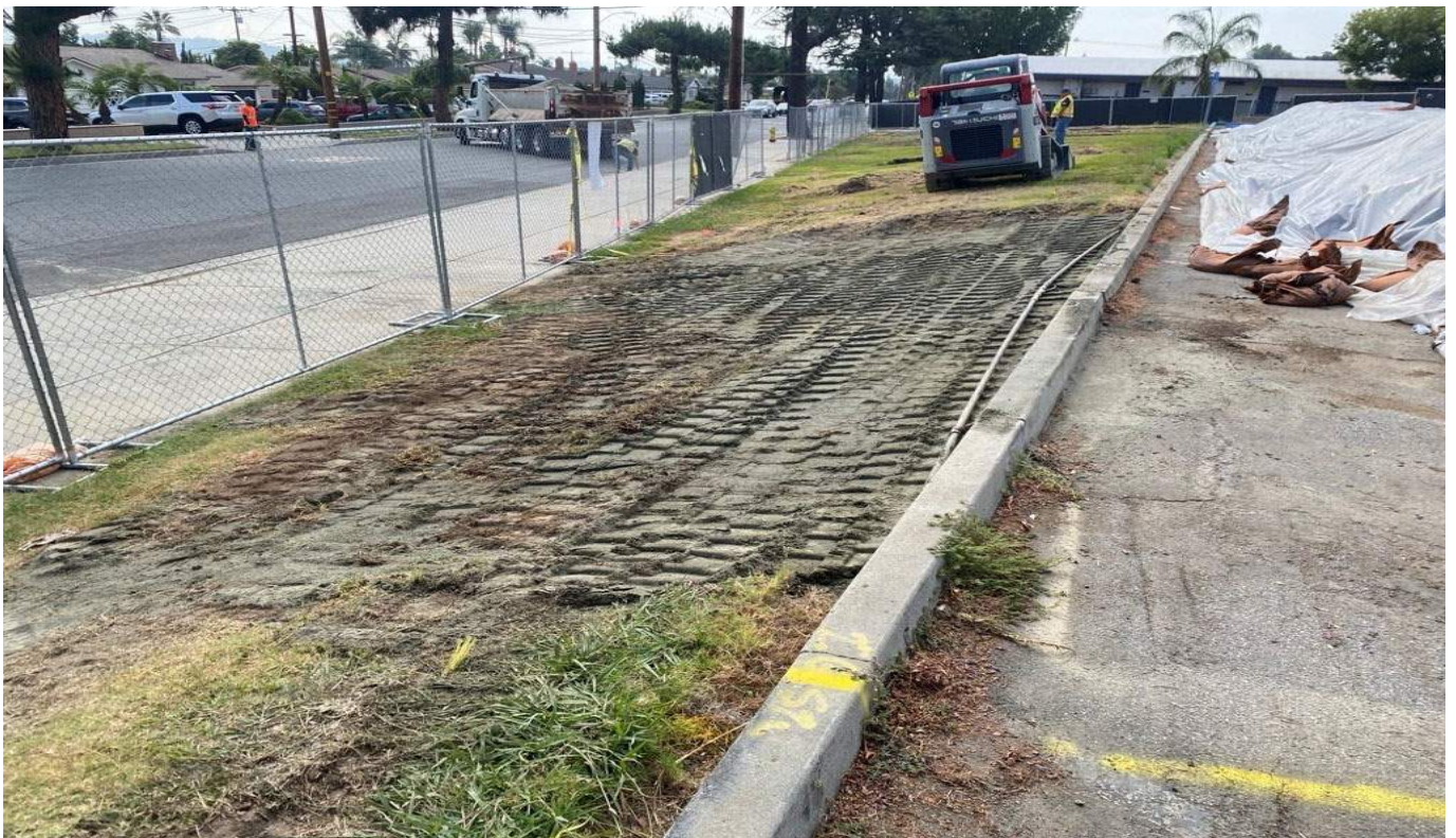
12: Zone 13.1 after backfill placement.
