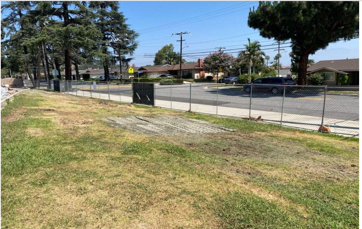
14: Zone 13.3 after backfill placement.
