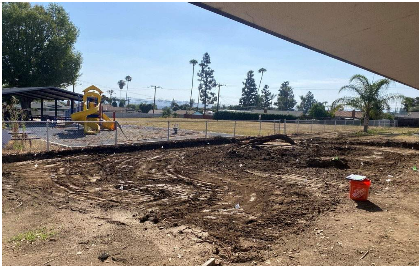
7: Zone 9 following 1-foot excavation.
