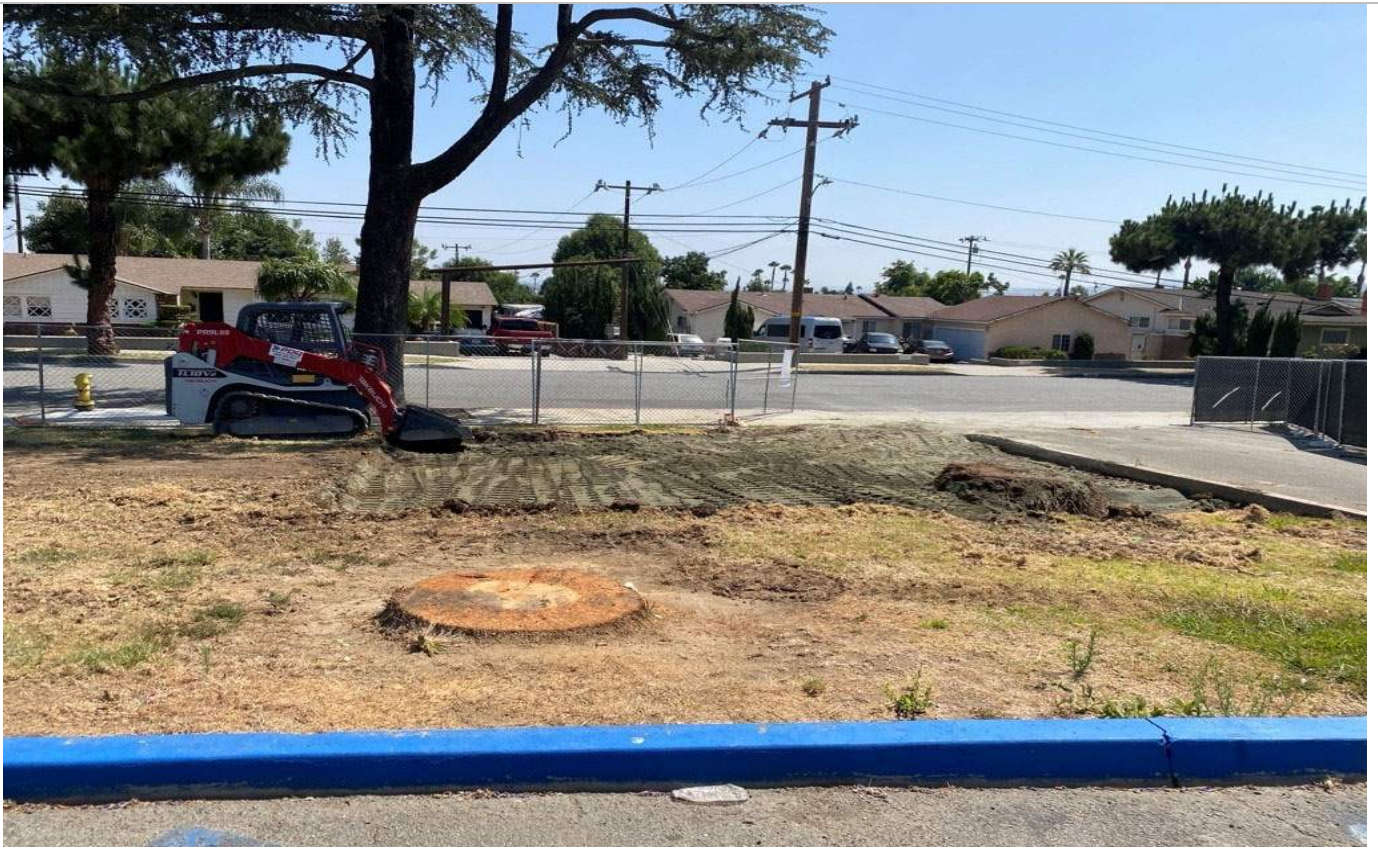
13: Zone 13.4 after backfill placement.
