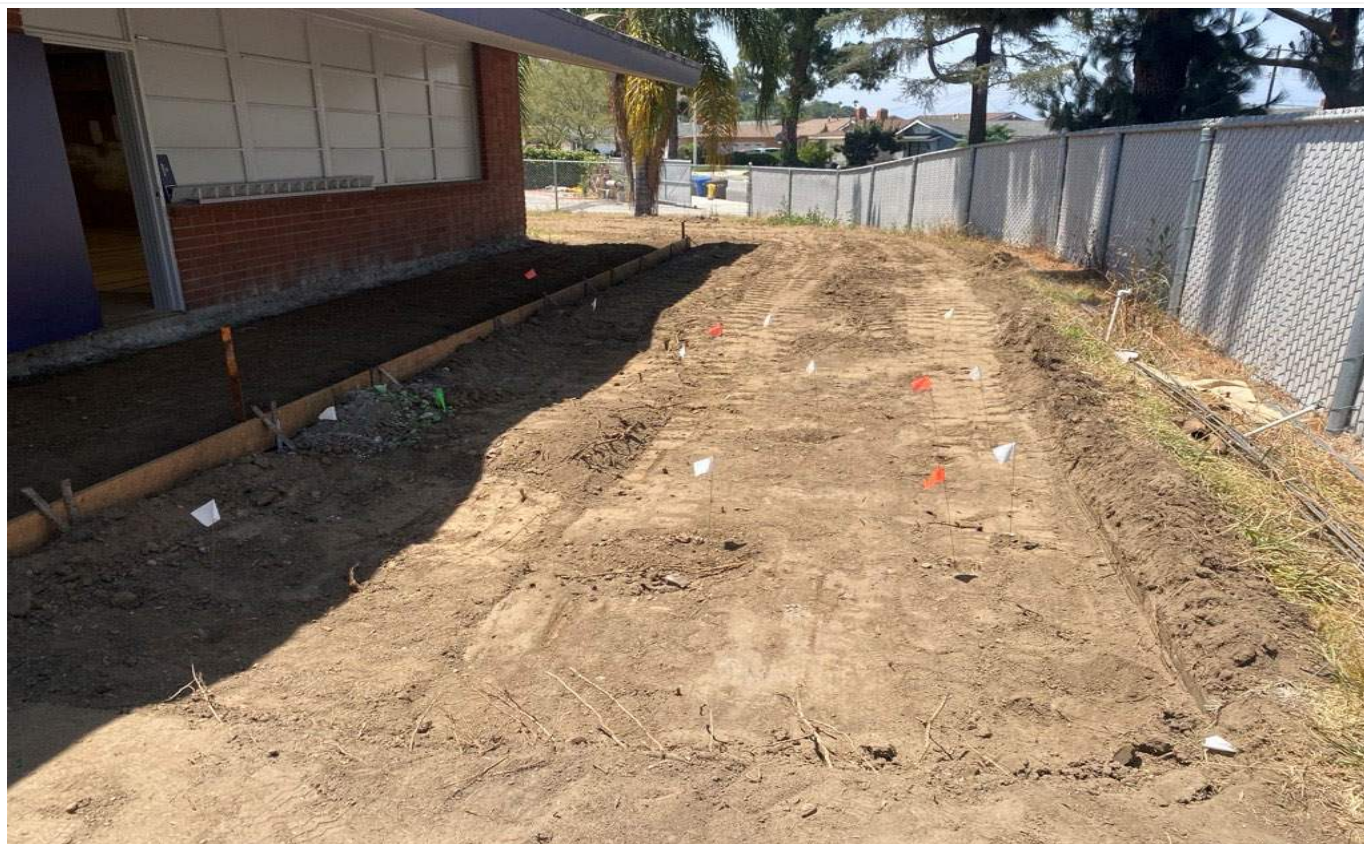
1: Zone 1 following 0.5-foot excavation. White flags indicate XRF sample locations; orange flags indicate confirmation sample locations.
