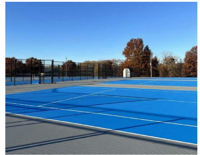
North Courts Looking Southwest
