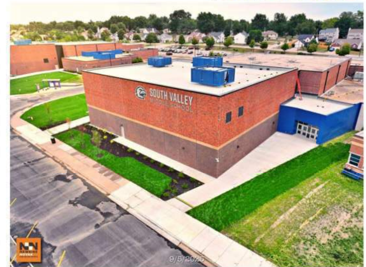
SVMS Exterior View
