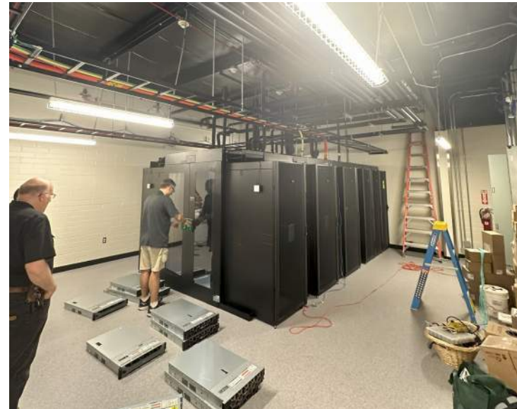
Data Pod Install
