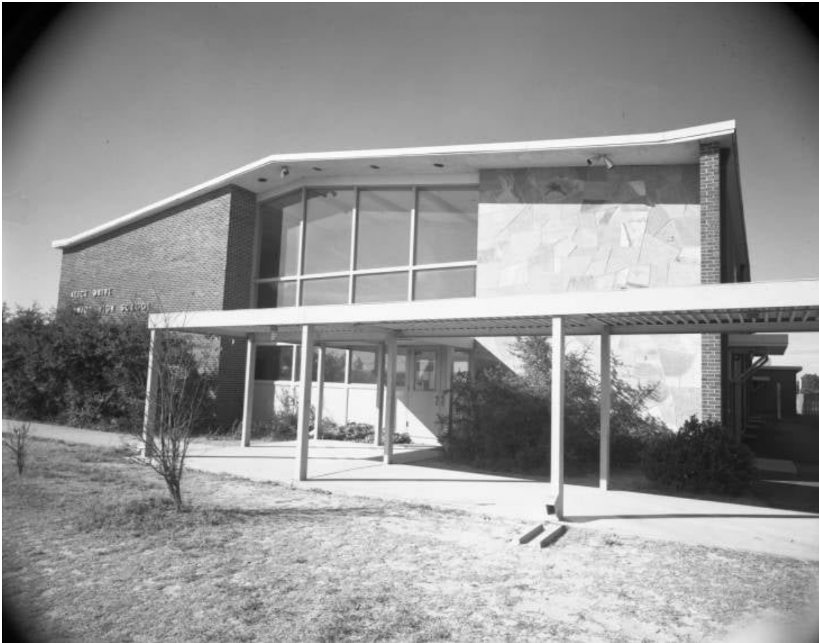
Figure 10: Alice Drive Junior High School in its original mid-century modern form, with the distinctive butterfly roofline, stone-and-glass entrance, and covered walkways characteristic of the schools built during South Carolina’s 1950s equalization campaign. Students gather outside the main entrance. Courtesy of local archival collections.
