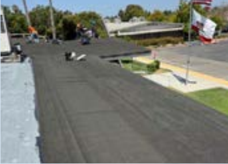
Adolfo Camarillo High School Roofing
