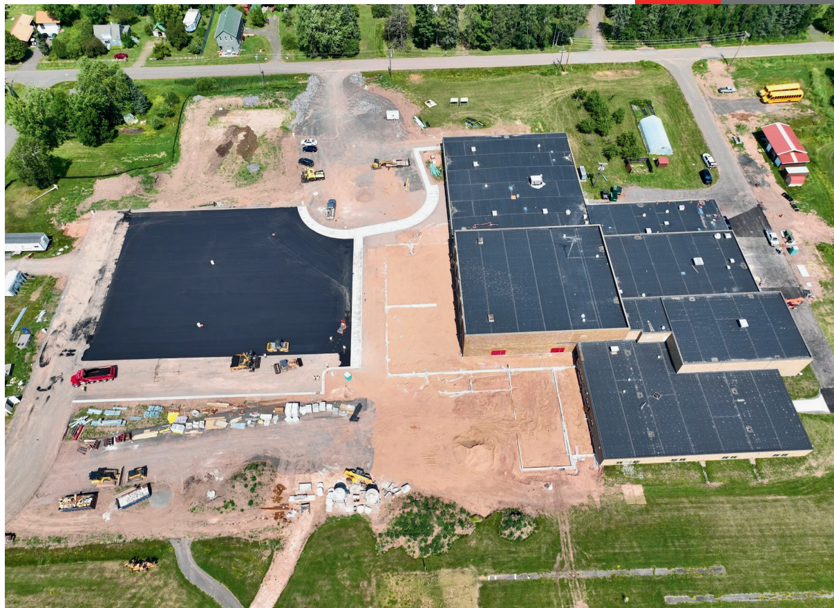
From above, you can see new asphalt in the parking lot and the new front sidewalk. The thin outline of the building addition is visible where the concrete footings rise just above the ground.
