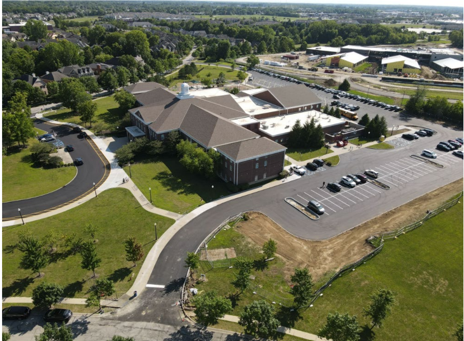
STONEGATE ASPHALT & CONCRETE REPLACEMENT
