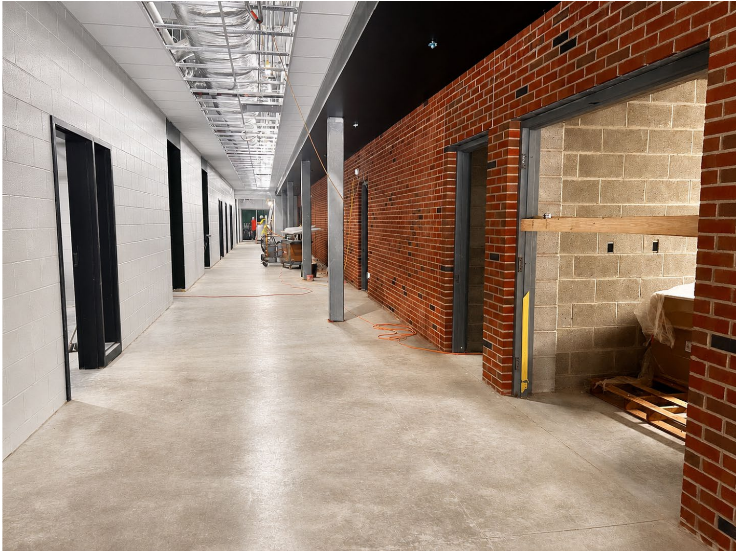
1ST FLOOR CORRIDOR
