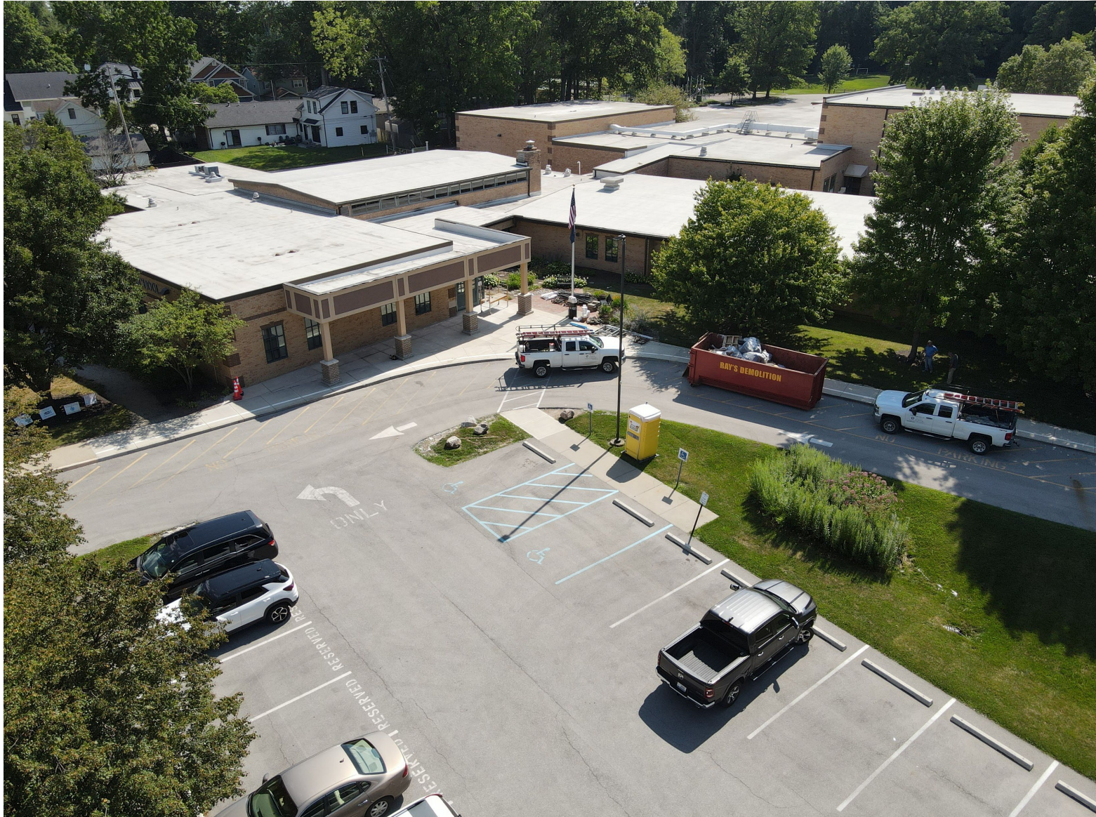
EAGLE ENTRANCE RENOVATION (8/1/26)
