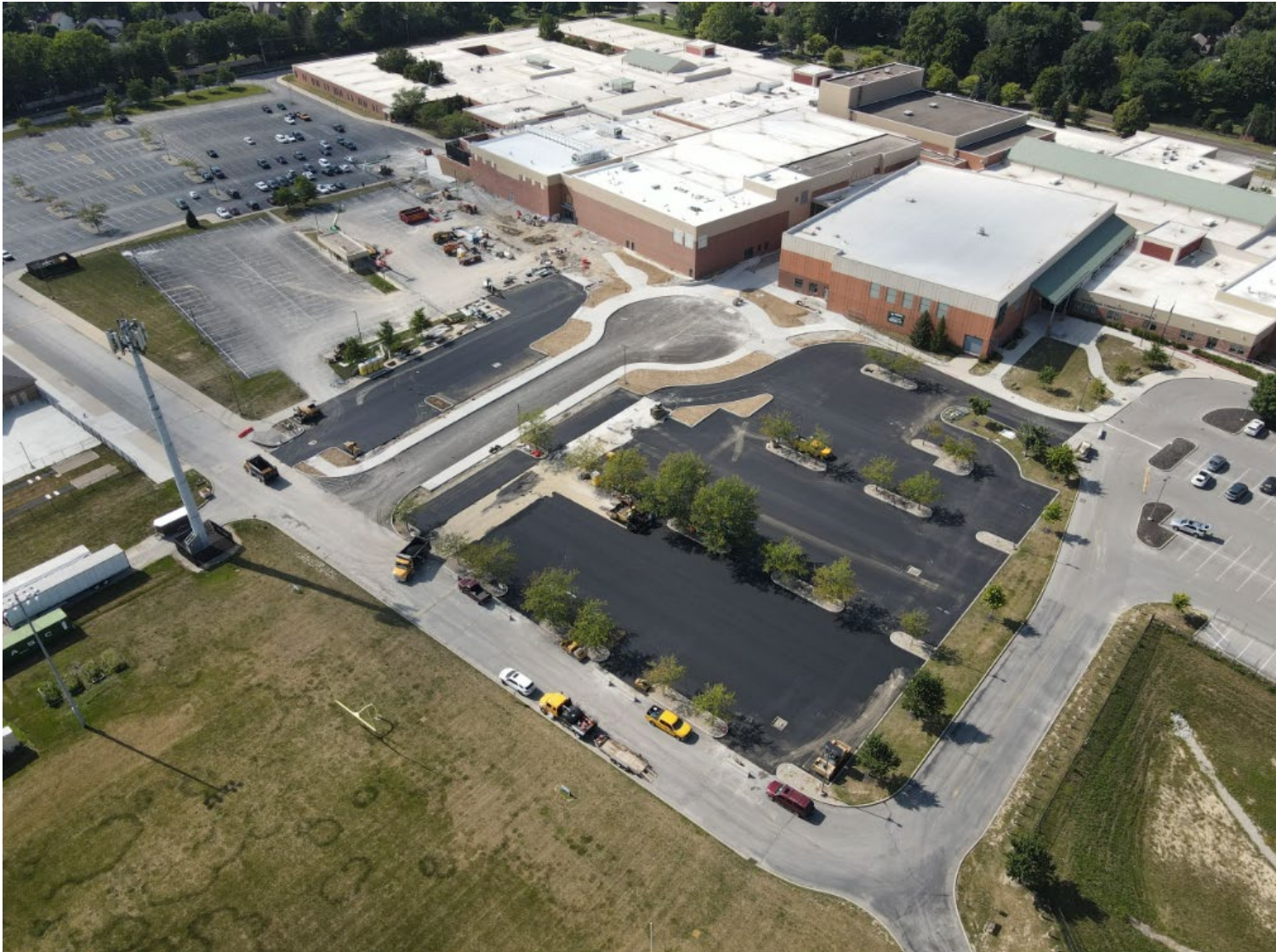
PARKING LOTS , DRIVES, & SIDEWALKS (8/1/26)
