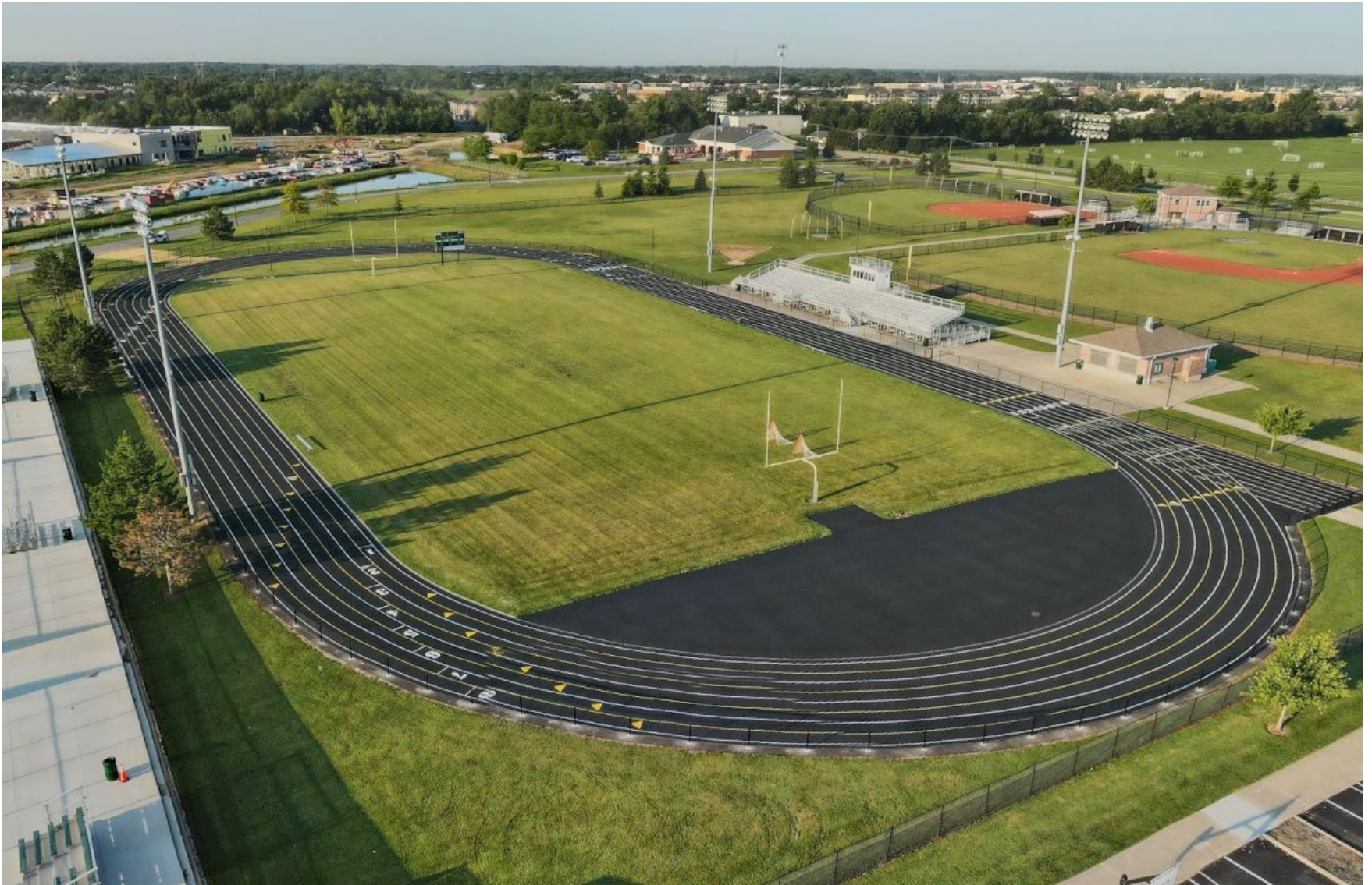
ZWMS TRACK SURFACE & FENCE REPLACEMENT
