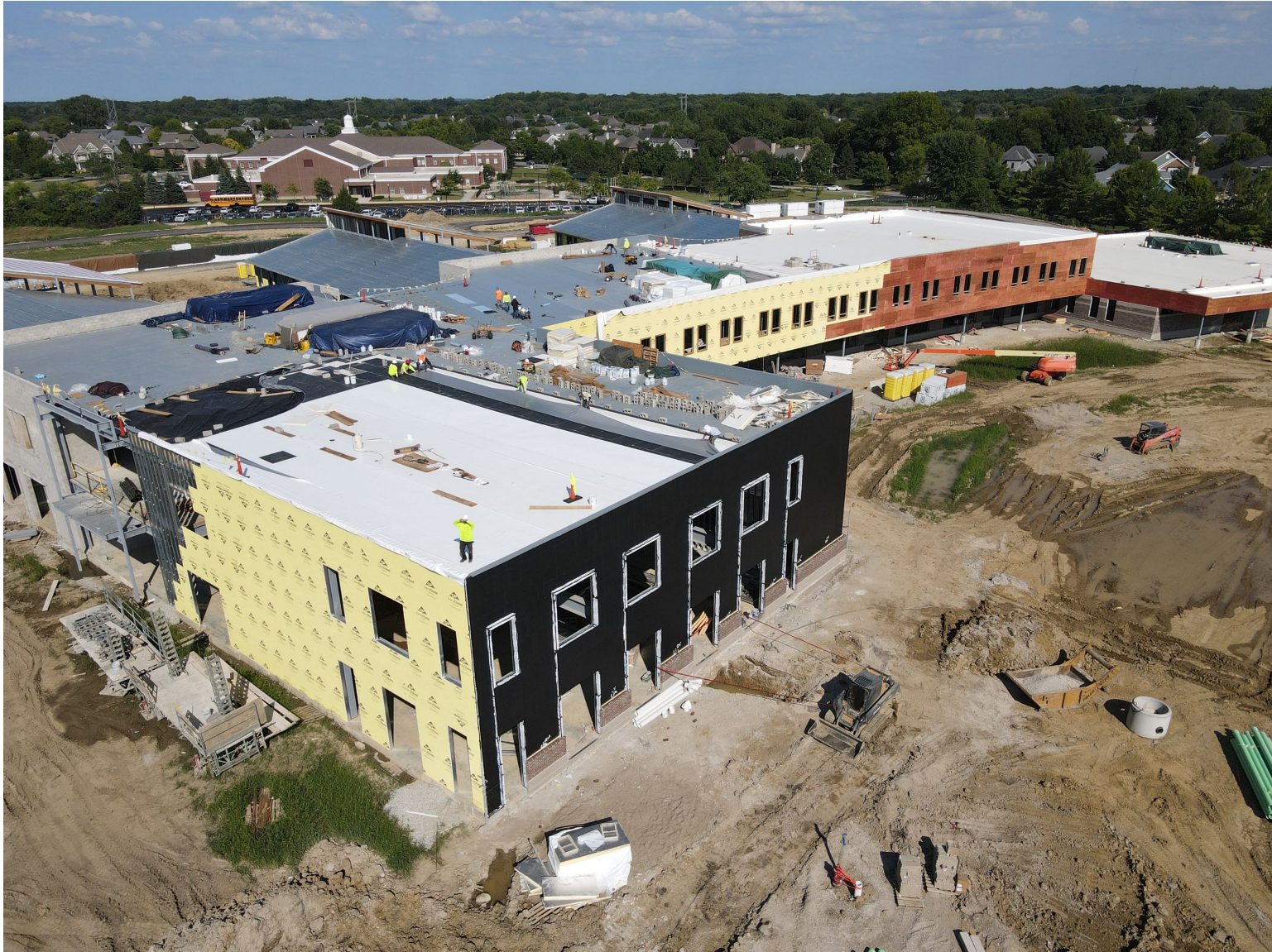
NORTHWEST 2-STORY WING - MAIN ESC ENTRY / BOARD ROOM (8-1-26)
