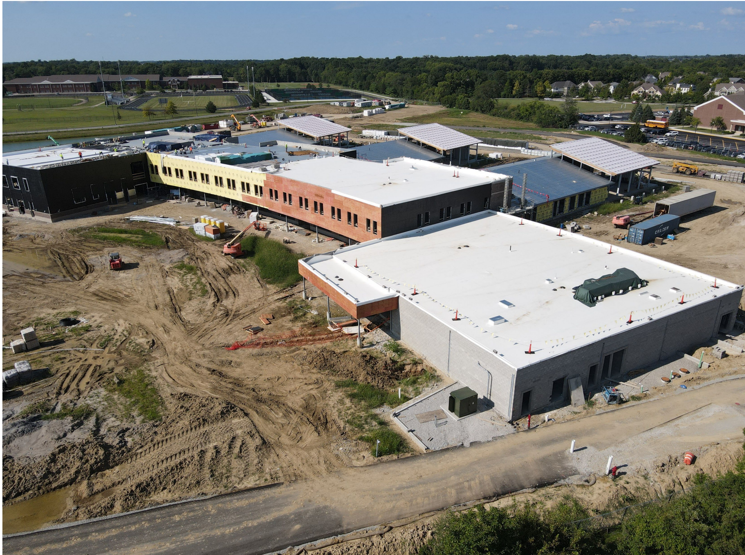
SOUTHWEST 1-STORY WING - ELC MAIN ENTRANCE / BUILDING SERVICES (8-1-26)
