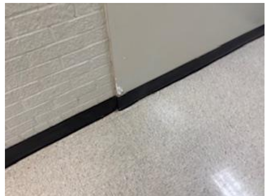
#34 View of PC-19 Light Grey Paint on Brick Wall
