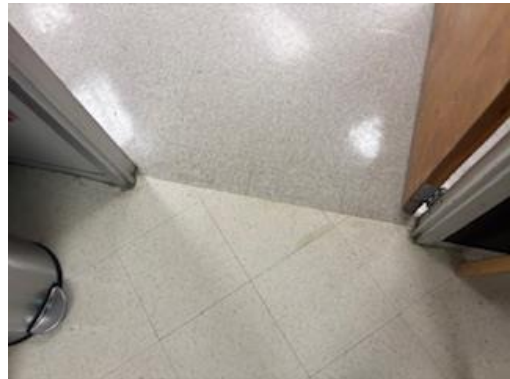
#14 View of HA-26: 12"x12" White with Light Grey Speck Vinyl Floor Tile and associated Mastic
