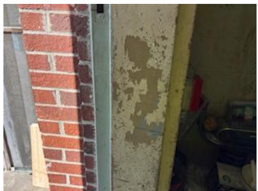
#36 View of PC-24 Tan Paint on Metal Door Frame
