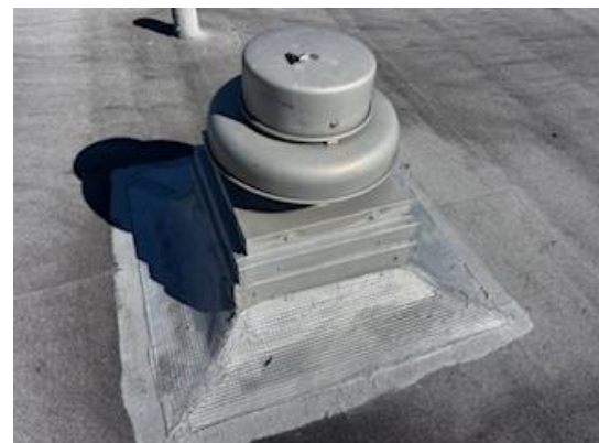
#6 View of HA-08: Grey Exhaust Hood Sealant
