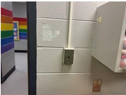
#29 View of PC-12 Light Grey Paint on CMU Walls
