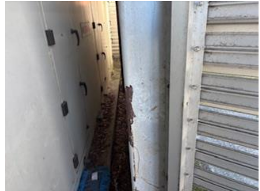
#26 View of PC-01 Grey/Silver Paint on Metal Gate
