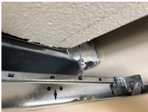
#23 View of HA-52 2' x 2' Ceiling Tile and HA-55 White HVAC Duct Seam Mastic and PC-22 White Paint on Gypsum Walls
