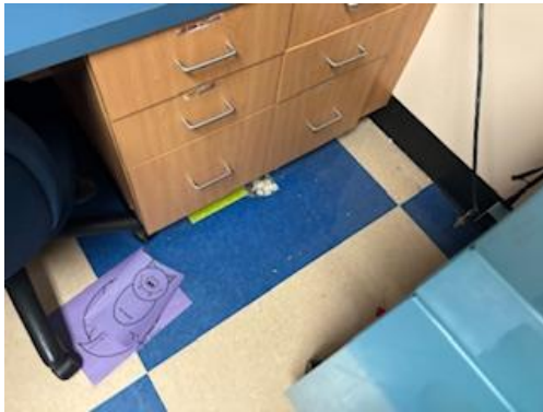
#25 View of HA-56, HA-58, HA-61 and HA-62 Annex Flooring Materials
