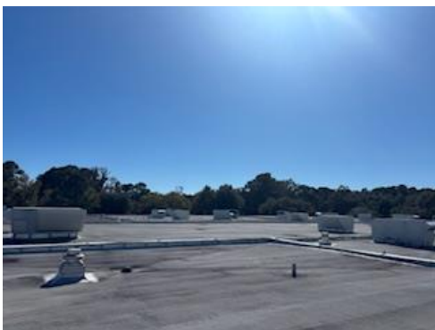
#5 View of HA-07: Main Building Roof
