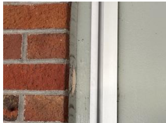
#8 View of HA-13: Grey Exterior Door Caulk and PC-06 Light Green Paint on Metal Door
