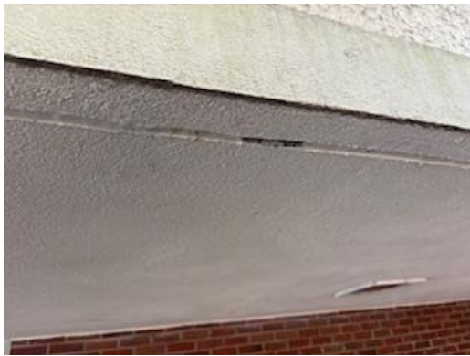
#7 View of HA-10: White Textured Soffit and HA-11: and associated Sealant
