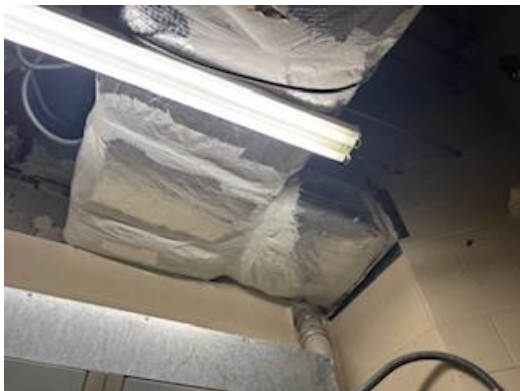
#17 View of HA-33: White HVAC Duct Seam Mastic
