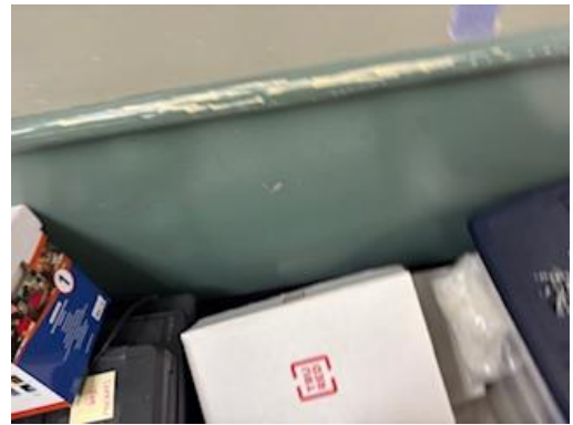
#32 View of PC-17 Green Paint on Wood Chair Rail
