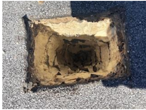
#2 View of HA-02: Annex Roof Core
