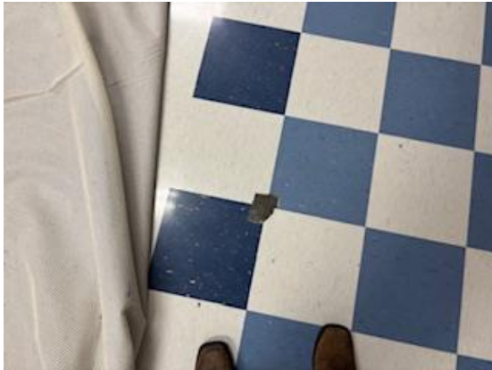
#19 View of HA-40, HA-41, and HA-42: Vinyl Floor Tiles
