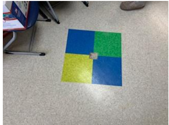
#22 View of HA-48, HA-49, and HA-50: Vinyl Floor Tiles
