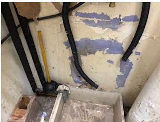
#33 View of PC-18 White Paint on Gypsum Wall
