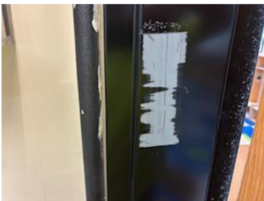
#35 View of PC-21 Black Paint on Metal Door Frame
