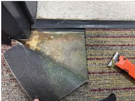
#15 View of HA-30: Green Carpet Mastic
