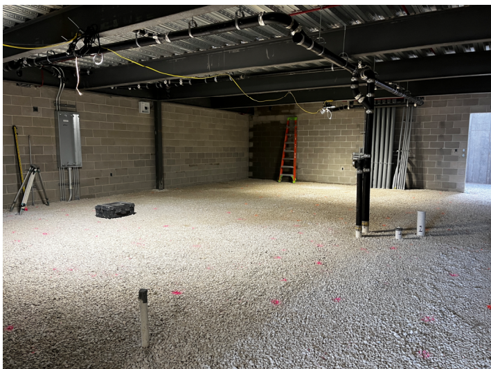
Gym Storage Fine Graded – Area A2 Ground Level
