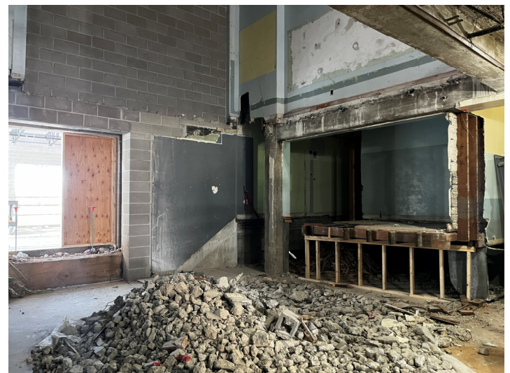
Demolition – Area A1 1 st Level Stair/Ramp
