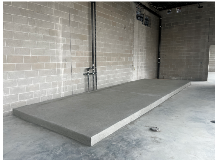
Concrete Housekeeping Pad Poured – Area B1 1 st Floor Mechanical Room
