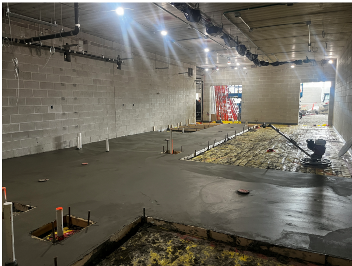
Concrete Poured – Area B1 Ground Level Locker Rooms
