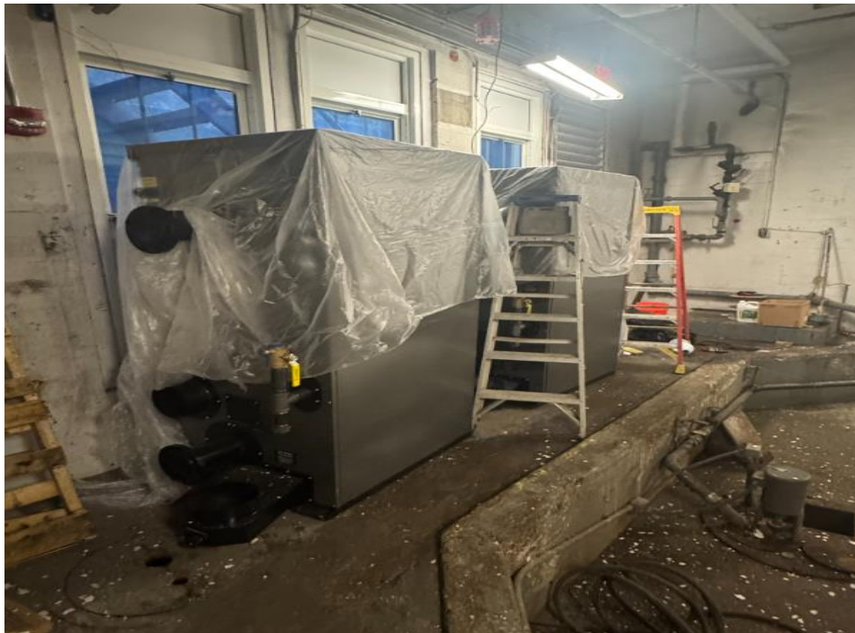
Hempstead Paterson – Boiler replacement
