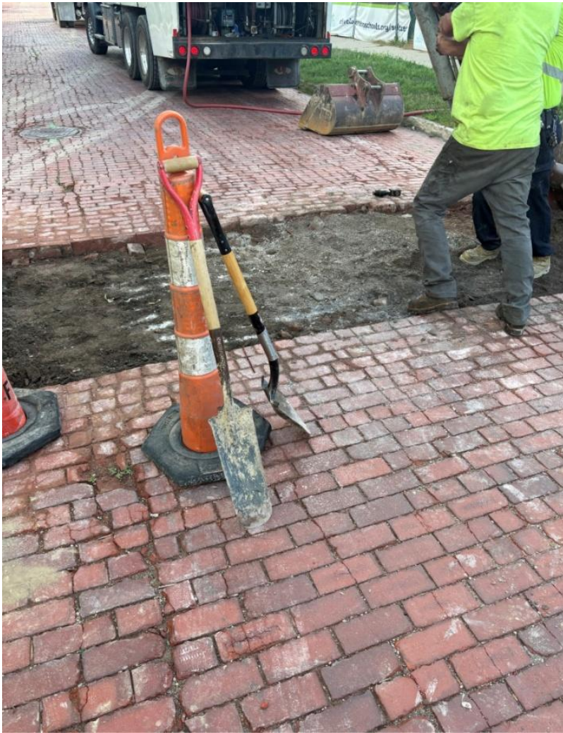
Prepare West 98 th St. for sewer tie-in
