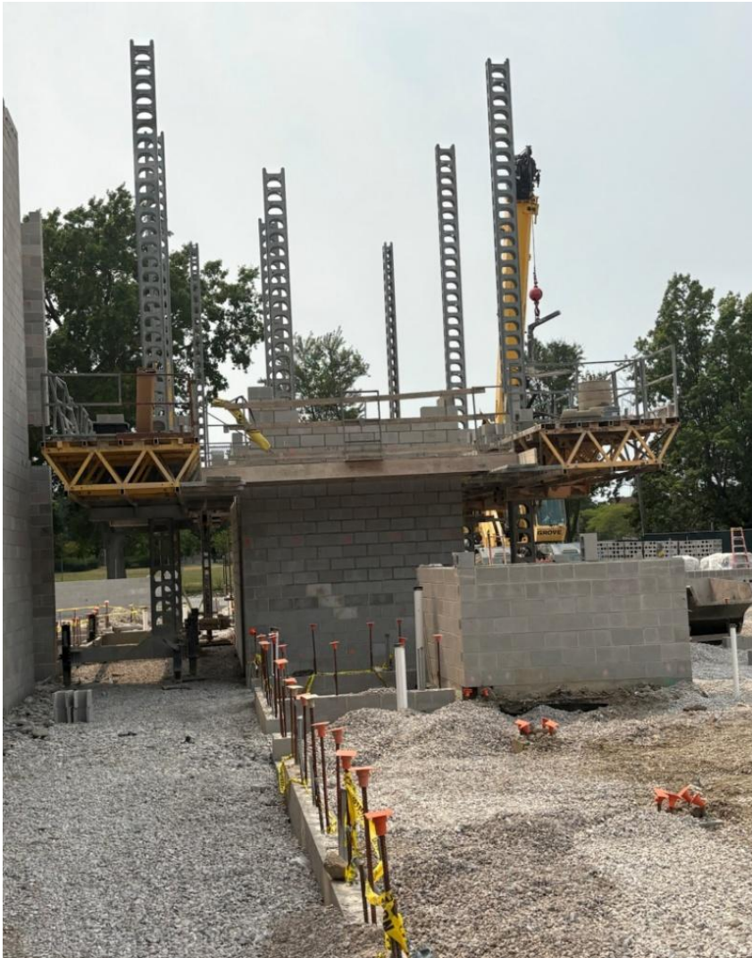
Stair No. 02 Masonry Walls
