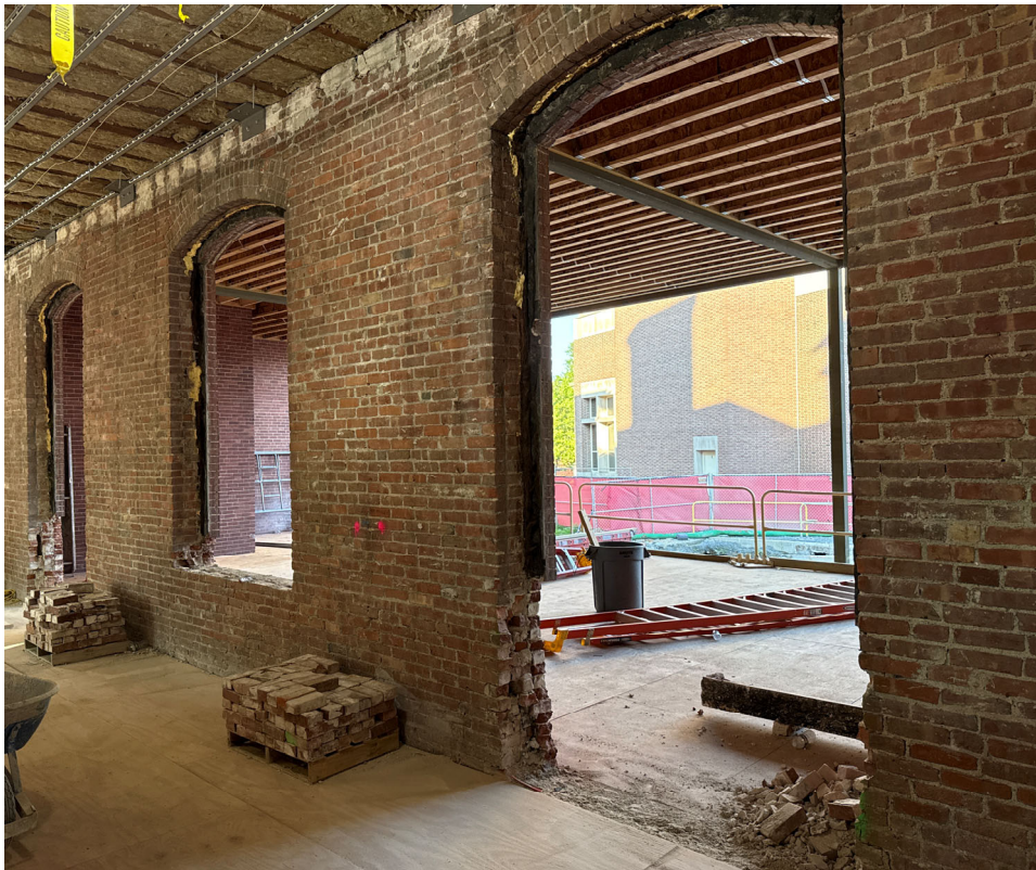
Brick Openings to Historic Building Addition
