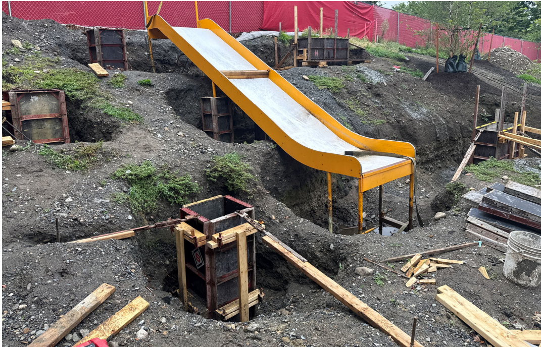
Footing Forms, Slide and Stone Scrambles in Pierce Park
