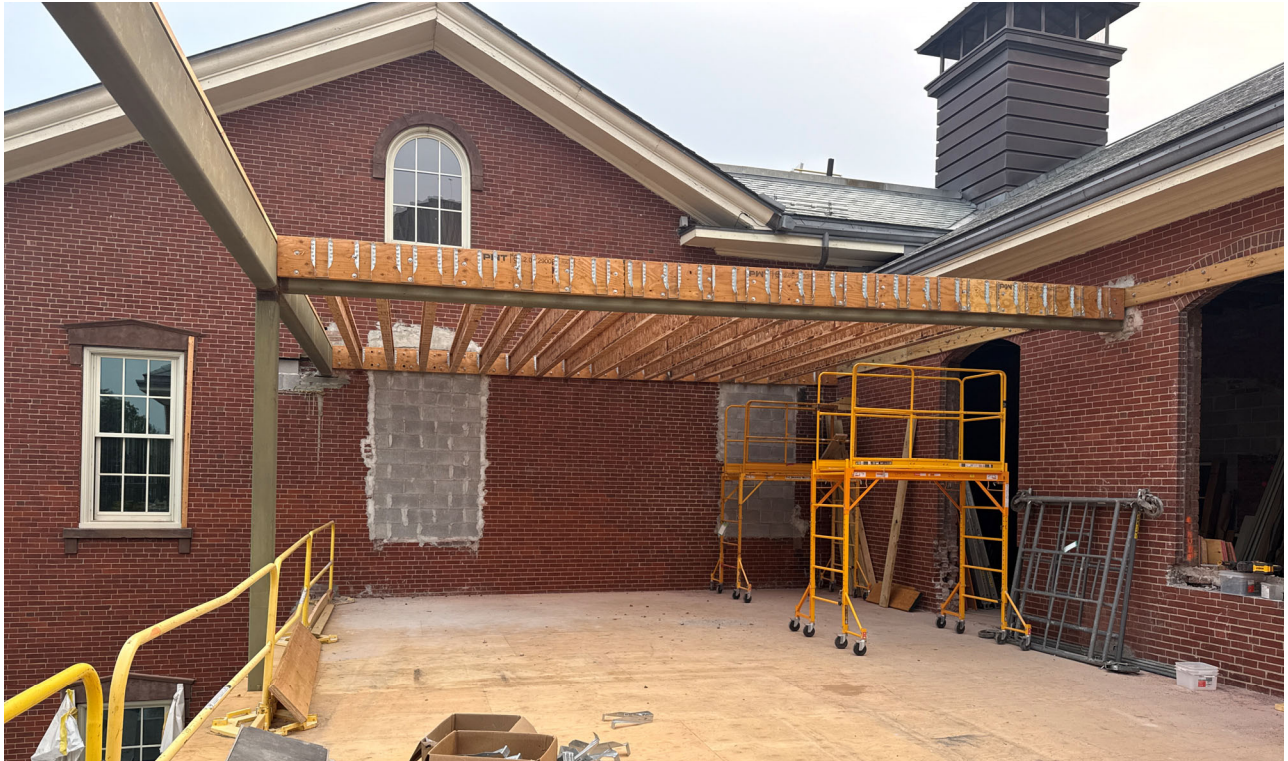
Framing of Addition to Historic Building
