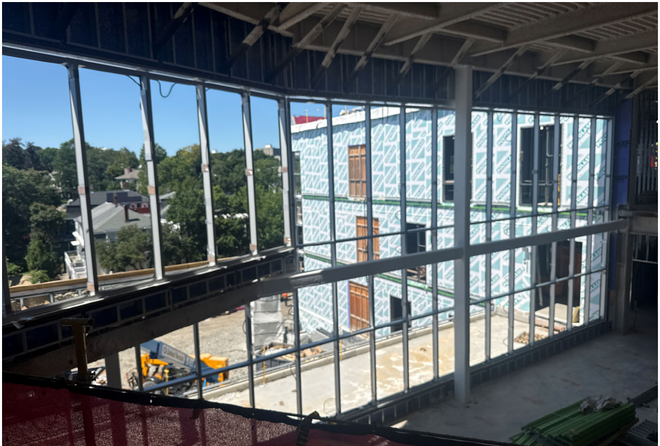
Curtainwall Installation, West Elevation at Library
