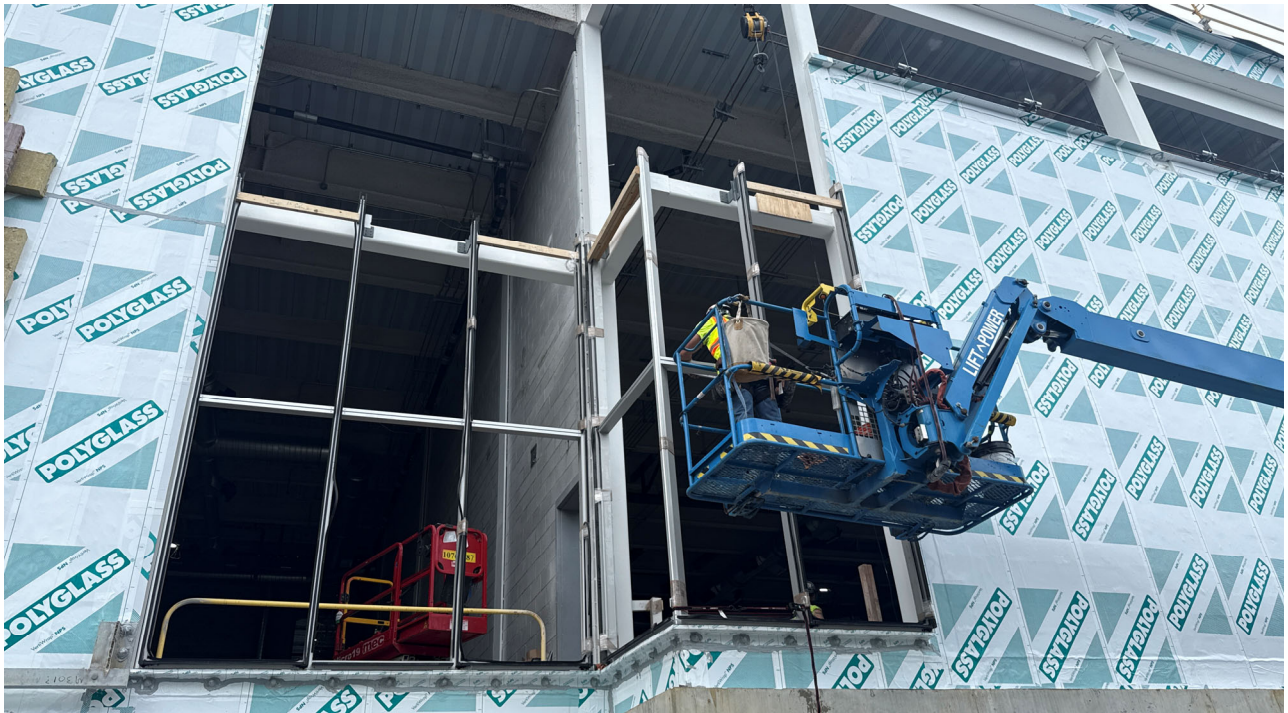
Curtainwall Installation, North elevation at Gyms
