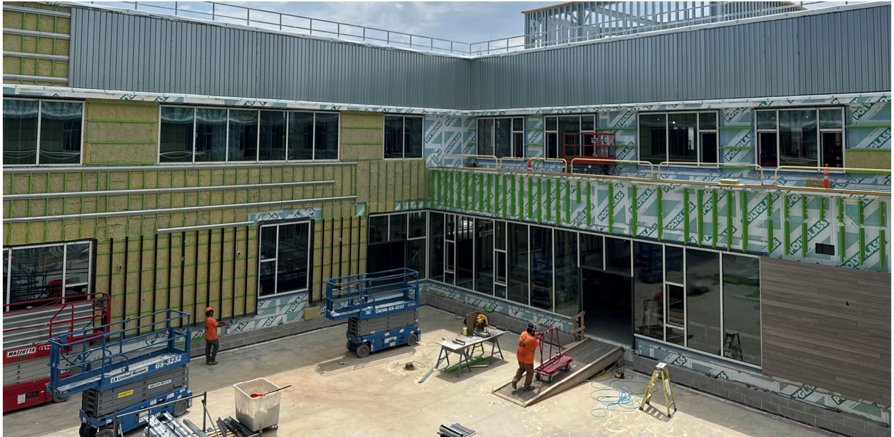
Zinc Panels Installation in Courtyard
