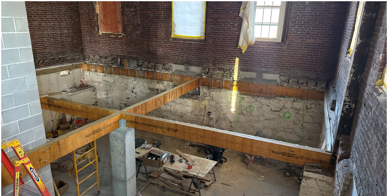
Wood Framing at Elevator Area
