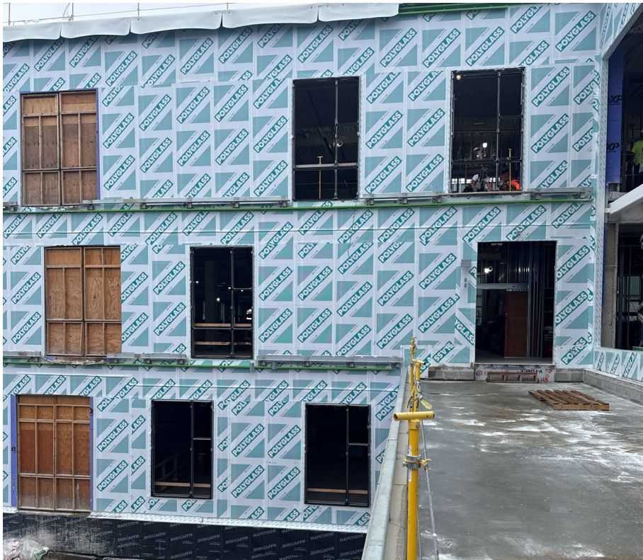
Window Frame Installation, Building A South Elevation
