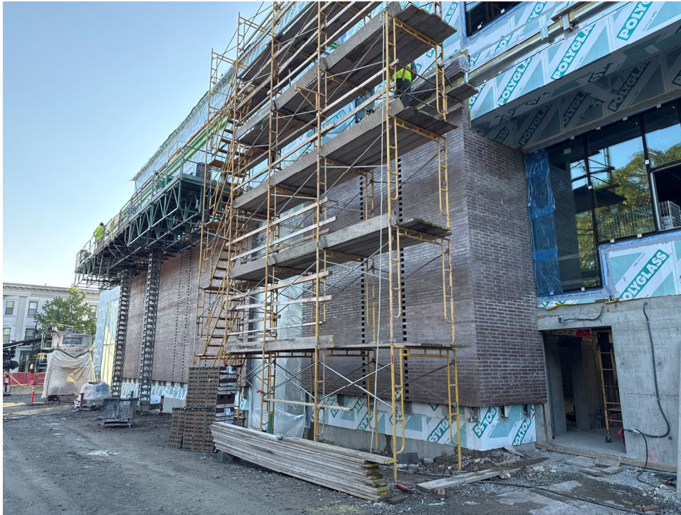
Brick Progress at West Elevation
