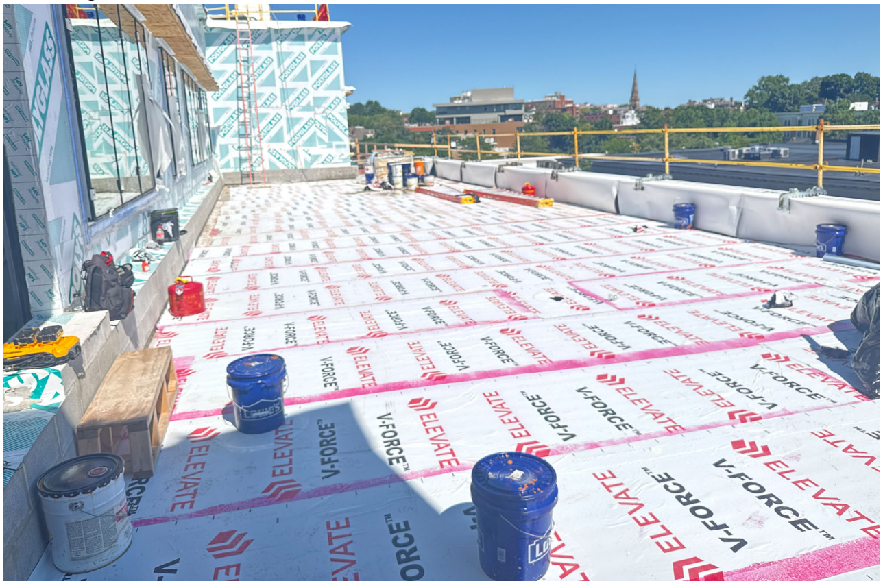
Low Roof and Walls at North Elevation
