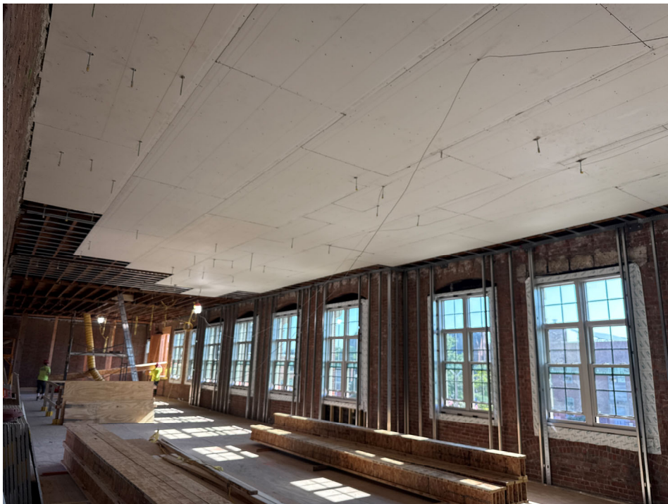
GWB Ceilings and Hangers on Level 1 in Historic Building
