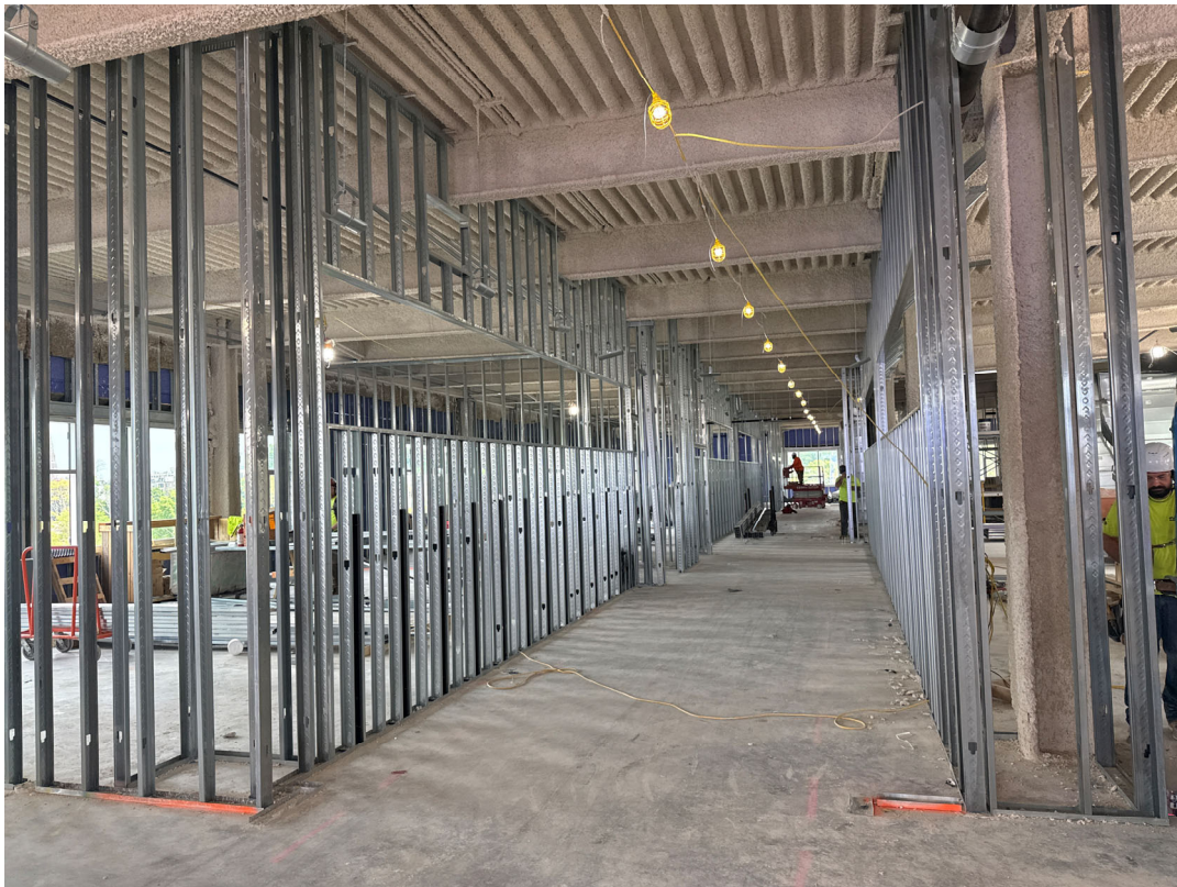
Interior Framing in A3 West
