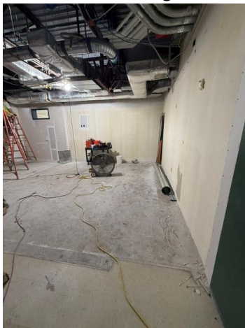
Sheetrock hung at breakfast area
