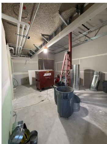
Sheetrock hung at kitchen
