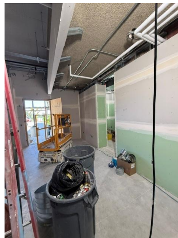
Sheetrock hung at kitchen
