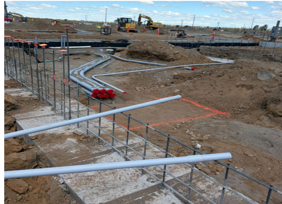
Underslab building electrical
