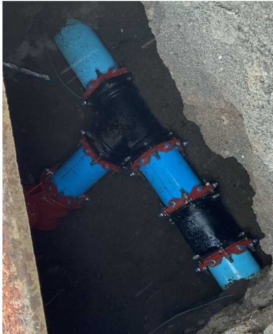
Watermain tie-in at 1 st Ave
