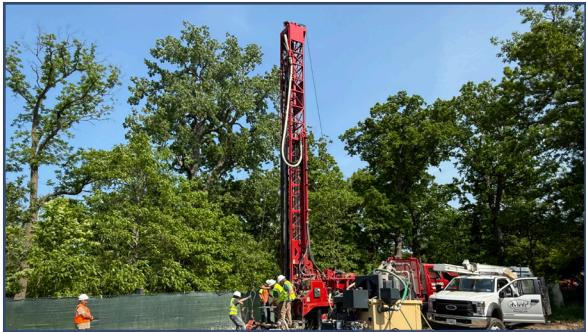
By drilling into the ground, the system uses stable underground conditions to efficiently heat and cool.
