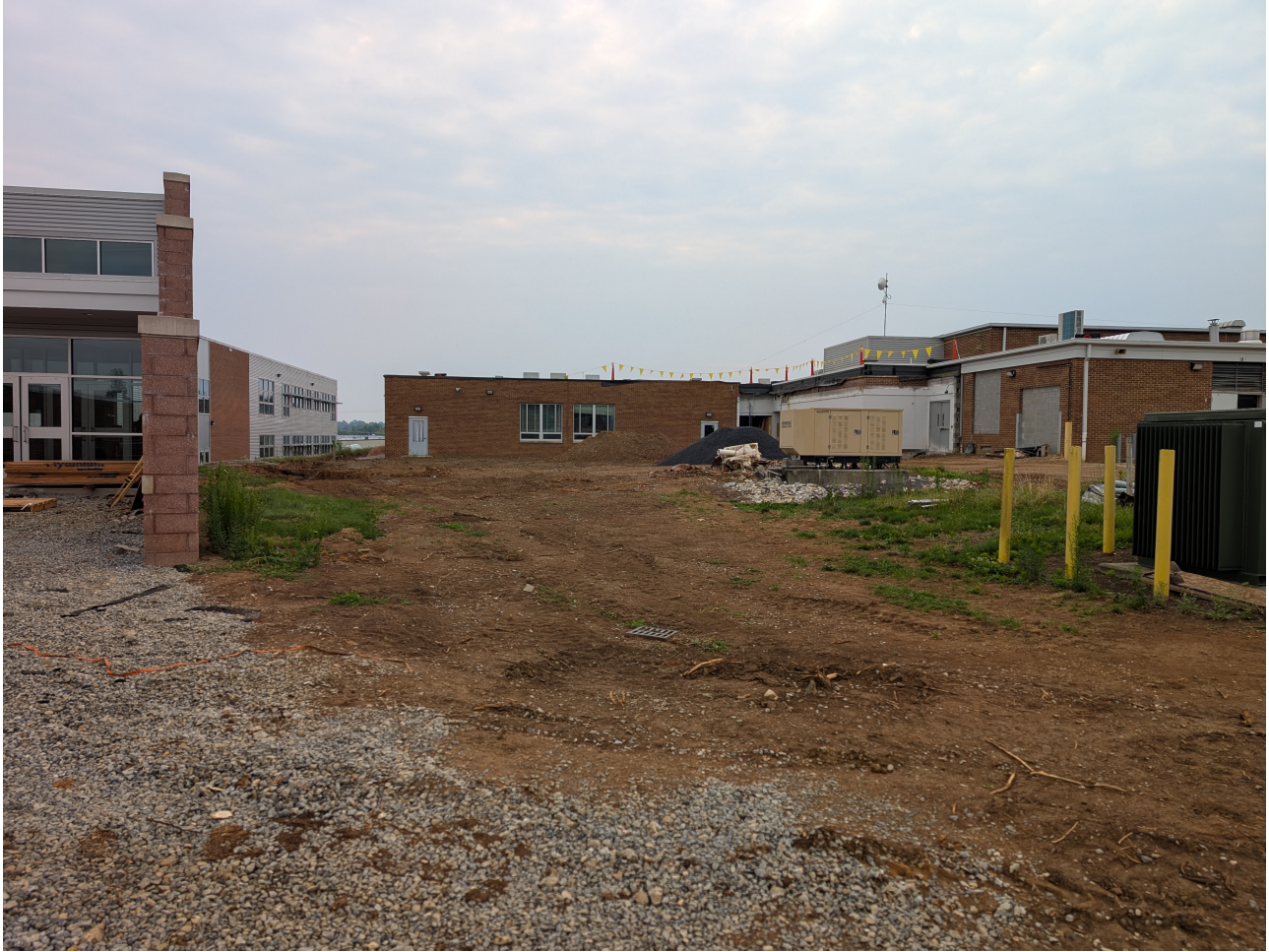
Hallway Demo Between Kindergarten Wing and Front of School
