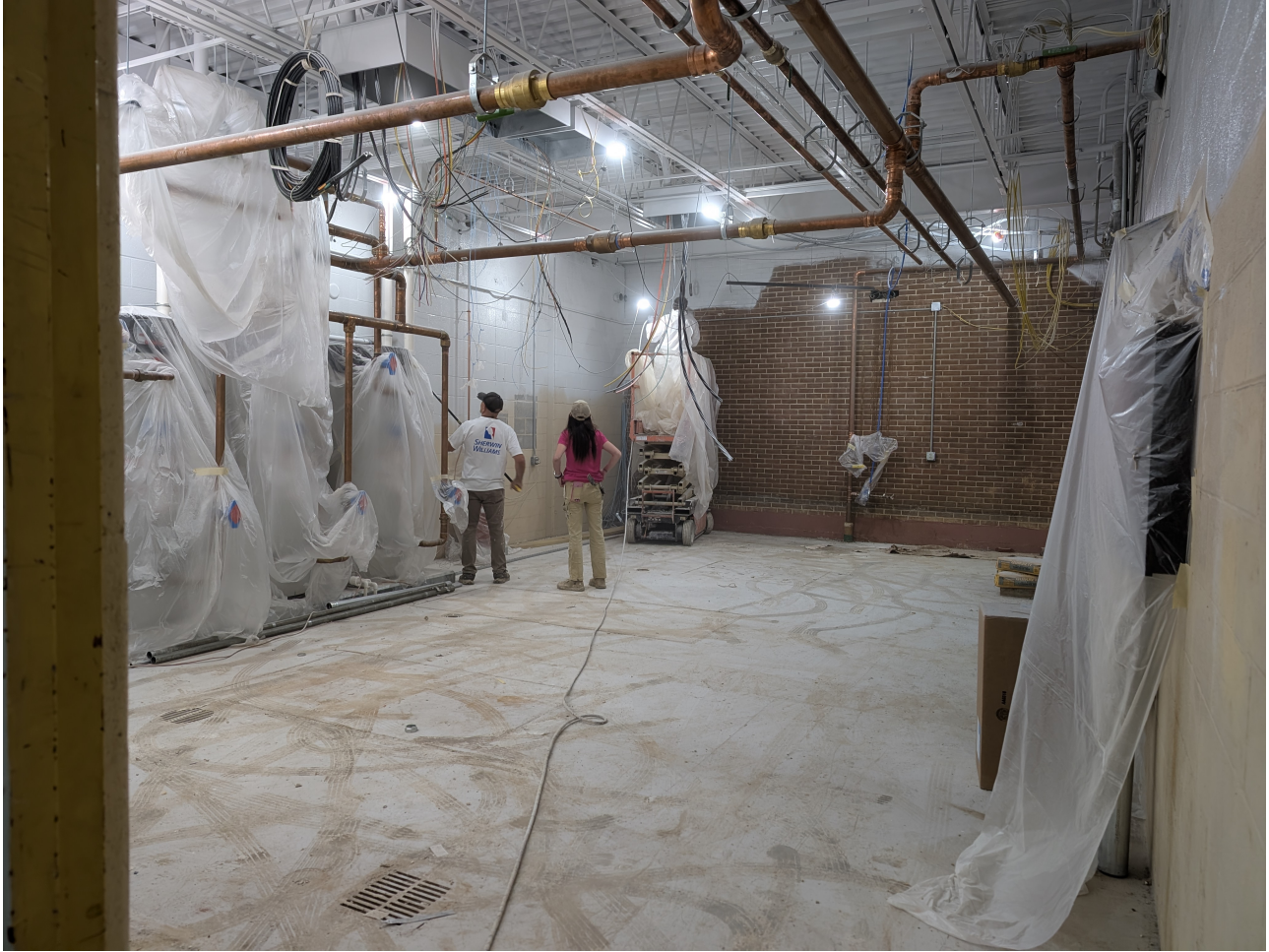
Painting of Interior Mechanical Room
