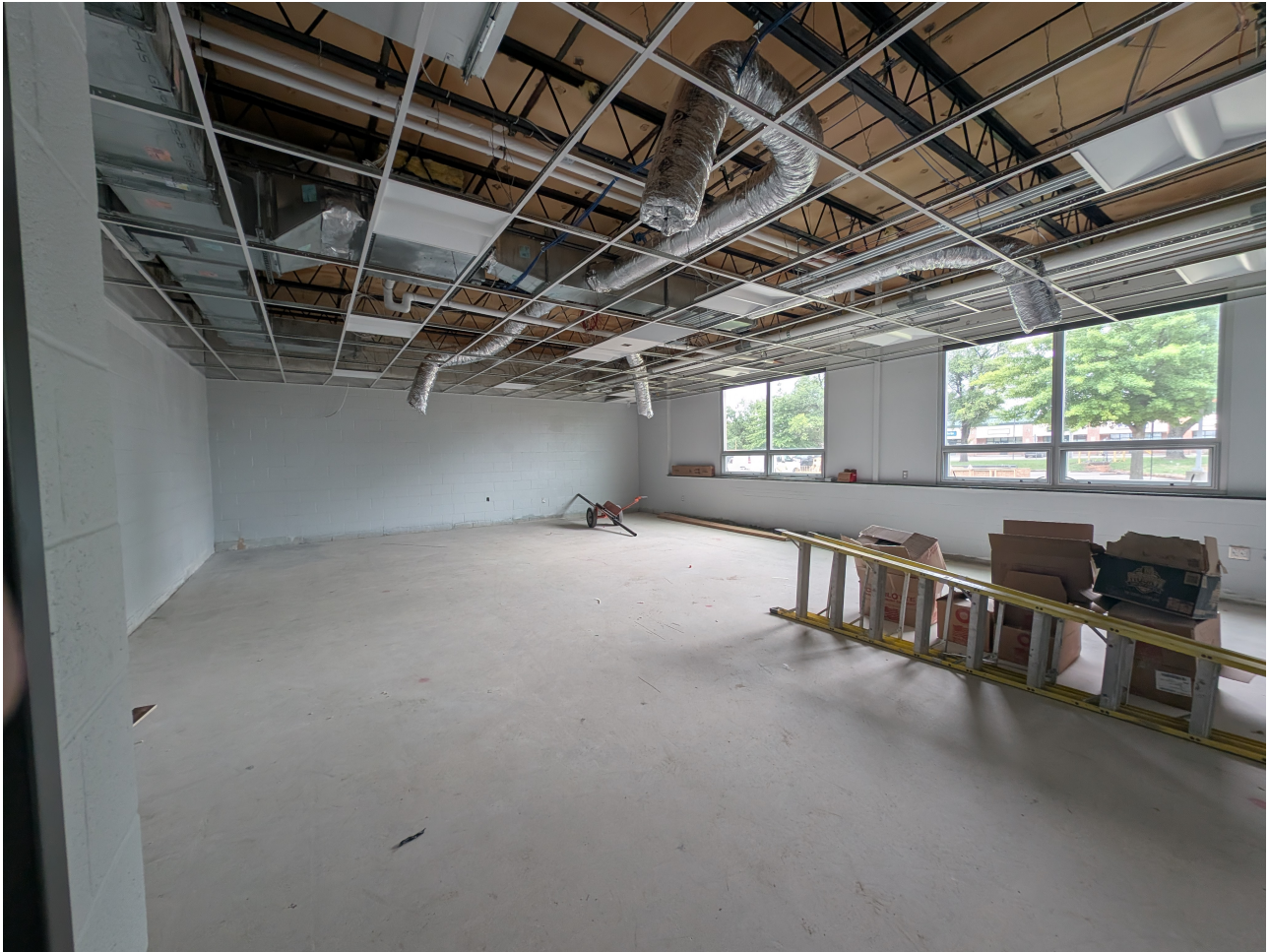
Classroom Progress in Classroom Wing 1 Area C
