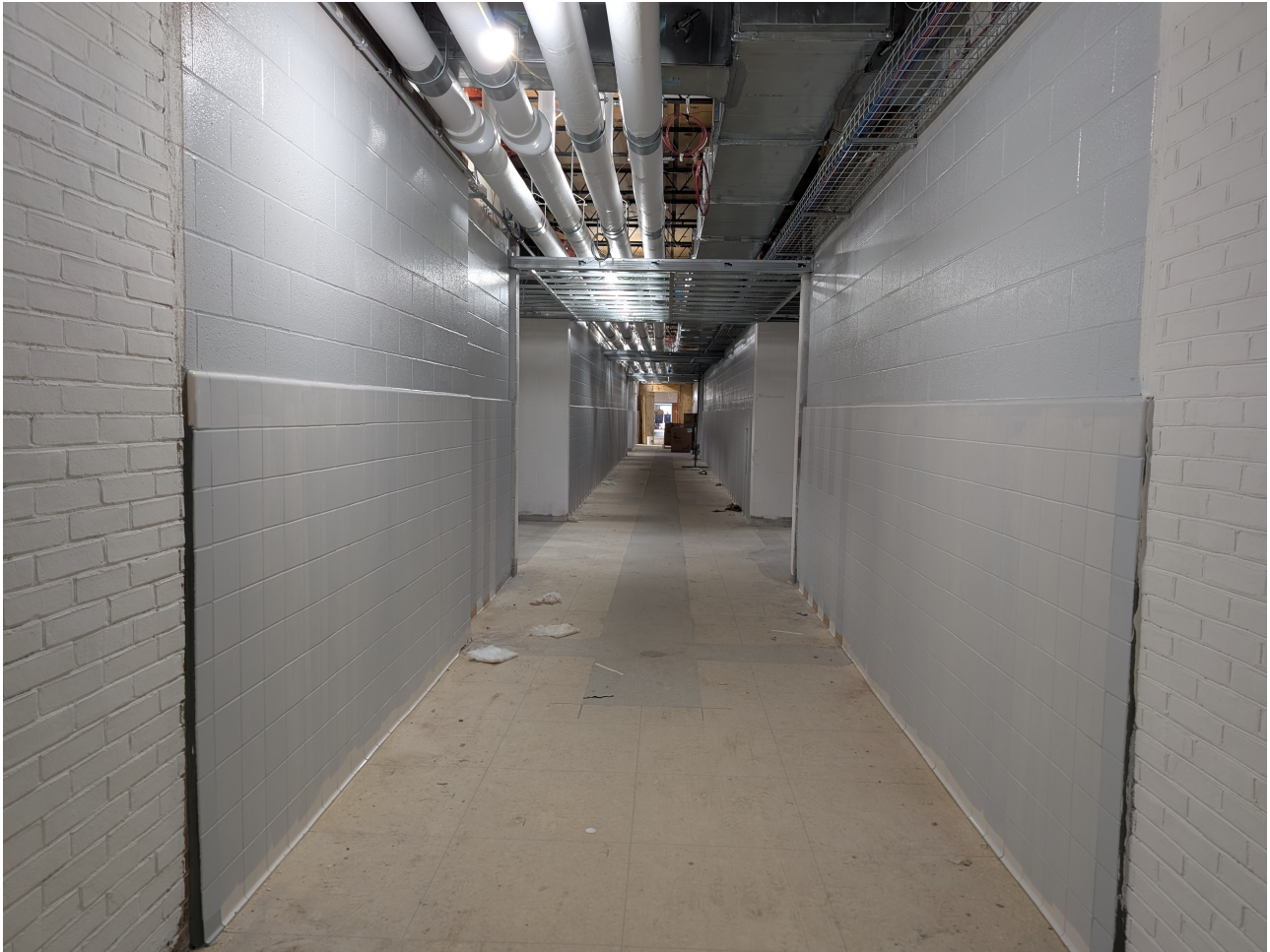
Classroom Wing 1 Area C Progress
