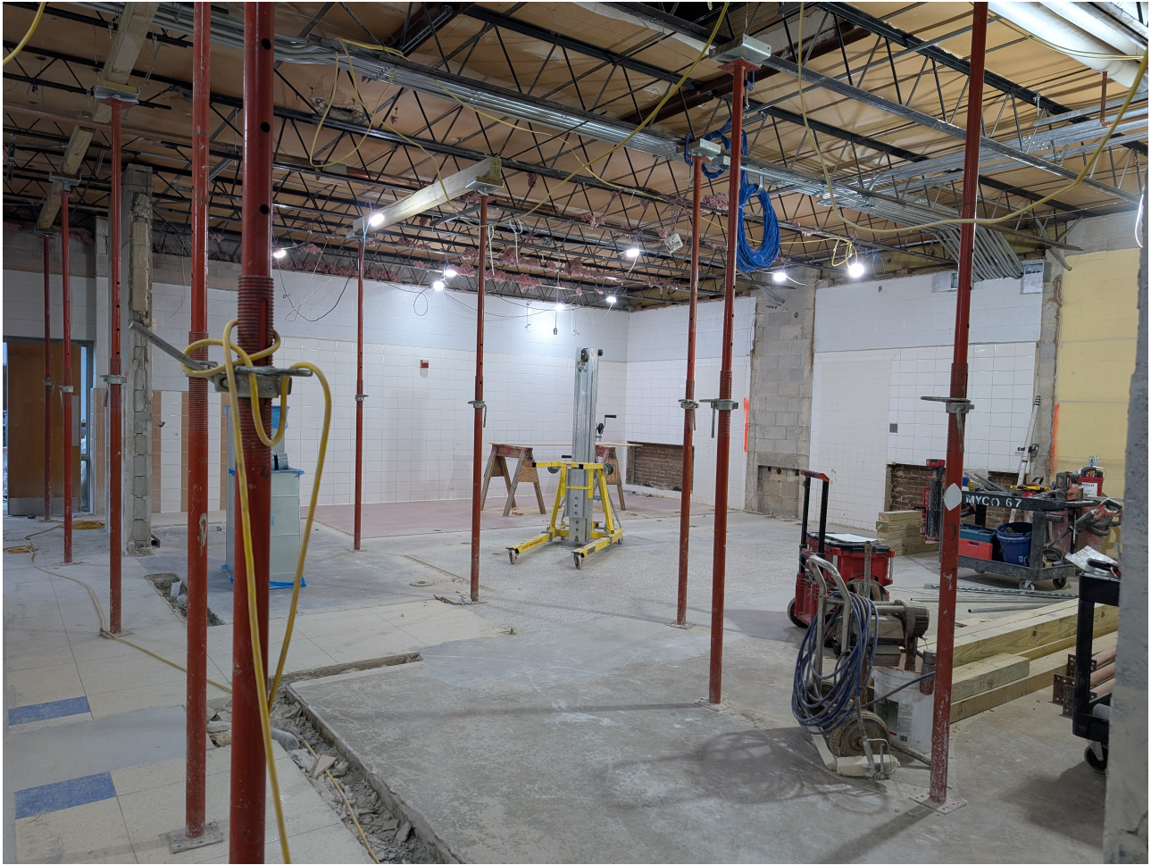
Gang Bathroom Demolition Progress Area C
