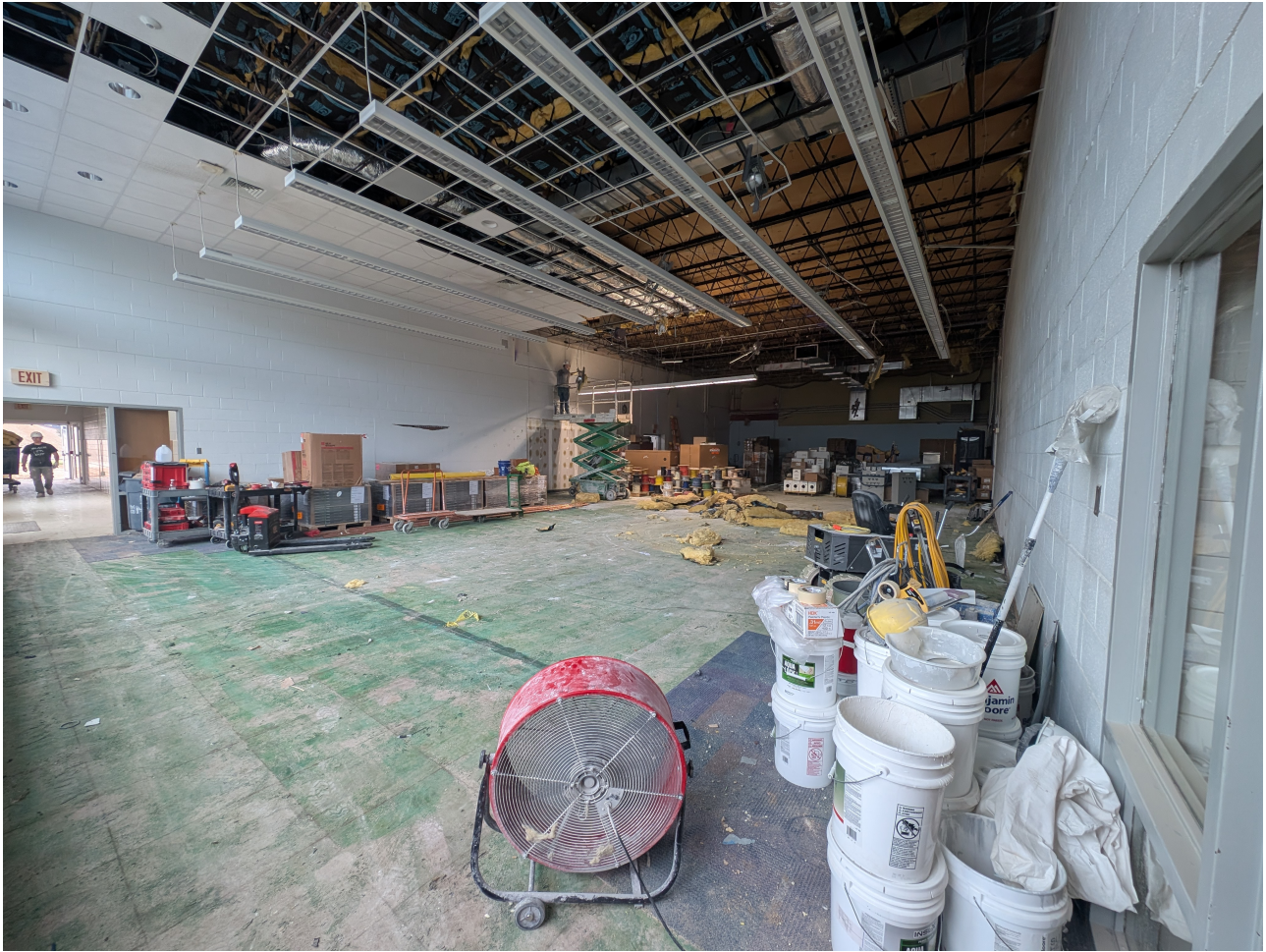
Library Demolition Progress
