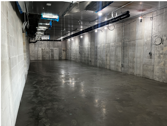
Concrete Poured – Area B1 Ground Level
