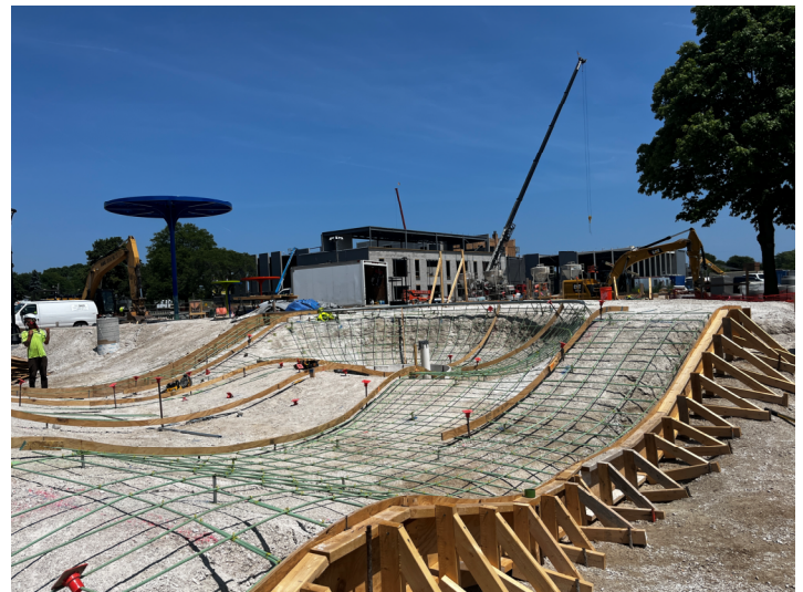
Installed Rebar – Pump Track – Site
