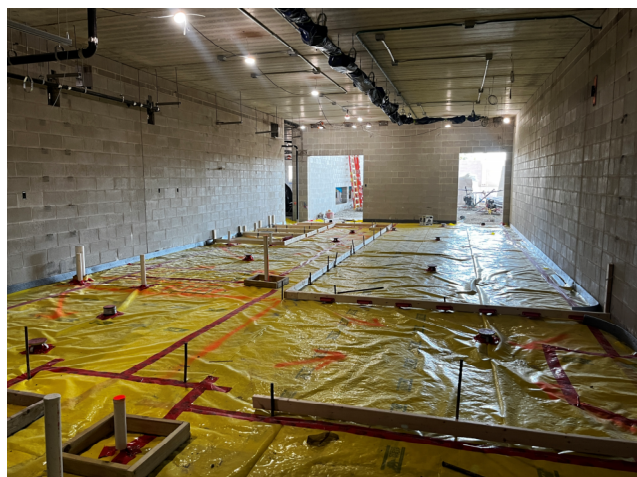
Room Prepped For Concrete Pour – Area B1 Ground Level
