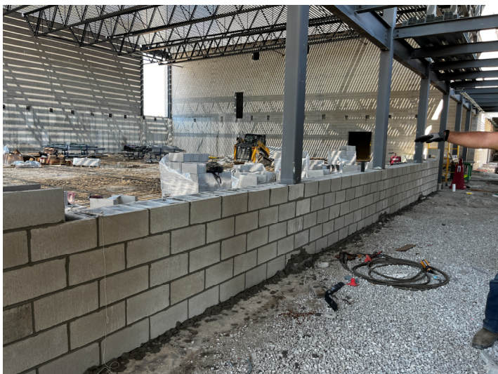
CMU Partition – Area C1 Ground Level Corridor
