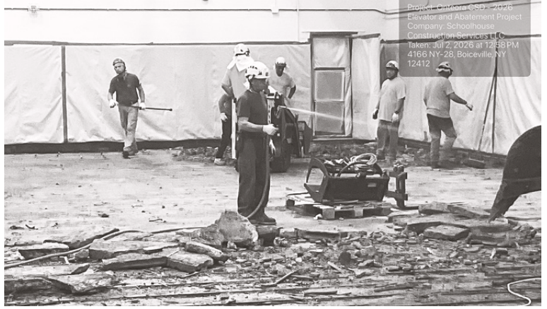
Our construction crew has been busy replacing the Middle School gymnasium floor. The work is anticipated to be completed and ready for students in October.
